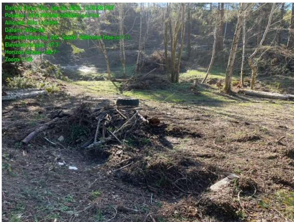
16. Cleared Vegetation at Willow Brook creek
