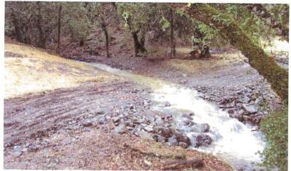
FIGURE 121E. Two weeks after this armored fill was constructed, a storm flow event occurred and the structure maintained its function and integrity. The road approaches had not yet been compacted or surfaced with road rock.
