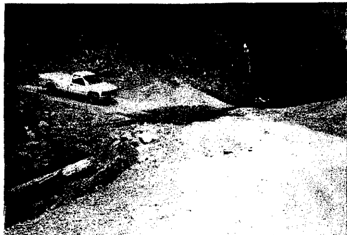
Figure 1. Wet ford on Class II perennial stream. Clean rock aggregate has been imported for the travelling surface and coarse rock armor protects the outer edge of the road bed. It is important that rock aggregate used in a ford be large enough to resist transport during winter flows. Fords should not be used if high winter flows would cut off access to inspect and maintain drainage structures further out the road. From Weaver and Hagans (1994).
