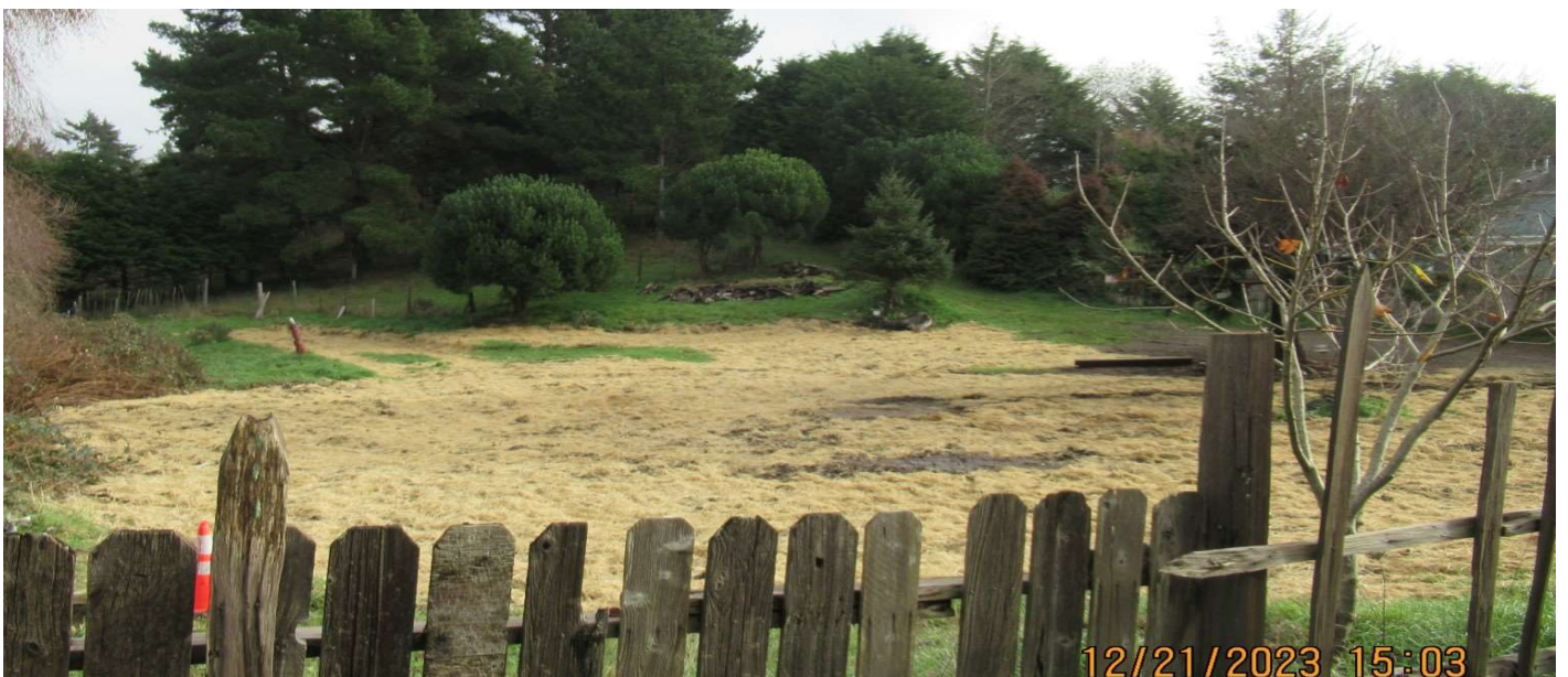
Weiler Road after abatement
