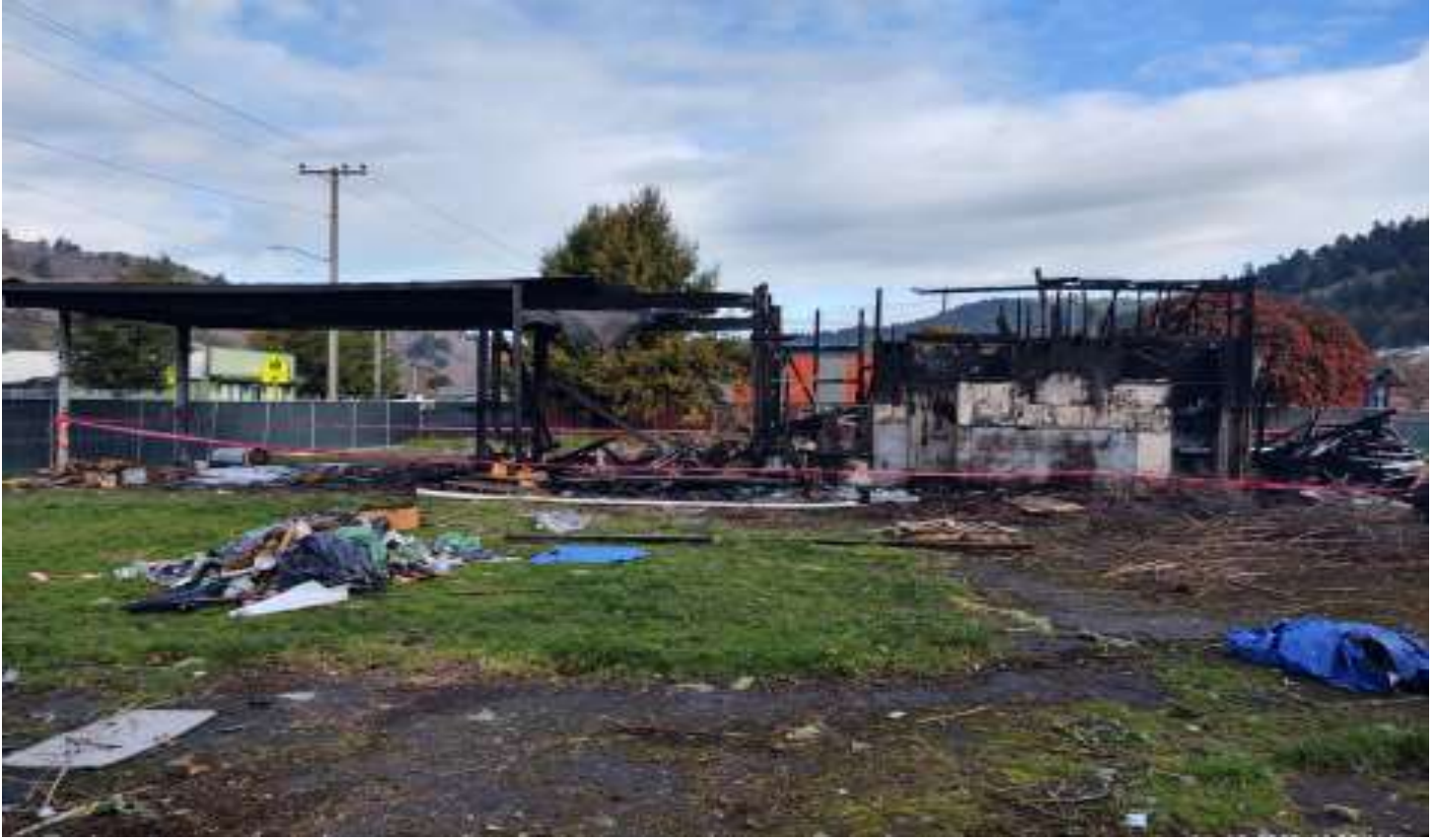
Gas station before abatement
