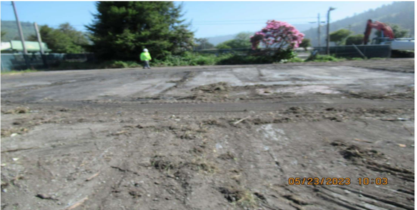
Gas station after abatement
