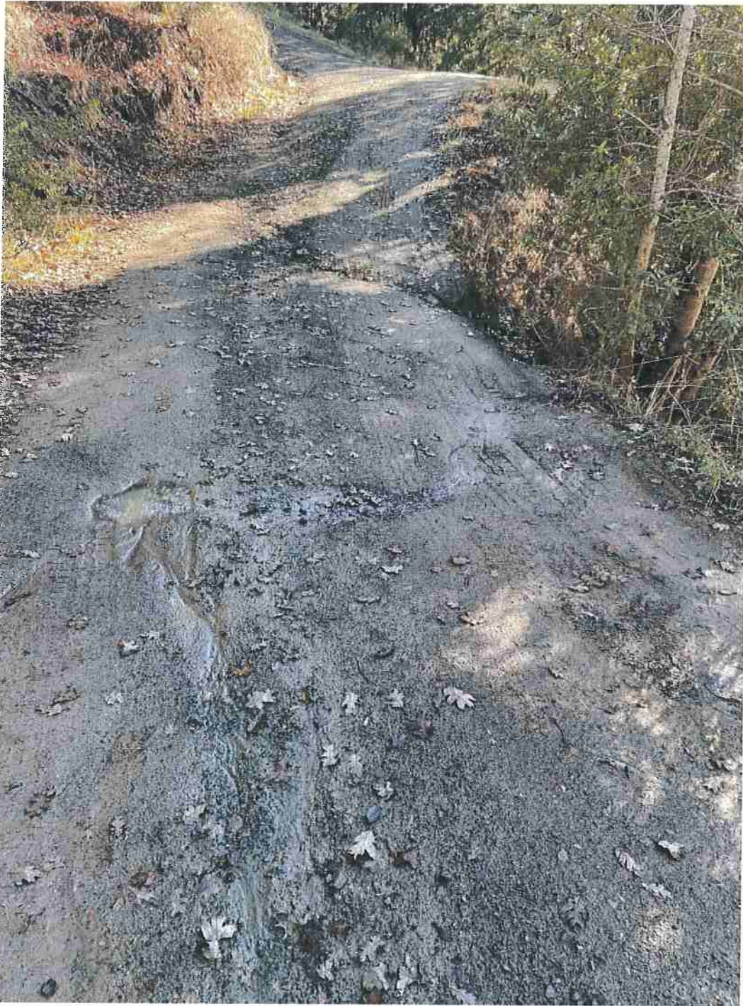
Photo 11. Watercourse crossing STX2.
