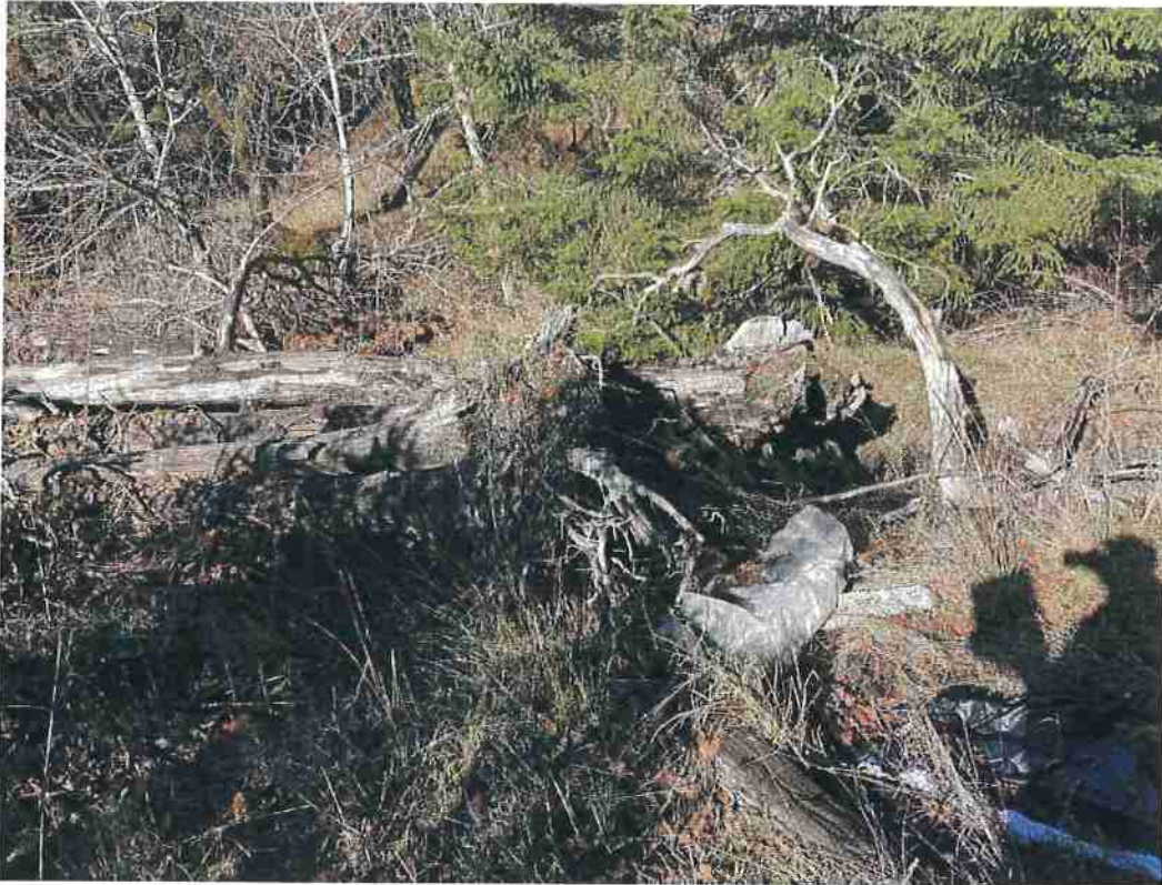
Photo 3. Conversion Site 2 – Hazard Reduction area along northern edge of Conversion Site.
