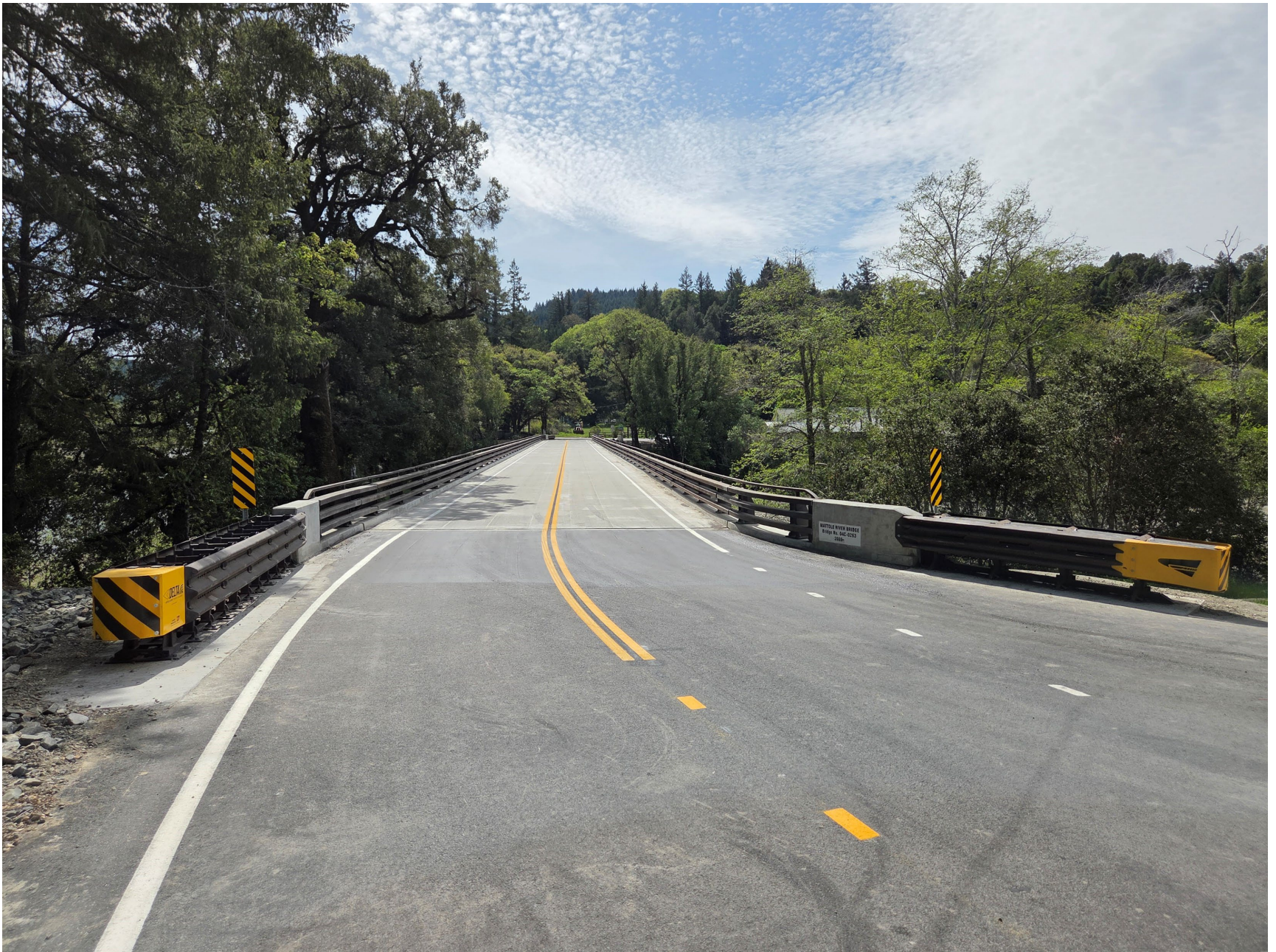
North side of the new bridge over the Mattole River at Honeydew (March 2026)
