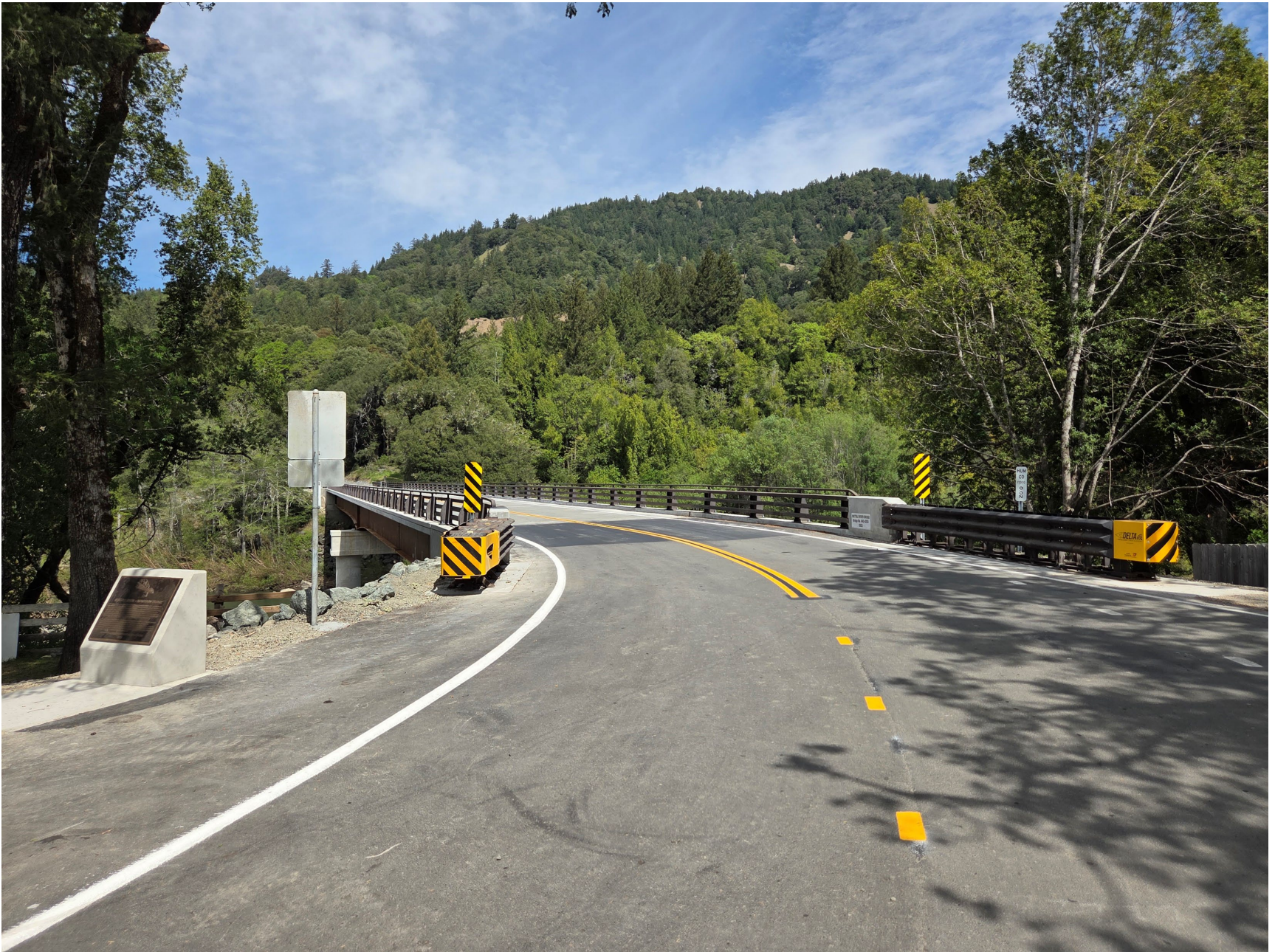
South side of the new bridge over the Mattole River at Honeydew (March 2026)
