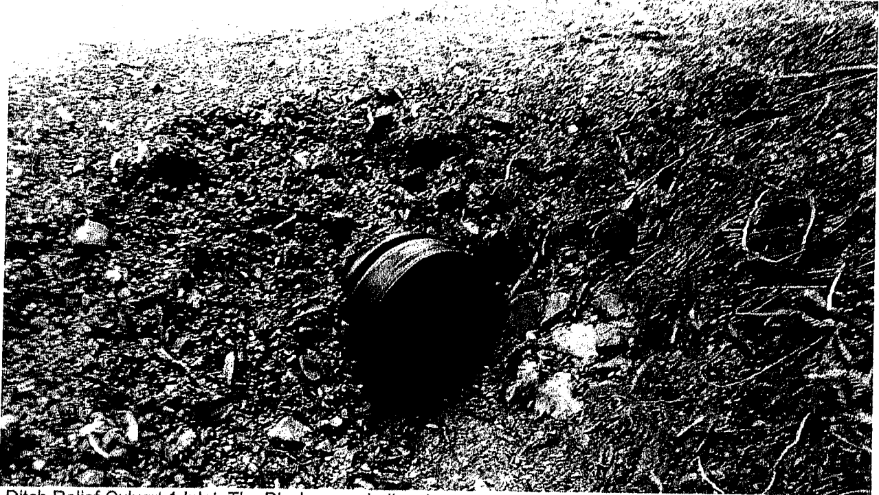
Ditch Relief Culvert 1 Inlet: The Discharger shall rock armor the inlet of this ditch relief culvert per attached specifications.
