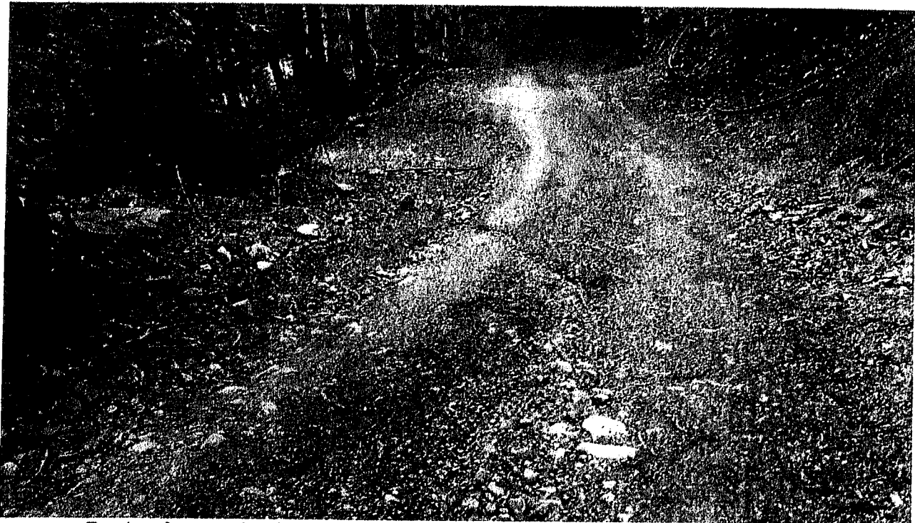
Road surface erosion that needs to be rocked between Road Point 4 and Road Point 6.
