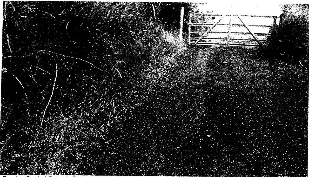
Erosion Control Point 2: Failed inside ditch draining onto the roads surface. The Discharger shall clear the inside ditch located along the left side of the photo and install a waterbar above the ditch that drains road surface flows into the inside ditch.
