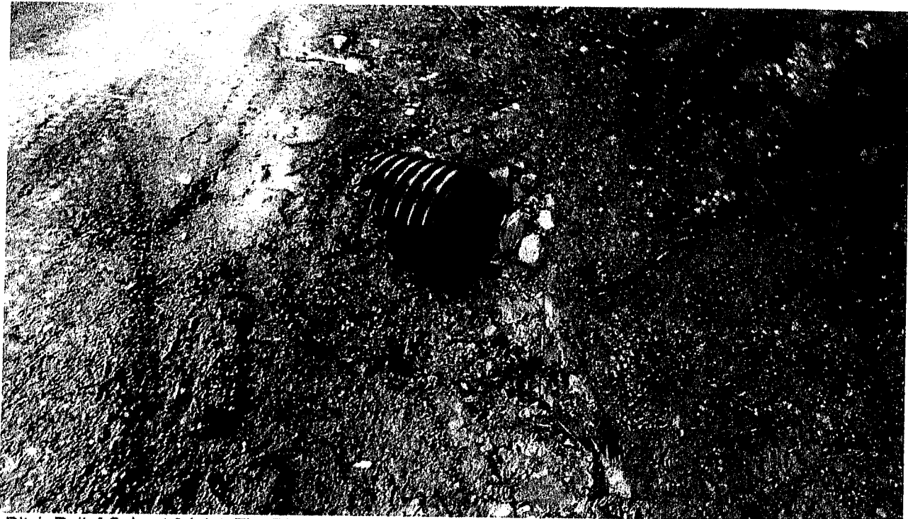
Ditch Relief Culvert 2 Inlet: The Discharger shall rock armor the inlet of this ditch relief culvert per attached specifications.
