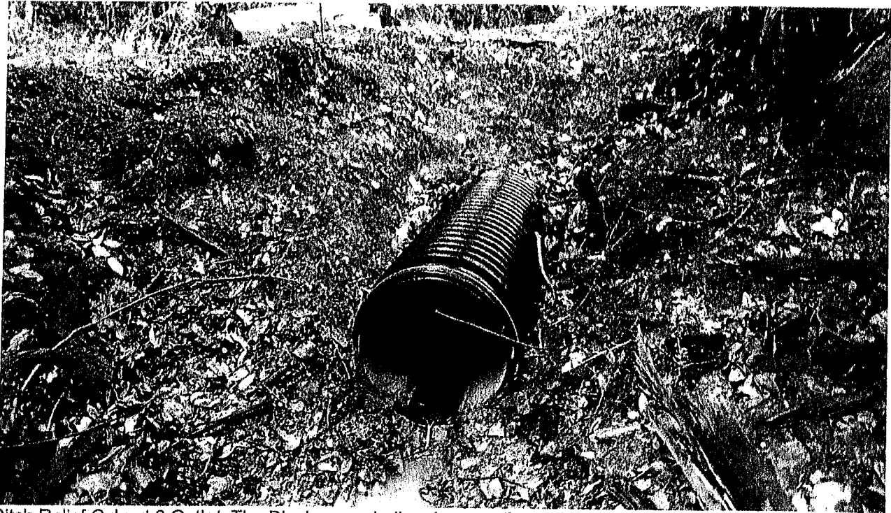
Ditch Relief Culvert 2 Outlet: The Discharger shall rock armor the outlet of this ditch relief culvert per attached specifications.
