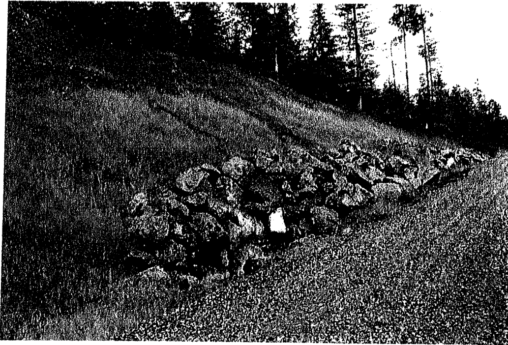
FIGURE 52. This wet and potentially unstable cut slope on a newly constructed road was stabilized using a buttress of large rock armor. To assure their effectiveness, rock buttresses and other retaining structures should be designed by a qualified engineer or engineering geologist.
