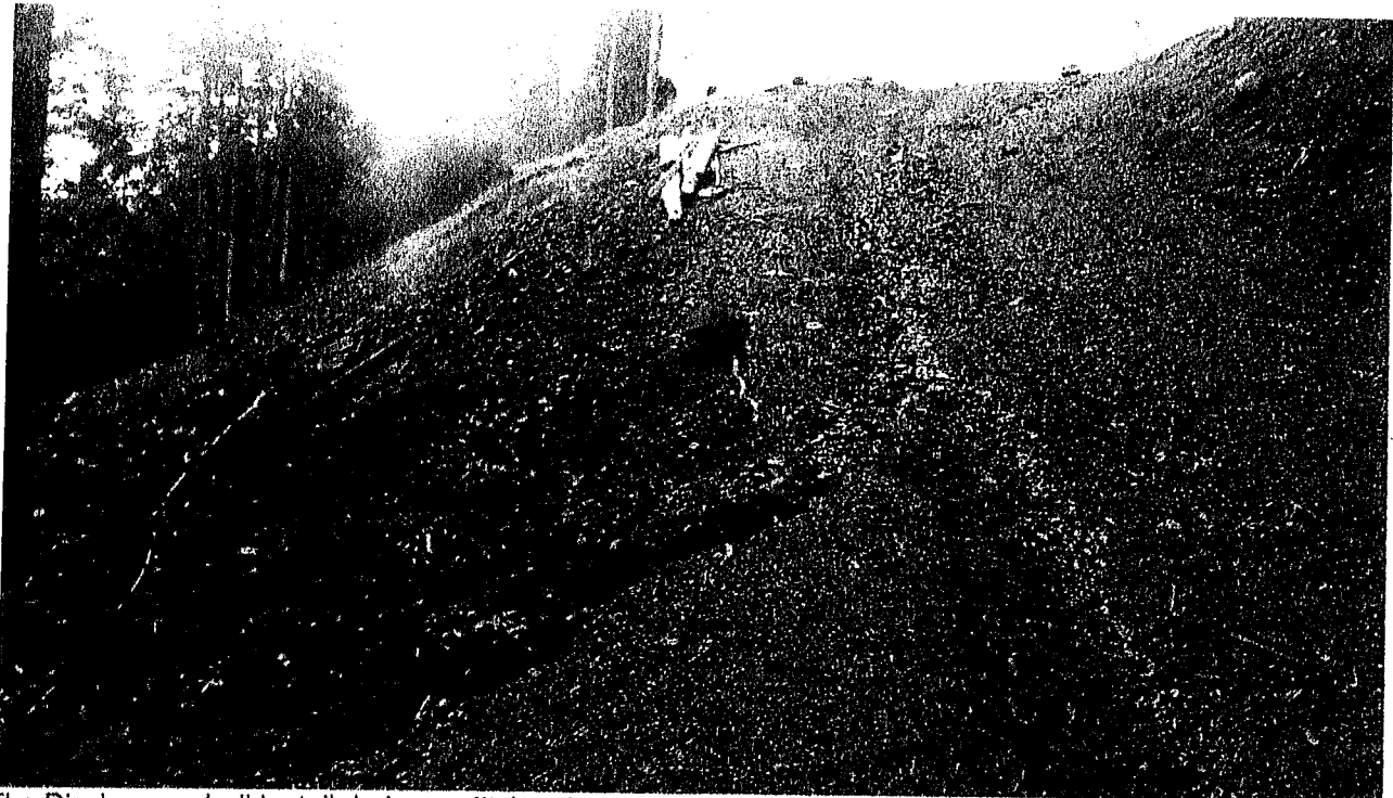
The Discharger shall install drainage ditches between the greenhouse above in the photo and direct the flows of the drainage ditches to the back of the greenhouses so that they no longer drain onto the road as shown in the photo above. This segment of road, between Road Point 4 and Road Point 6 shall be rocked.
