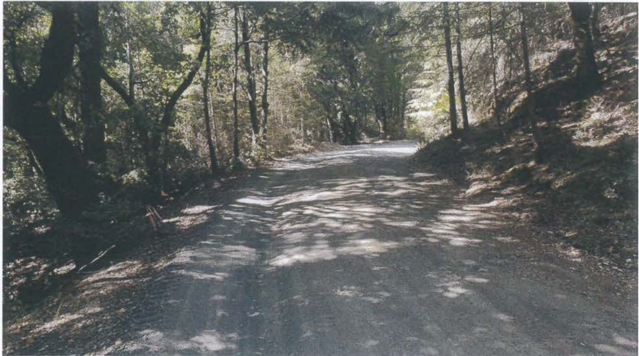
Site 25 looking up grade towards Site 24.
