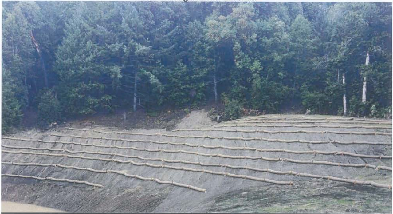
Jute netting & Straw-wattles
