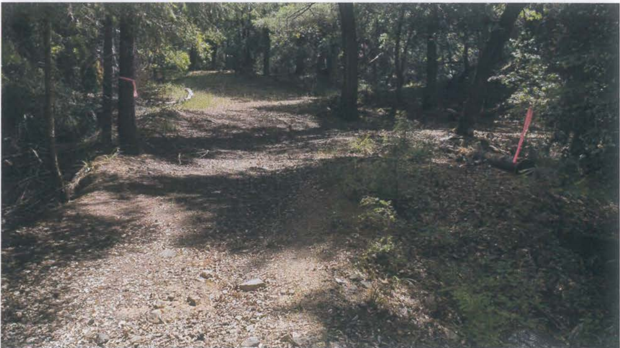
Site 19. Approximate location of watercourse re-alignment. A waterbar (Site 18) will be installed further up grade from the re-aligned watercourse.
