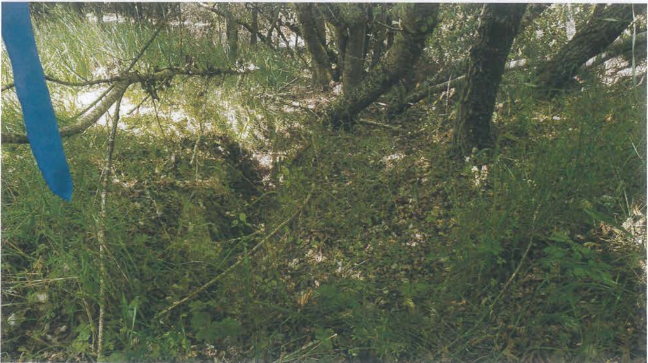
Site 35. Looking at the down channel and where the culvert outlet will approximately be located.
