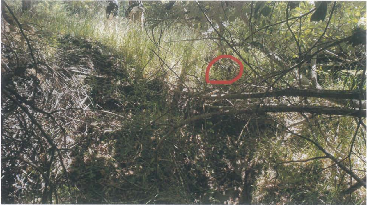
Site 35. Looking at the outlet(circled). The culvert upgrade will re-align the watercourse to its original channel, which will require the outlet to be placed in the lower left of the photo.
