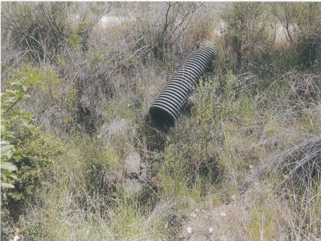
Site 11. Looking at the outlet of the culvert.
