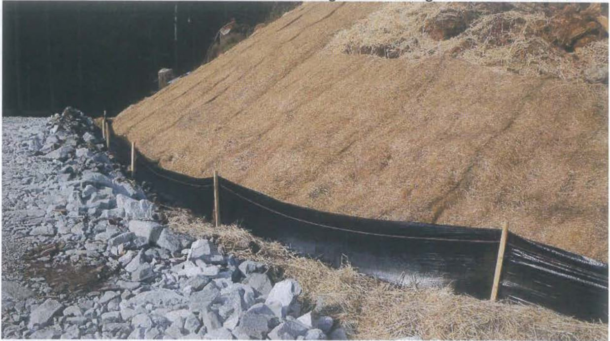
Erosion Control Matting & Silt Fencing
