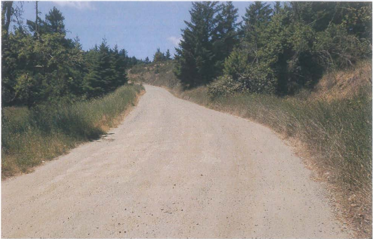
Looking up grade from Site 12 towards Site 11.
