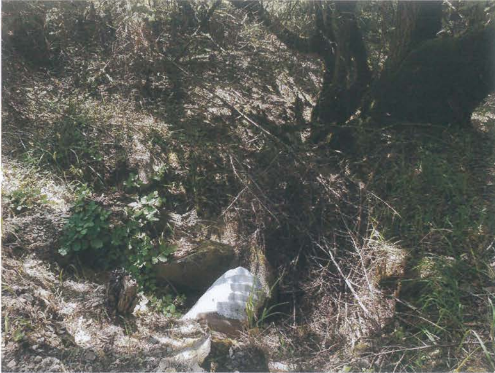
Site 05. Looking down-channel from the outlet.
