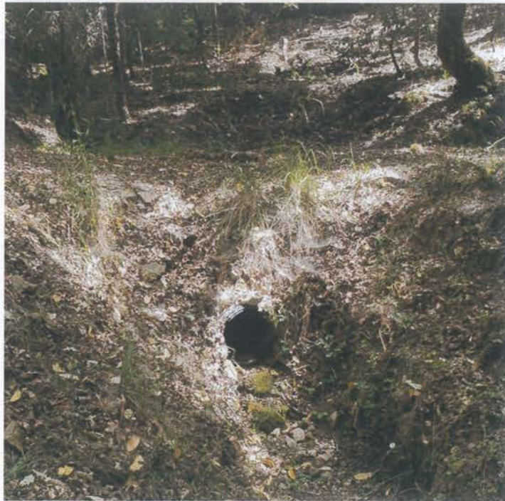
Outlet of the watercourse crossing at Site 17
