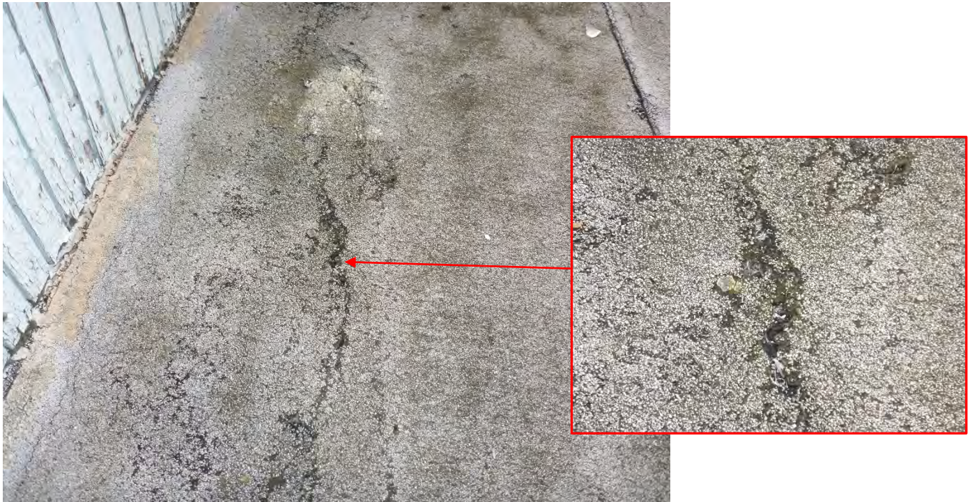
Photo #18: Roof has open voids and gaps. Holes in roof.
