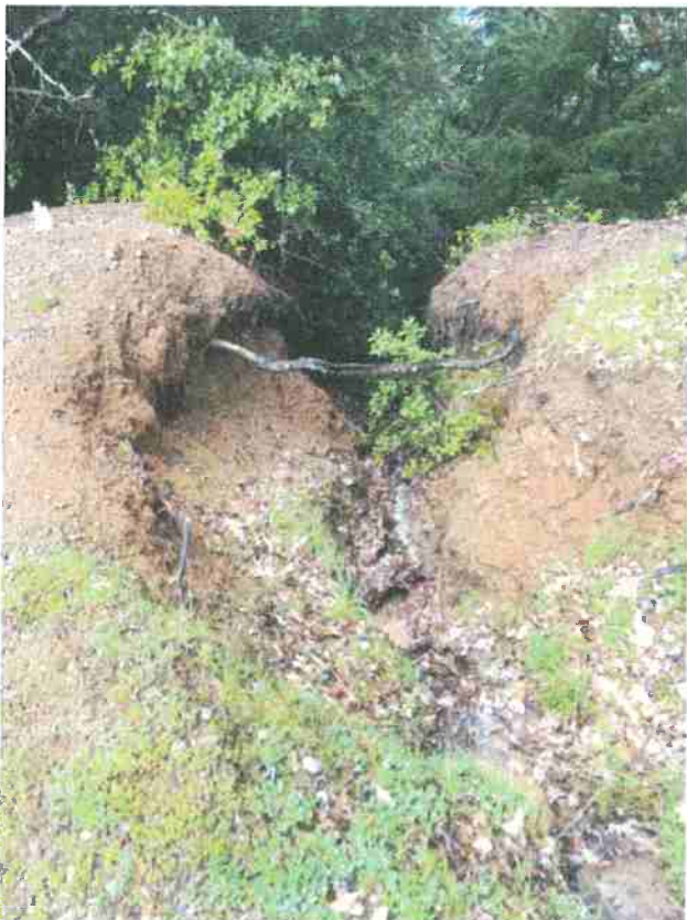
Unprotected discharge point.
