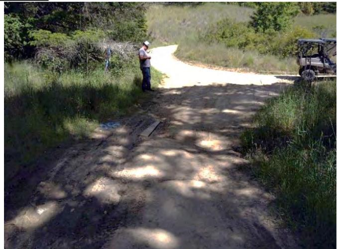
87. Inside ditch drains 200 feet of inboard ditch across a road intersection and into a class III watercourse adjacent to point 86. Direct the inside ditch into the inlet side of 86. The inside ditch shall then be lined for 200' up to road point 88. Line ditch with 2" to 4" sharp angular rock (15 yards). **223-074-004**
