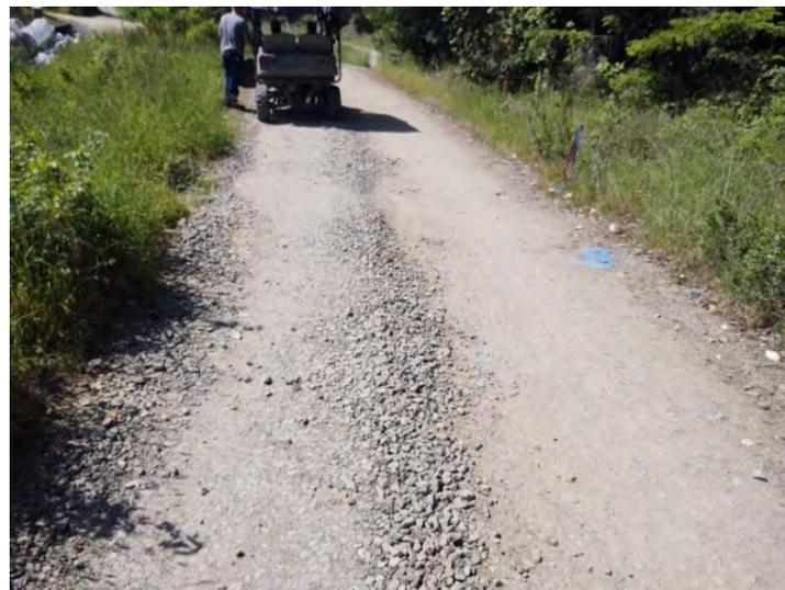
99.5 Install rocked rolling dip across entire width of road. Catch inside ditch. Line dip with 1-2 yards of 2" to 4" sharp angular rock. **223-074-006**
