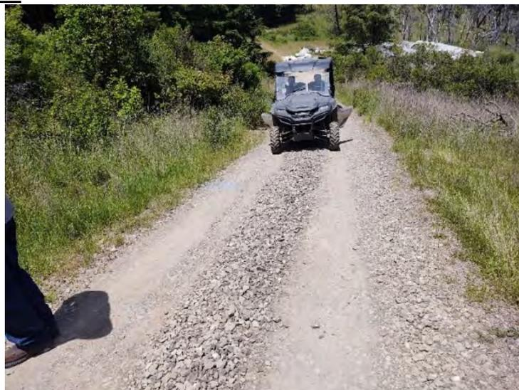
93. Install rocked rolling dip across entire width of road. Line dip with 1-2 yards of 2" to 4" sharp angular rock.
