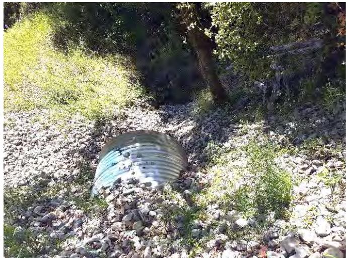
57. Surface drainage present. Maintain inside ditch around the turn and drain at the existing location. Line the nick point at the outlet of the inside ditch with 3 yards of 2" - 4" diameter rock. **223-074-009**
