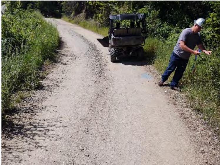
90. Install a 24" diameter cross drain. Rock nick point at outlet with 1-2 yards, 2"-4" rock to prevent erosion. Clean inside ditch back to the intersection. **223-074-004**
