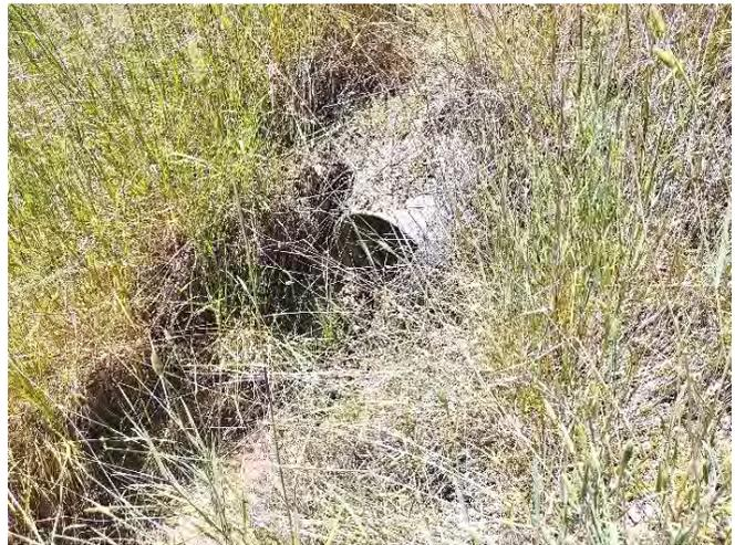
48. Surface drainage present. Install rocked rolling dip across entire width of road. Line dip with 1-2 yards of 2" to 4" sharp angular rock. Dip can drain left or right. Excessive cannabis debris and soil present adjacent to the landing. Remove debris and soil by hand. **223-074-009**
