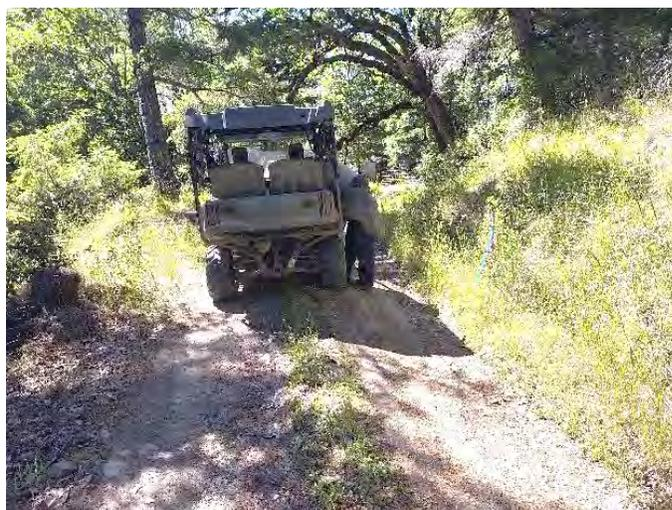
37. Surface drainage present. Install rocked rolling dip across entire width of road. Line dip with 1-2 yards of 2" to 4" sharp angular rock. Dip can drain left or right prior to the gate entrance. **223-074-006**
