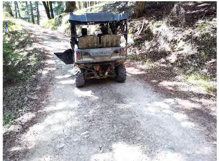
6. Surface drainage present. Install rocked rolling dip across entire width of road. Line dip with 1-2 yards of 2" to 4" sharp angular rock. **223-074-009**
