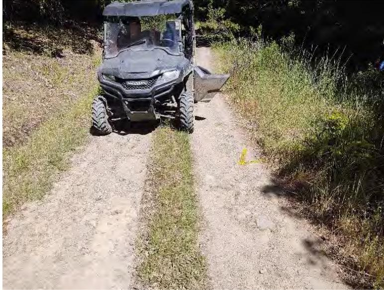
8. Existing 18" cross drain. Clean and maintain. Inslope road towards inlet of cross drain. Place ½ yard of 2"-4" of rock at the outlet to slow overland flow. **223-074-009**
