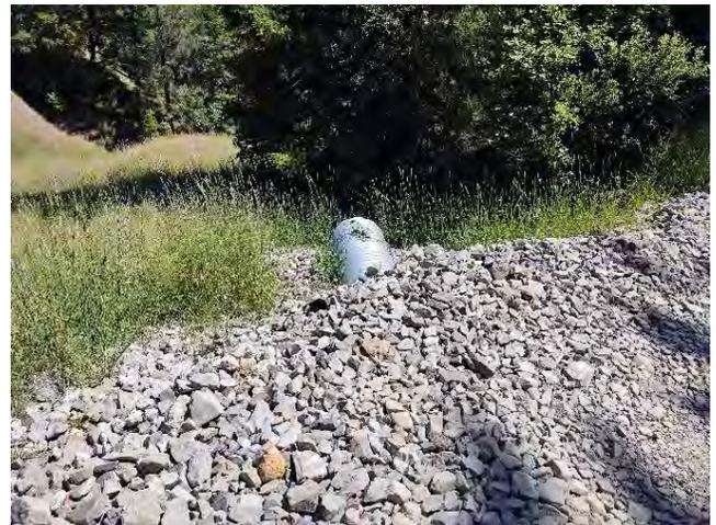
60. Surface drainage present. Install rocked rolling dip across entire width of road. Line dip with 1-2 yards of 2" to 4" sharp angular rock. **223-074-004**
