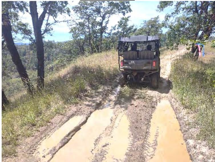
96.5 Install rocked rolling dip across entire width of road. Catch inside ditch. Line dip with 1-2 yards of 2" to 4" sharp angular rock. **223-074-004**
