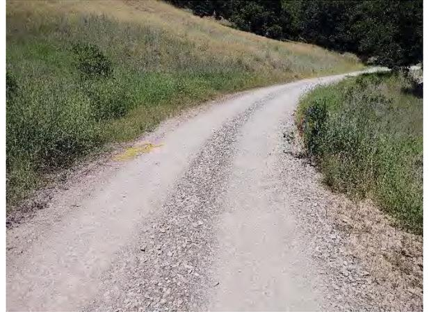
53. Surface drainage present. Install rocked rolling dip across entire width of road. Line dip with 1-2 yards of 2" to 4" sharp angular rock. Add rock down the outboard edge of the road for 3' to protect the nick point erosion. **223-074-009**
