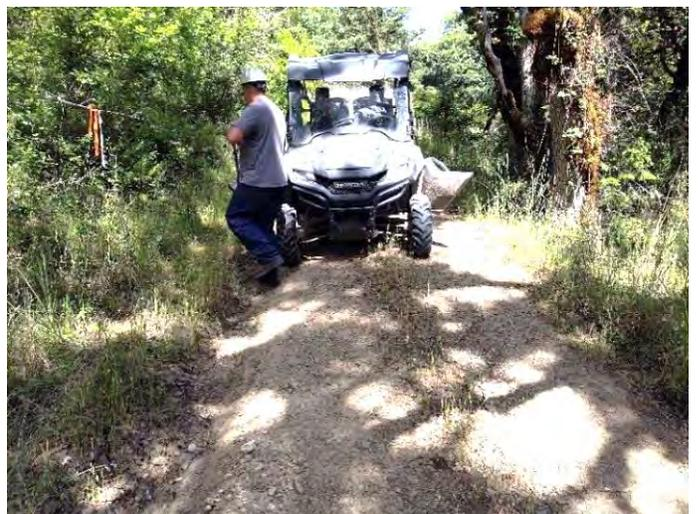
76. Surface drainage present. Install rocked rolling dip across entire width of road. Line dip with 1-2 yards of 2" to 4" sharp angular rock. **223-074-004**
