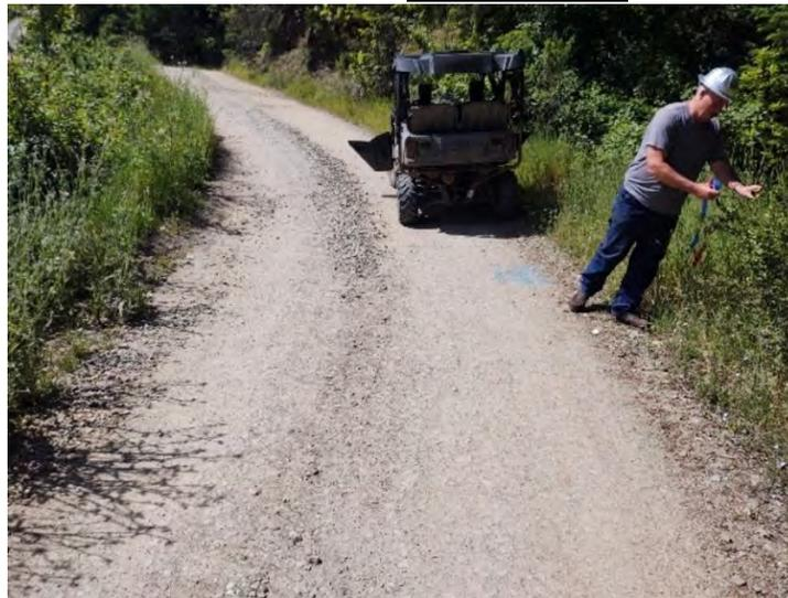
99. Install rocked rolling dip across entire width of road. Line dip with 1-2 yards of 2" to 4" sharp angular rock. **223-074-006**
