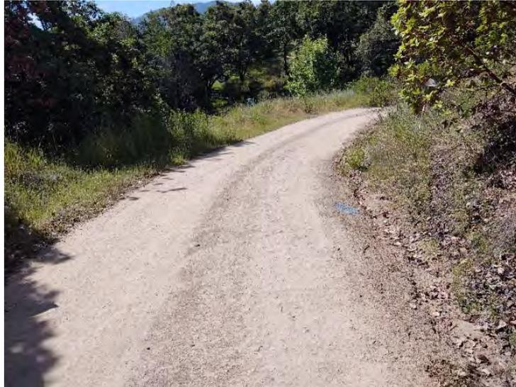
89. Install rocked rolling dip across entire width of road. Catch inside ditch. Line dip with 1-2 yards of 2" to 4" sharp angular rock. Clean the inside ditch back up the road for 50'. **223-074-004**
