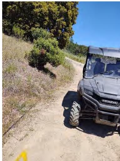
58. Surface drainage present. Install rocked rolling dip across entire width of road. Line dip with 1-2 yards of 2" to 4" sharp angular rock. **223-074-009**
