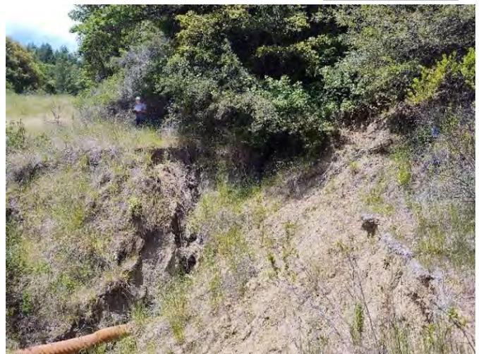
71. Over hanging fill present for 40'. Crossing is beyond crossing 70 and shall not be repaired. Excavation of site would increase soil erosion by 2 x the amount present. Site shall naturally meter spoils to watercourse. No operations are recommended. 50 cu yard potential sediment. ECP **223-074-006**
