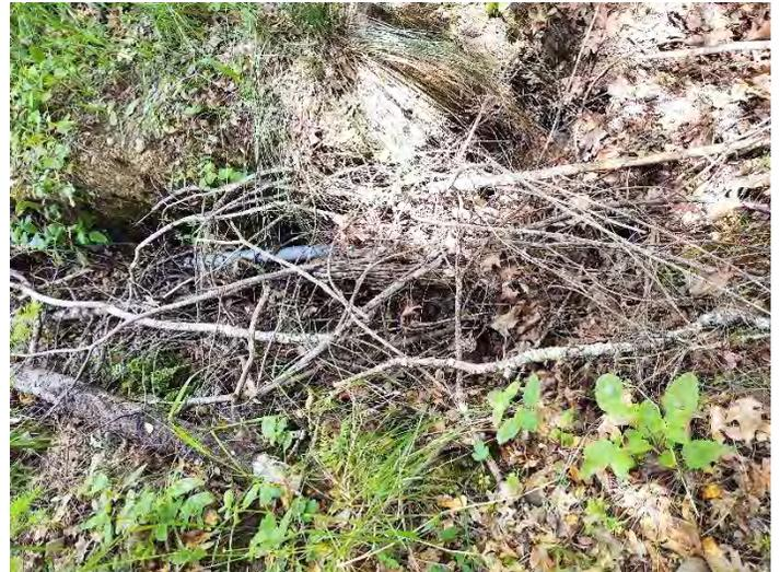
74. Surface drainage present. Install rocked rolling dip across entire width of road. Line dip with 1-2 yards of 2" to 4" sharp angular rock. **223-074-004**
