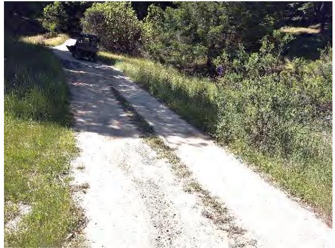
5. Surface drainage present. Install rocked rolling dip across entire width of road. Line dip with 1-2 yards of 2" to 4" sharp angular rock. **223-074-009**
