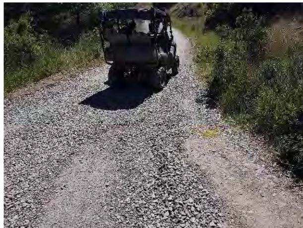
54.5. Surface drainage present. Install rocked rolling dip across entire width of road. Line dip with 1-2 yards of 2" to 4" sharp angular rock. **223-074-009**
