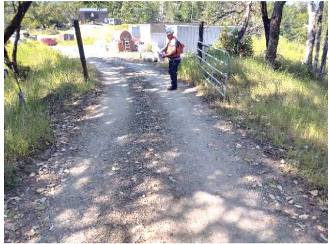
38. Surface drainage present. Install rocked rolling dip across entire width of road. Line dip with 1-2 yards of 2" to 4" sharp angular rock. Drain right. **223-074-006**
