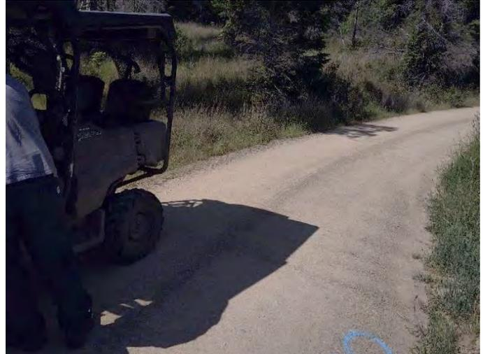
91. Storm flow crosses at the base of road intersection. Install 24" diameter culvert at the corner and direct it across the mainline road and into the vegetation. **223-074-004**
