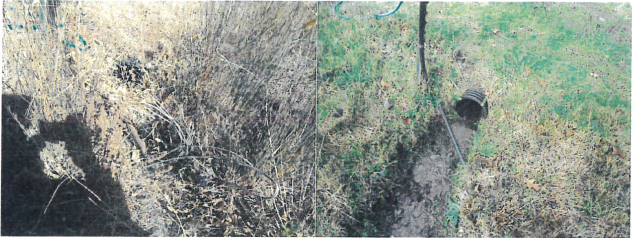
Ditch relief culverts during September site visit, then during monitoring October 18, 2016
