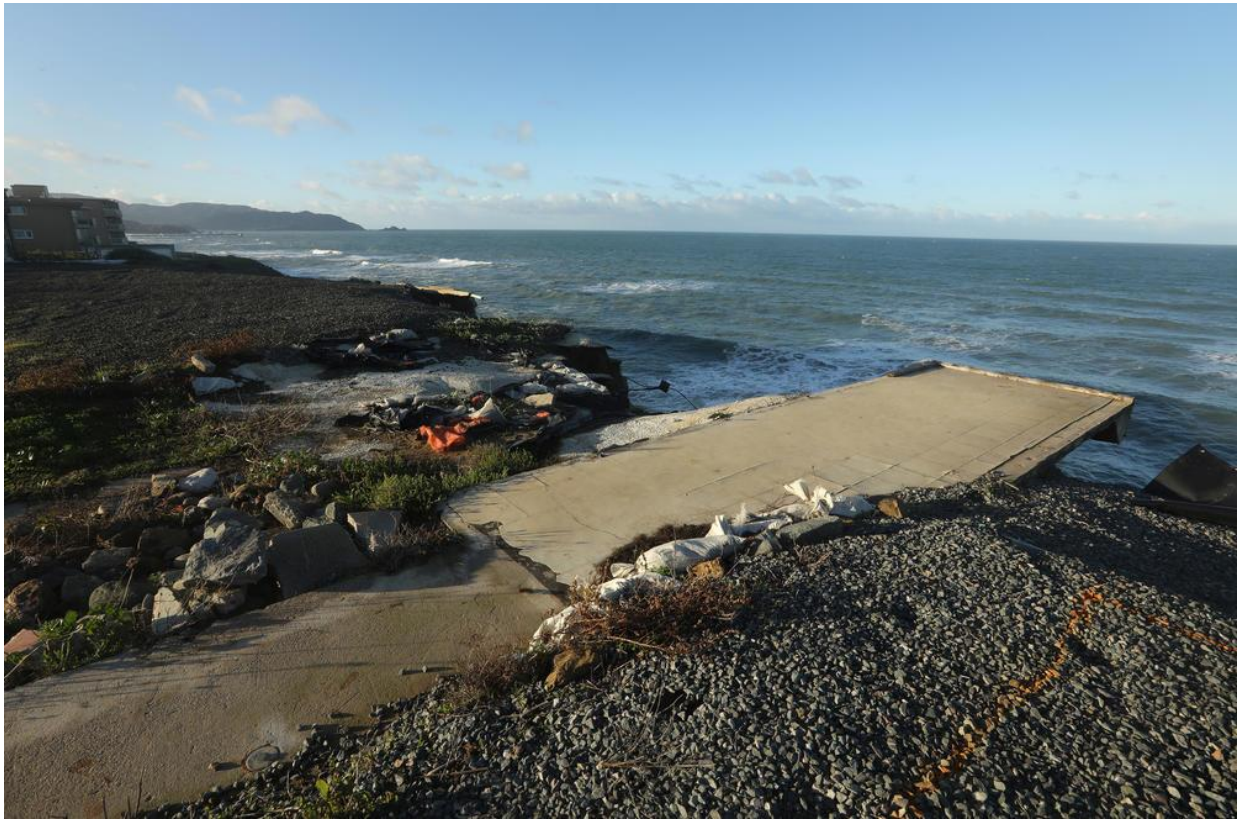
Along Esplanade Avenue in Pacifica, a walkway is all that's left of an apartment building. (Carolyn Cole / Los Angeles Times)
