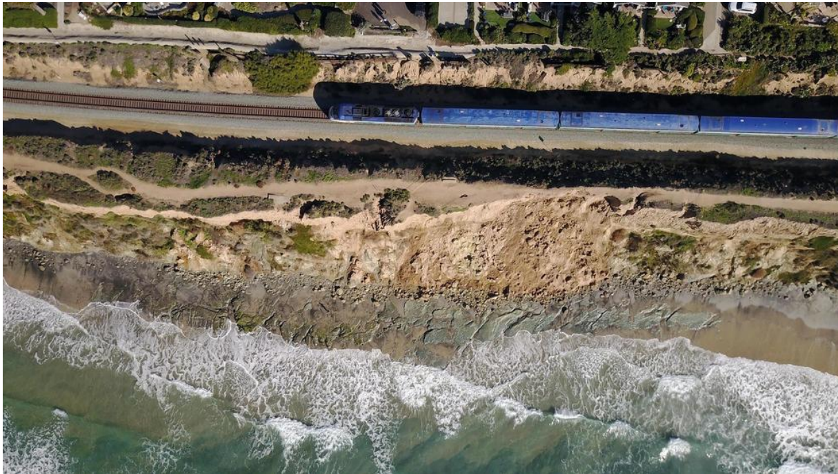
On the southern end of Del Mar, train tracks run precariously close to the edge of rapidly crumbling cliffs. (John Gibbins / San Diego Union-Tribune)
