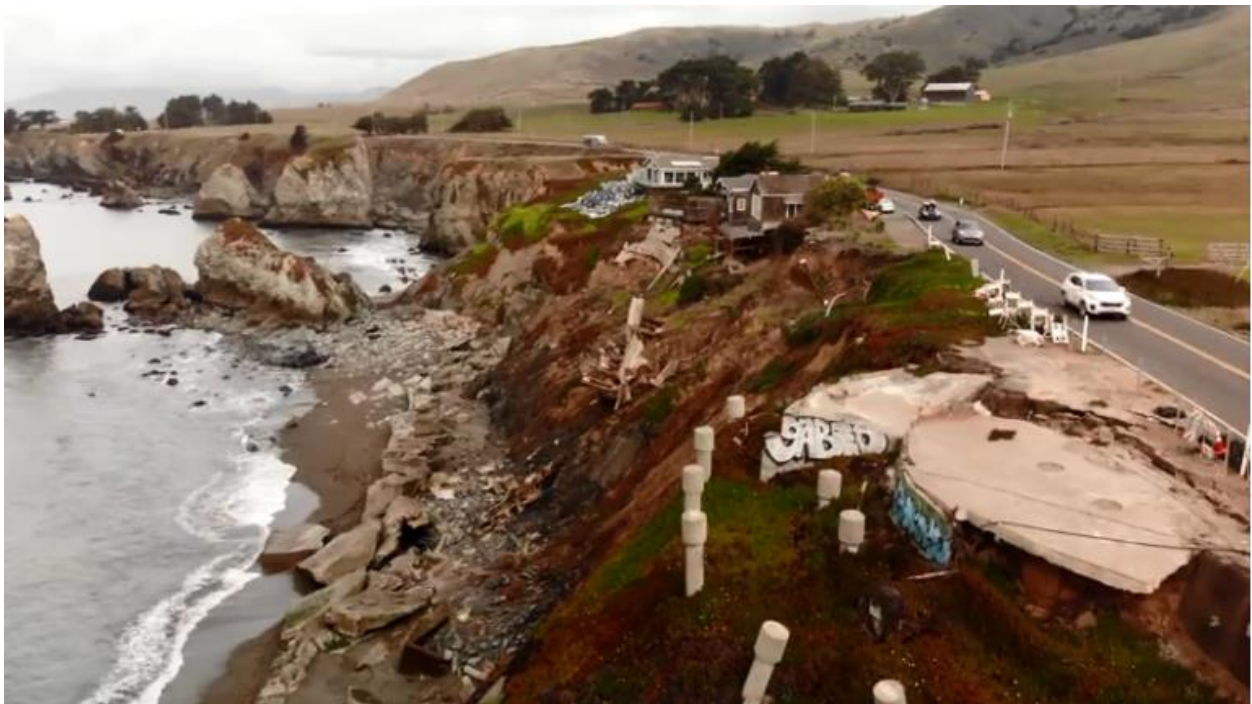
At Gleason Beach, remnants of homes and piles of seawalls, smashed into pieces, clutter the coastline. (Carolyn Cole / Los Angeles Times)
