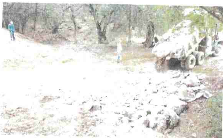
FIGURE 121D Well graded rock armor is then backfilled into the structure and spread across the breadth of the U-shaped stream crossing, and about one-third the way up the roadbed, so that streamflow will only flow over or come in contact with resistant armor material. The armor must be spread and compacted across the design width of the expected flood flow channel width so peak flows will not flank the armored structure.
