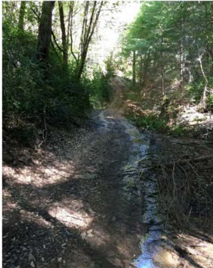
Figure 2. Steep road segment and intermittent watercourse diversion immediately adjacent to a perennial Class II stream.
