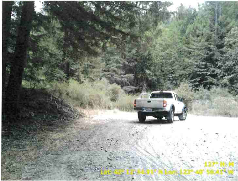
Figure 5.. Photograph showing Road Point 24 which is a pullout that shall be maintained as a pullout.
