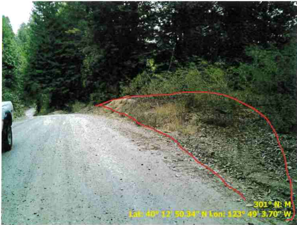
Figure 8. Photograph showing Road Point 16 which is a pullout that need to be regraded.
