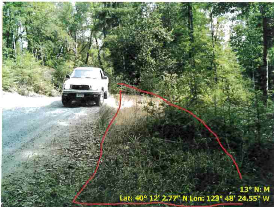
Figure 22. Photo of Road Point 84 showing a pullout that needs to be regraded and vegetation cleared.
