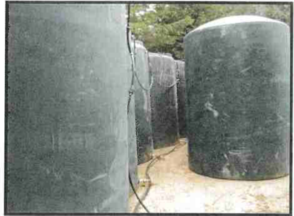
Eight (8) 5000 gallon storage tanks= 40,000 gallon storage
