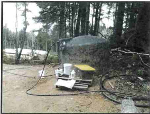
1500 gallon mixing tank
