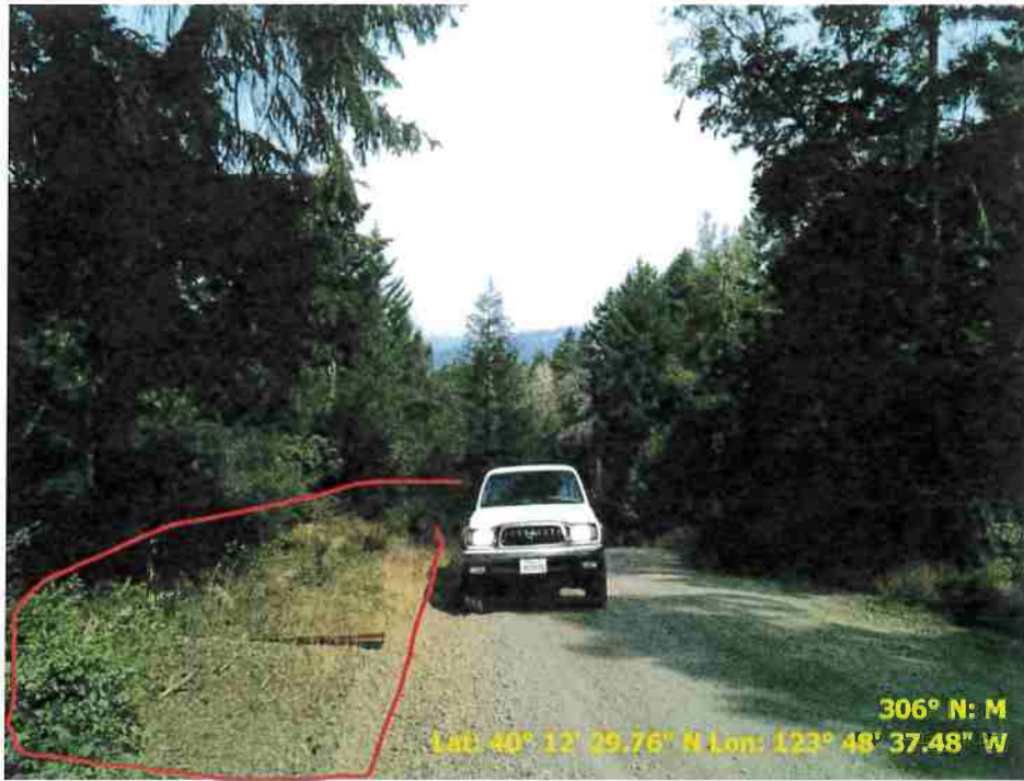
Figure 15. Photo of Road Point 71 showing a pullout that needs to be regraded.
