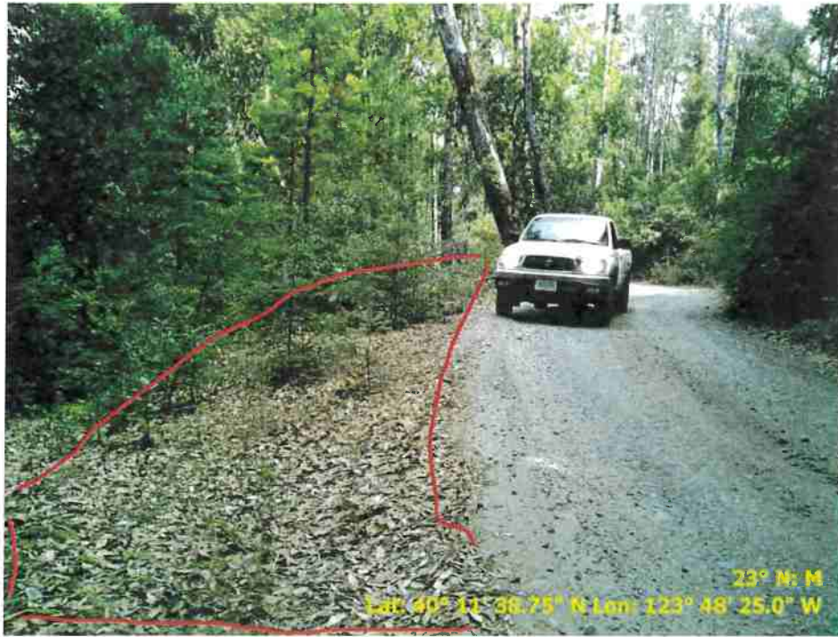
Figure 31. Photo of Road Point 104 showing a pullout that needs to be cleared of vegetation and regrading.
