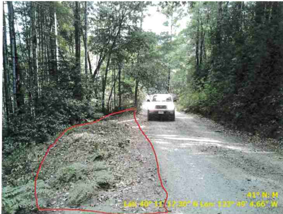
Figure 39. Photo of Road Point 127 showing a pullout that needs to be cleared of vegetation and regrading.
