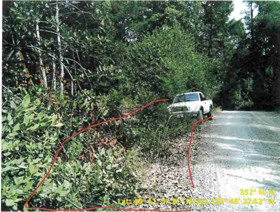
Figure 27. Photo of Road Point 91 showing a pullout that needs vegetation cleared and to be regraded.
