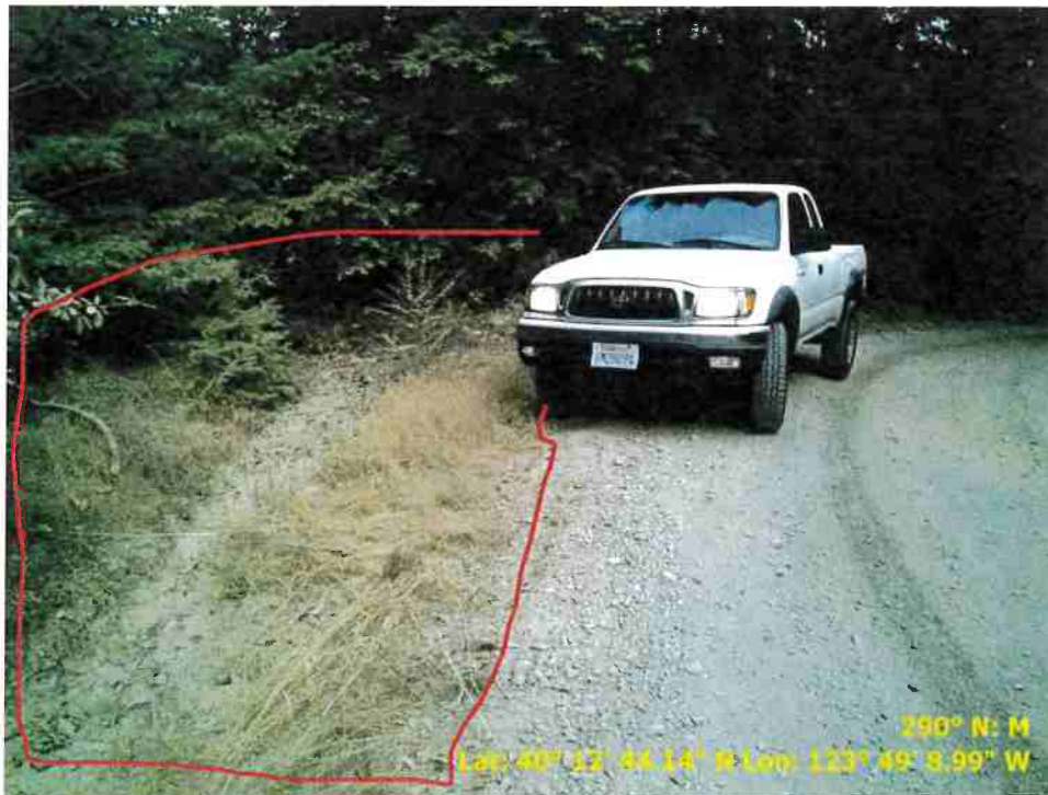
Figure 10. Photograph showing Road Point 31 which is a pullout that need to be regraded.
