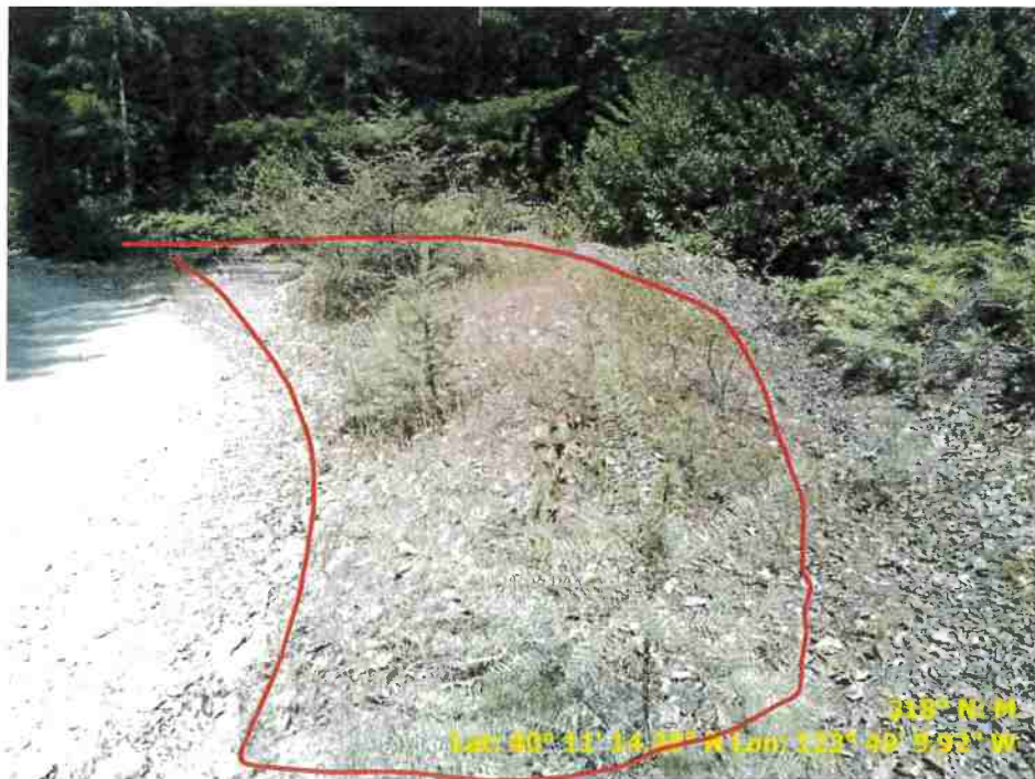
Figure 43. Photo of Road Point 301 showing water-bar/rolling dip that needs surface rock..
