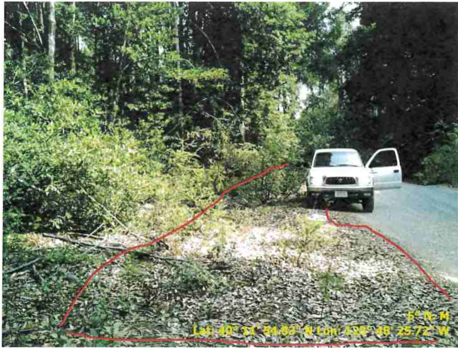
Figure 23. Photo of Road Point 80 showing a pullout that needs to be regraded and vegetation cleared.
