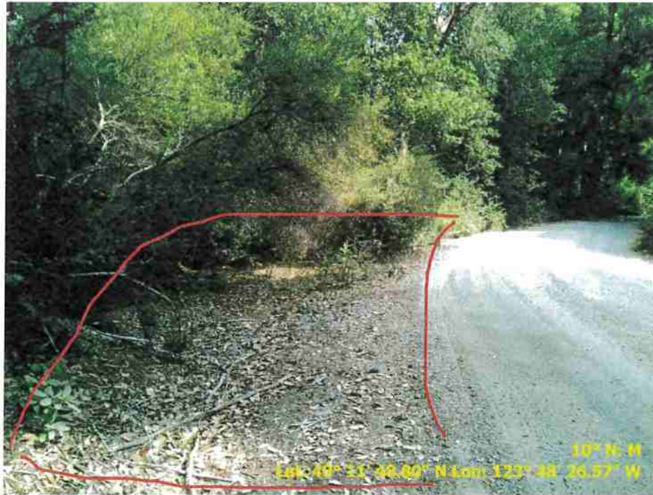
Figure 25. Photo of Road Point 91 showing a pullout that needs vegetation cleared and to be regraded.
