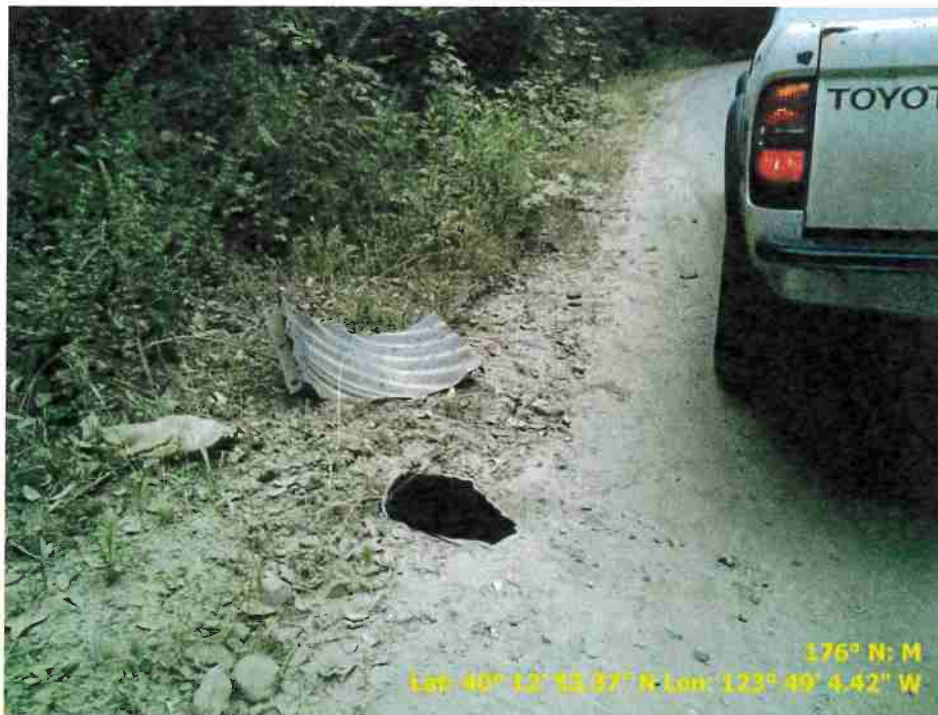
Figure 6. Road point 15 shows an 18" drainage relief culvert with and exposed opening that needs to be repaired or replaced.
