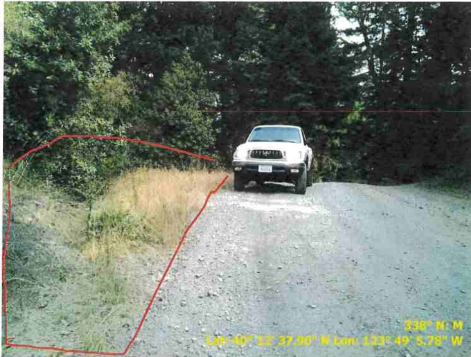
Figure 11. Photograph showing Road Point 40 which is a pullout that need to be regraded.
