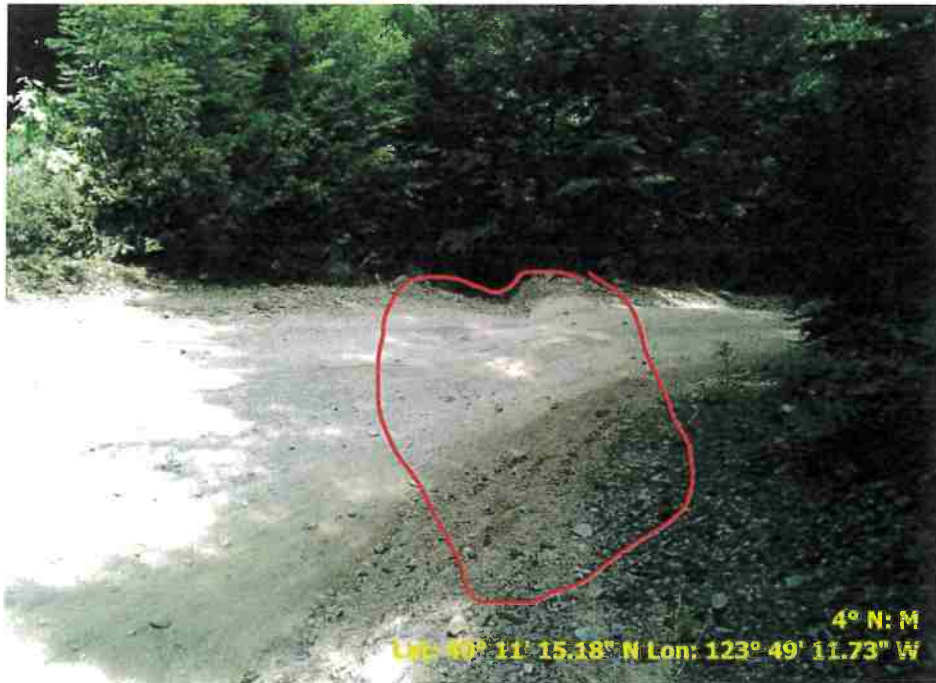
Figure 43. Photo of Road Point 301 showing water-bar/rolling dip that needs surface rock..
