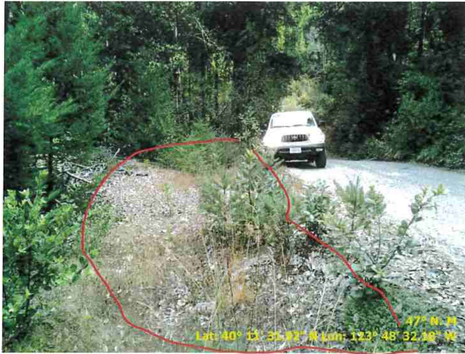
Figure 33.. Photo of Road Point 110 showing a pullout that needs to be cleared of vegetation and regrading.
