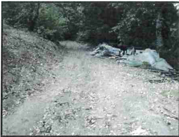
Placement of rolling dip to convey water off of road surface
