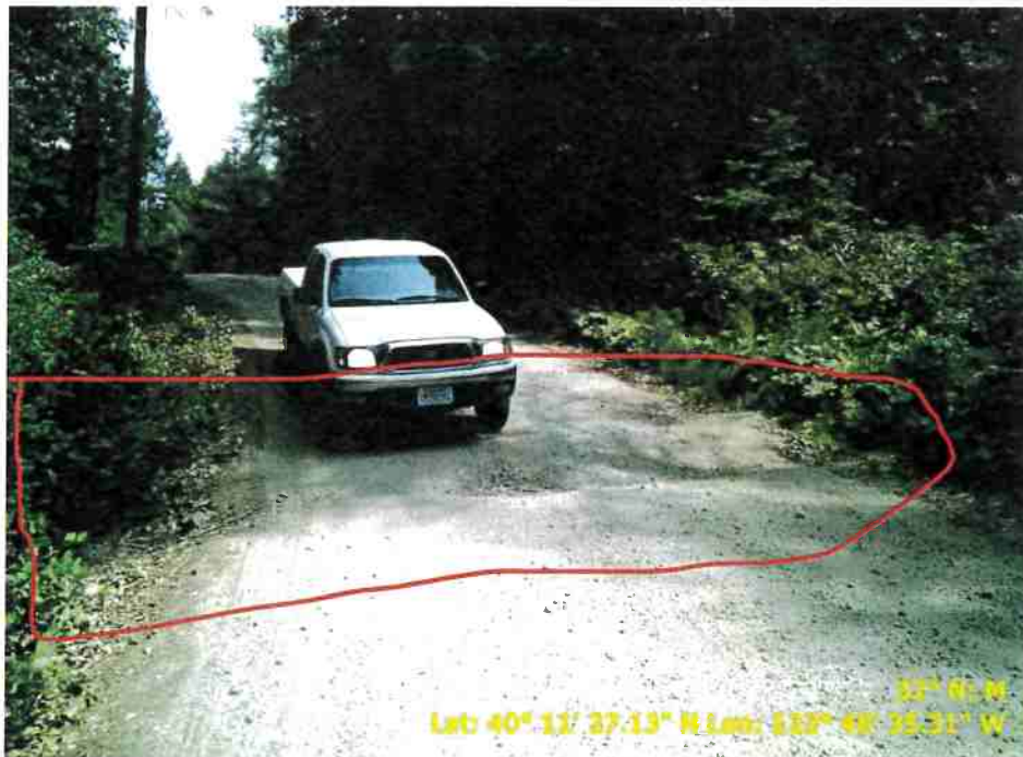
Figure 34. Photo of Road Point 112 showing where concentrated road runoff crosses the road. The fix is to install a culvert or a rocked rolling dip.
