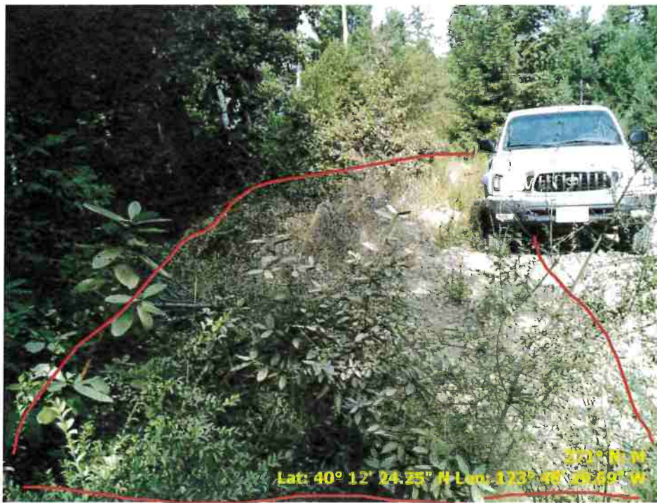
Figure 16. Photo of Road Point 74 showing a pullout that needs to be regraded and vegetation cleared.
