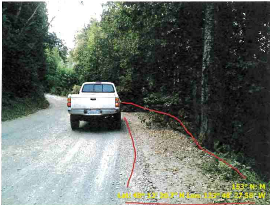
Figure 18. Photo of Road Point 77 showing a pullout that needs to be have a stump cleared and regraded.
