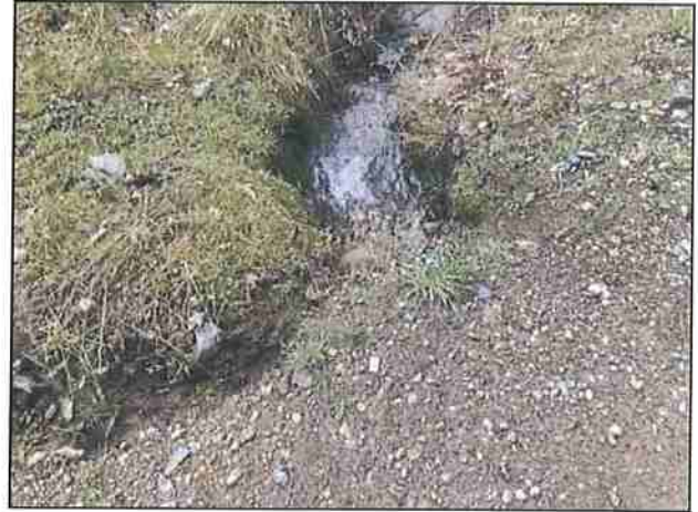
Photo #98 Gorden Rd Looking @ Partially Clogged Culvert Out Size Unknown
