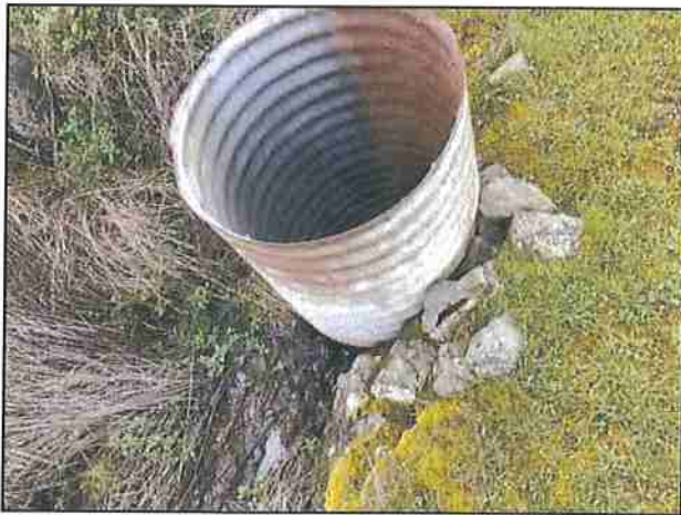
Photo #349 Showers Pass Rd Looking @ 30" Culvert In
