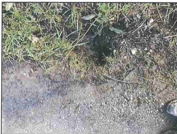
Photo #197 Showers Pass Rd Looking @ Partially Clogged Culvert In (Size Unknown)
