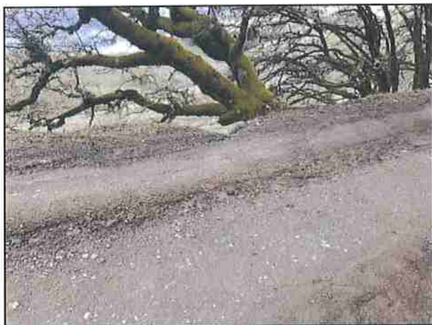
Photo #141 Showers Pass Rd Looking @ Erosion Cazused by Clogged Culvert (Photo 140/142).
