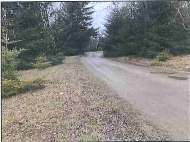
Photo #57 Gorden Rd Slope 0.4% Width 17'7"
