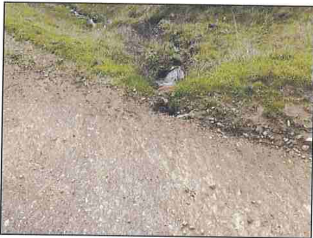
Photo #373 Showers Pass Rd Looking @ Partially Clogged Culvert Out (Size Unknown)
