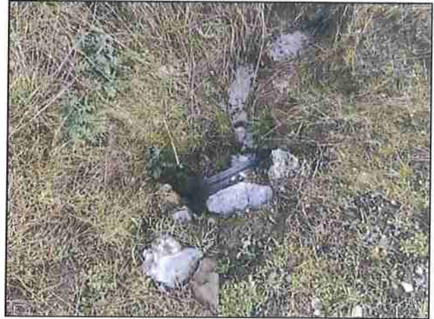
Photo #92 Gorden Rd Looking @ Clogged 24" Culvert In
