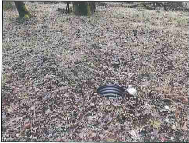
Photo #103 Gorden Rd Looking @ Partially Clogged Culvert Out Size Unknown
