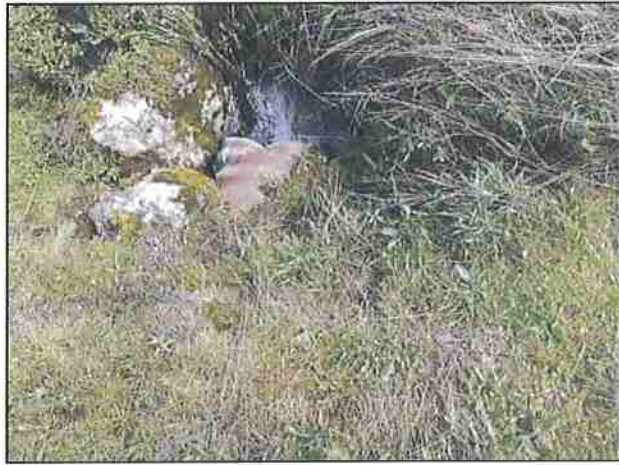
Photo #224 Showers Pass Rd Looking @ 12" Partially Collapsed Culvert In
