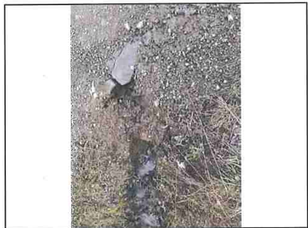
Photo #142 Showers Pass Rd Looking @ Partially clogged Culvert Out (Size Unknown)
