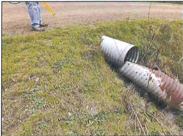
Photo #355 Showers Pass Rd Looking @ Broken Culvert Out (Size Unknown)
