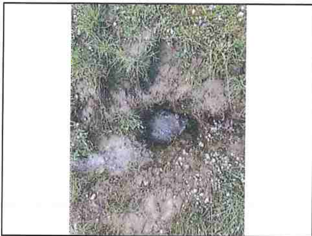
Photo #149 Showers Pass Rd Looking @ Partially clogged Culvert In (Size Unknown)
