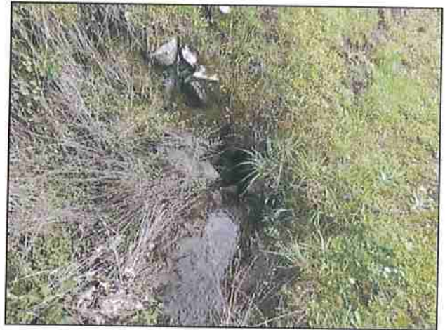
Photo #372 Showers Pass Rd Looking @ Partially Clogged Culvert In (Size Unknown)
