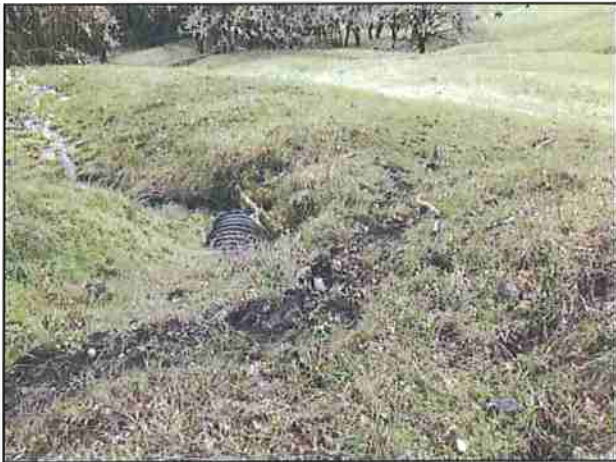
Photo #343 Showers Pass Rd Looking @ Partially Clogged 18" Culvert Out
