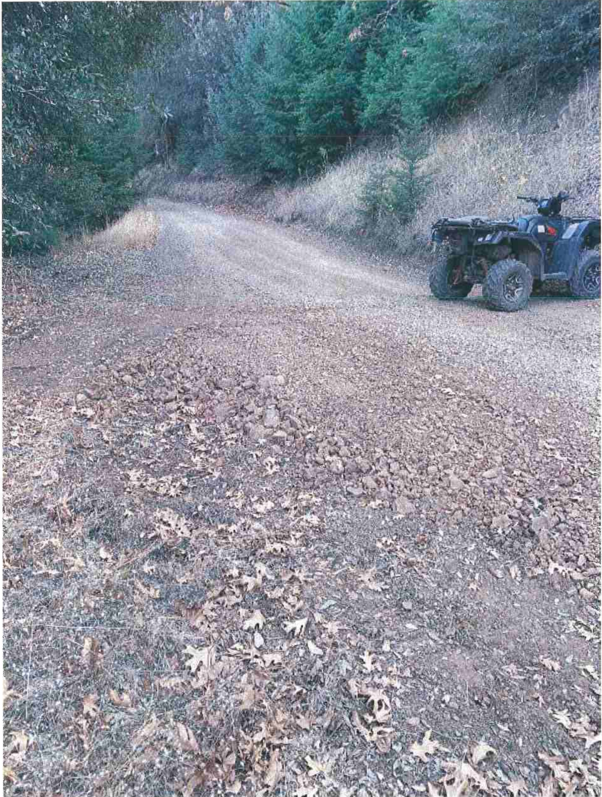
Existing rolling dip; Photographed November 19, 2018
