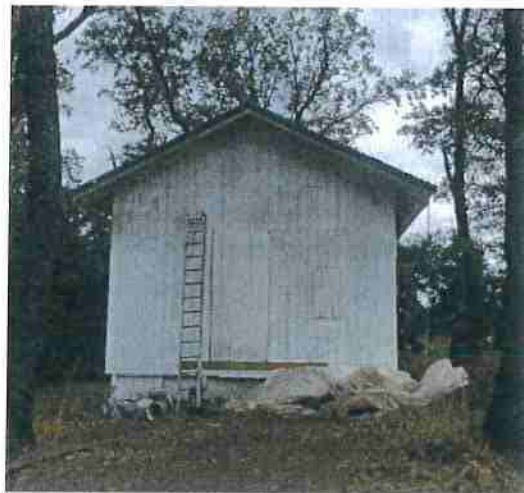
Photo 4: View of the Drying Shed facing northeast.
