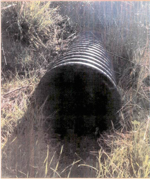
RP6) View of outlet, existing and functional DRC.
