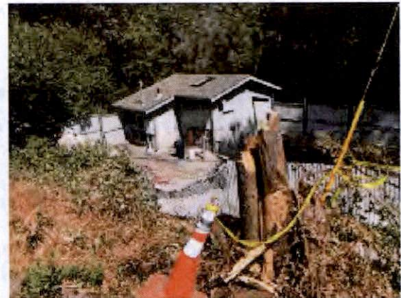
Figure 6. RCSD lift station following a recent vehicular accident.
