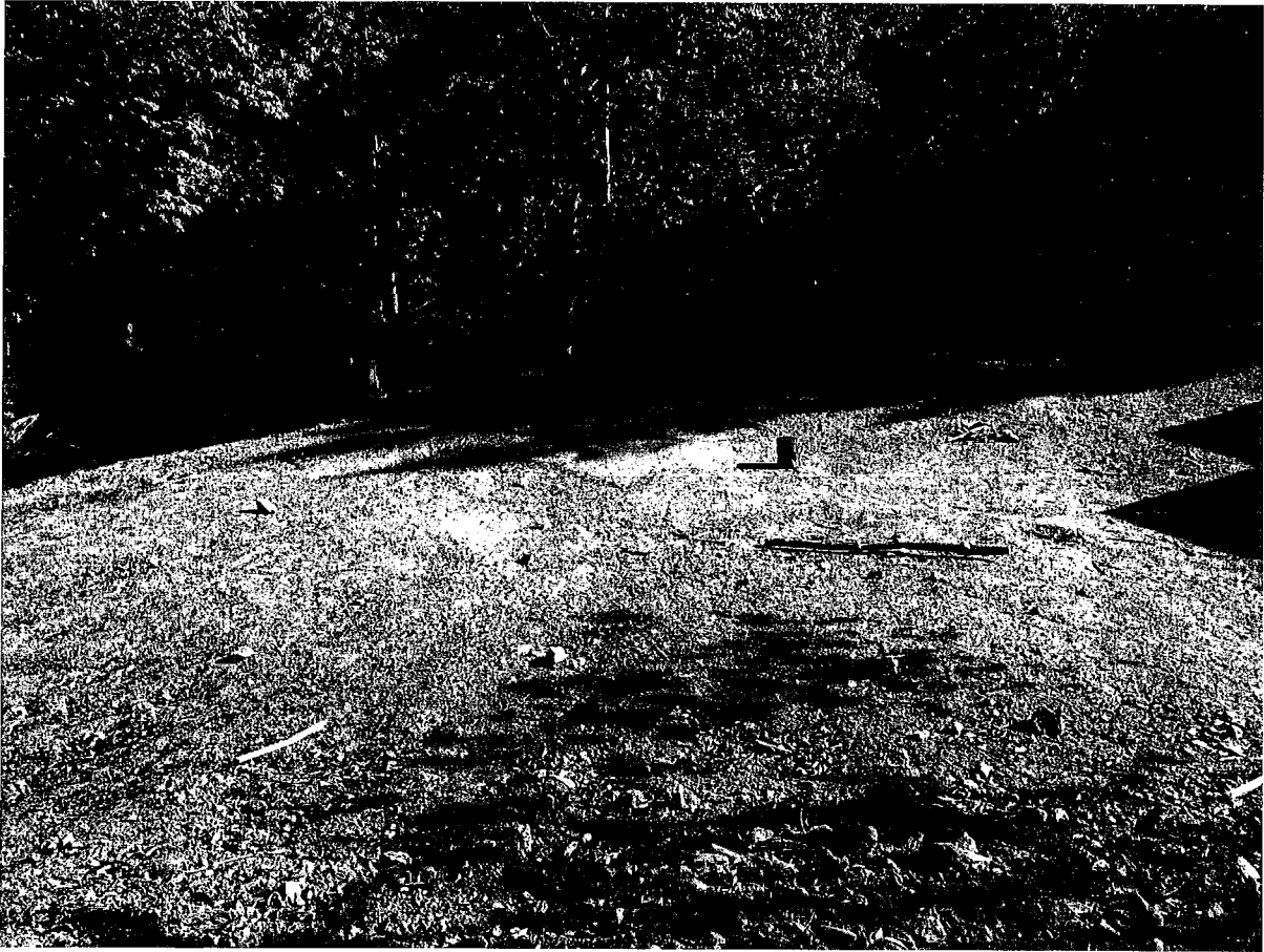
Photo 10. Observation Point C(1) where grading and tree removal occurred within the WLPZ of a Class III watercourse.
