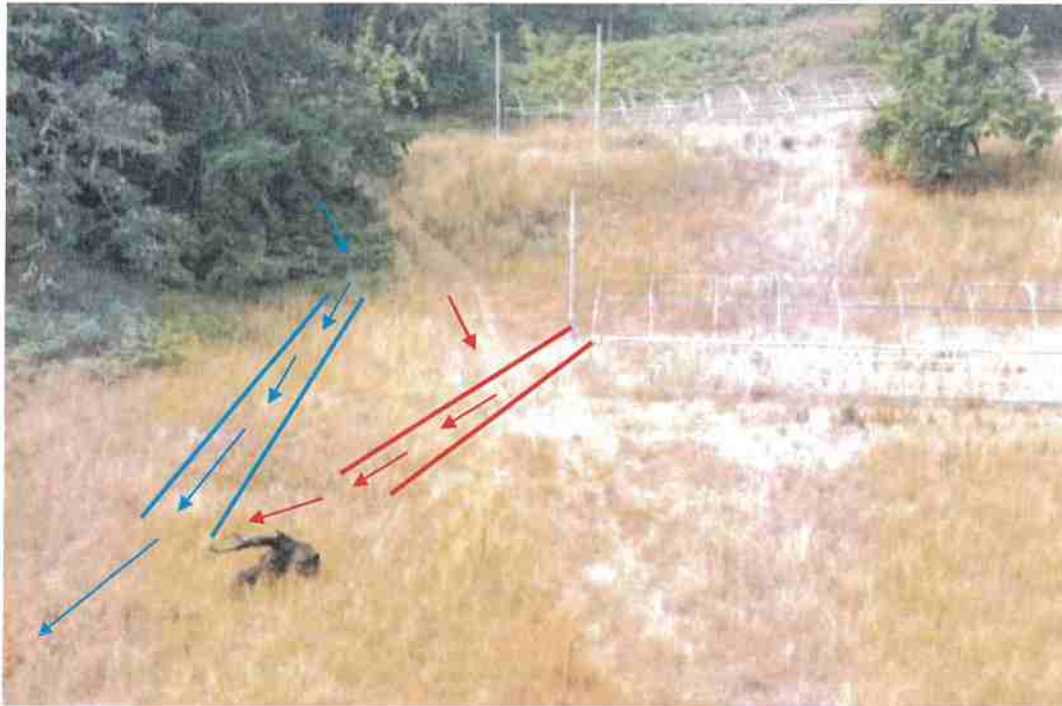
Figure 3: Lower excavation portion of flowpath in blue and with long waterbar on center terrace and road in red
