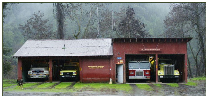
Orleans Fire Engine Bay. Photo: OVFD.
