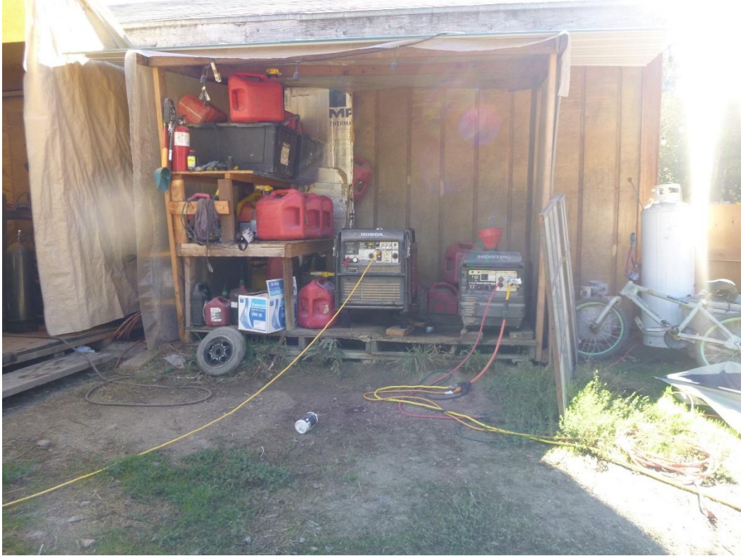
Photo 11. Generator location, no sound blocking material present
