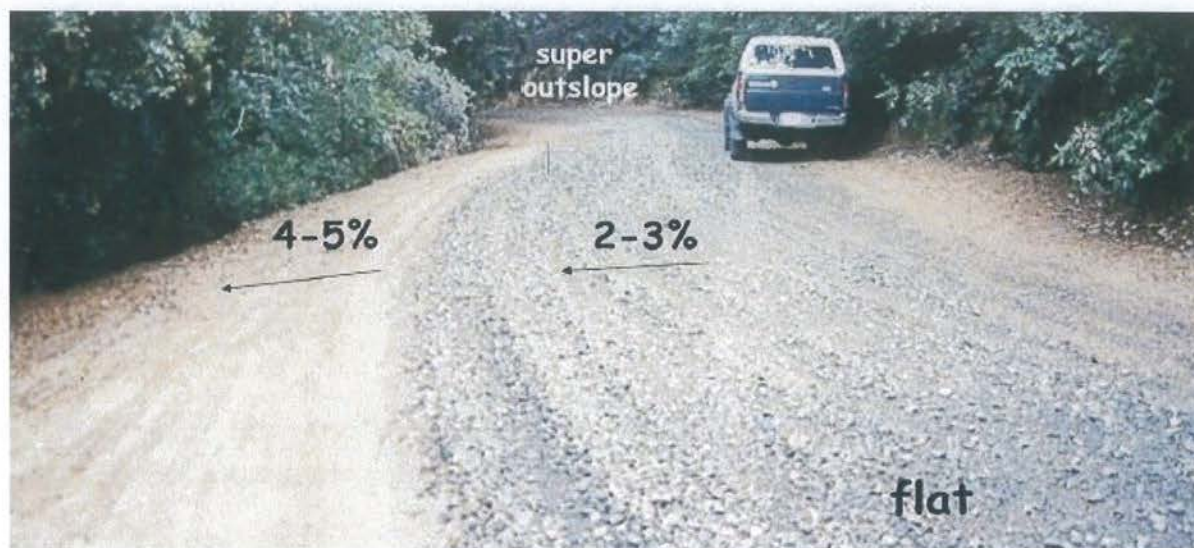
FIGURE 29. Road shape changes as the road travels through the landscape. For example, an out-sloped road will have a steep or "banked" outslope through inside curves, a consistent outslope through straight reaches and a flat or slightly insloped shape as it goes through an outside curve. The road may have an outslope of 2-3% across the travel surface while the shoulder is more steeply outsloped to ensure runoff and sediment will leave the roadbed.
