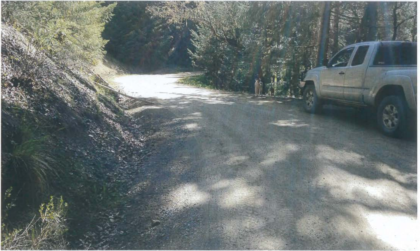
Road Segment 6 to 7: This photo shows the segment of crowned road with an inside ditch from Road Point 6C looking easterly towards Road Point 7. At Road Point 6C, install a rocked rolling dip approximately 30 feet west of the gully below the road. Photo date 4-24-2020.
