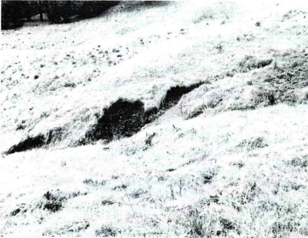
Photo 1. Gully 1 erosion (downslope segment).
