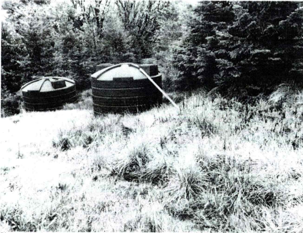
Photo 3. Existing water tanks in wet area at head of watercourse - to be relocated.
