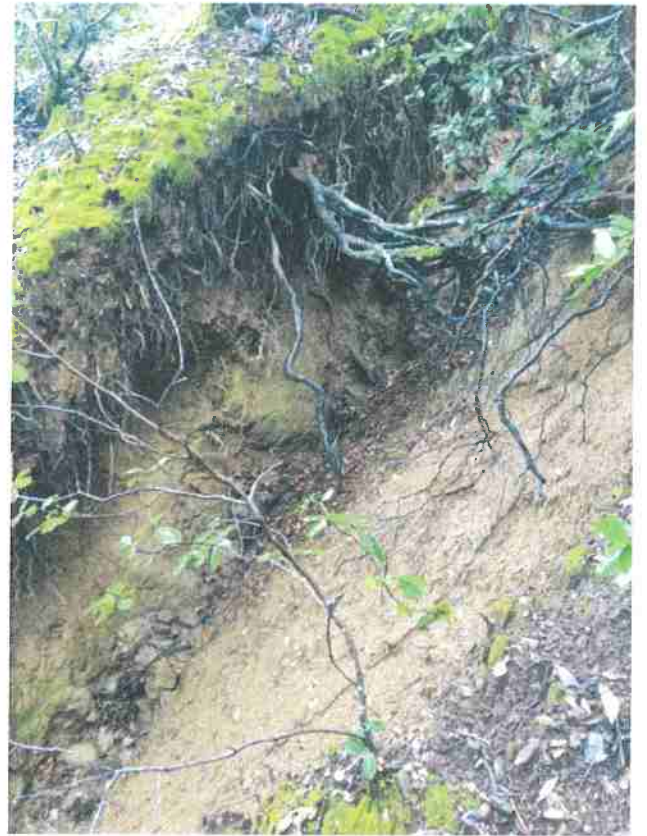
Erosion below discharge point.
