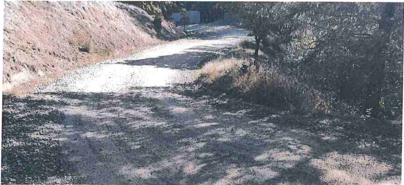
Figure 1: Station 16+01.67 - Slope exceeds Category 2 Standards
