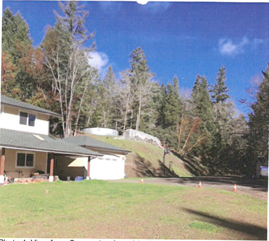
Photo 4: View from Conversion Area A looking north, showing the remainder of the main house on the left and the water tank and cultivation structures of Cultivation Area B in the center.
