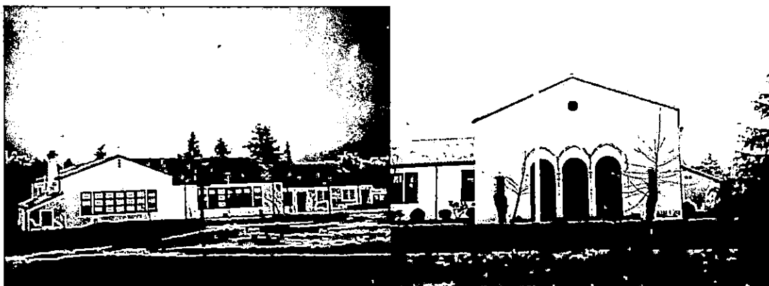
Garberville Elementary School (no date)
