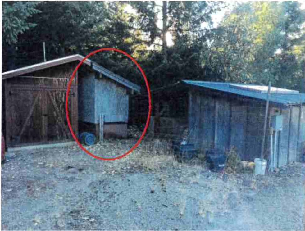
Photo 6. Generator storage, industrial generator circled
