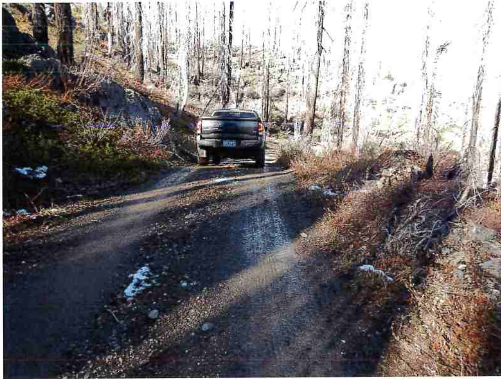
Photo 27: RP 14. Vehicle traveling north, photo taken facing north.
