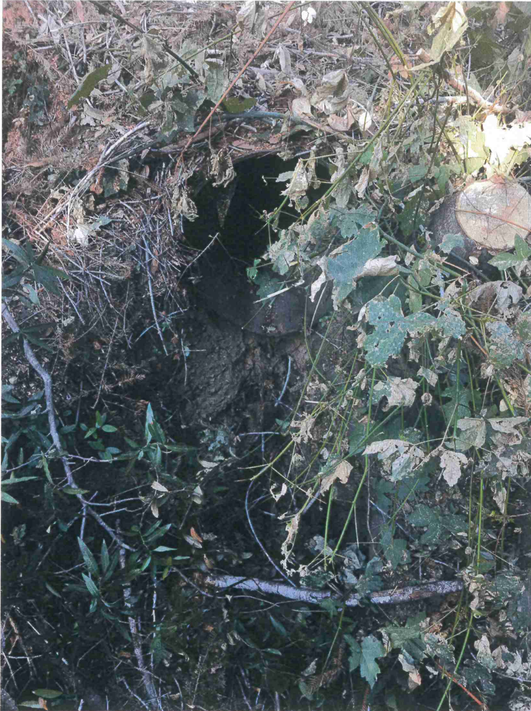
Picture 8: Outlet of Crossing #2. Photo date 8-13-2019
