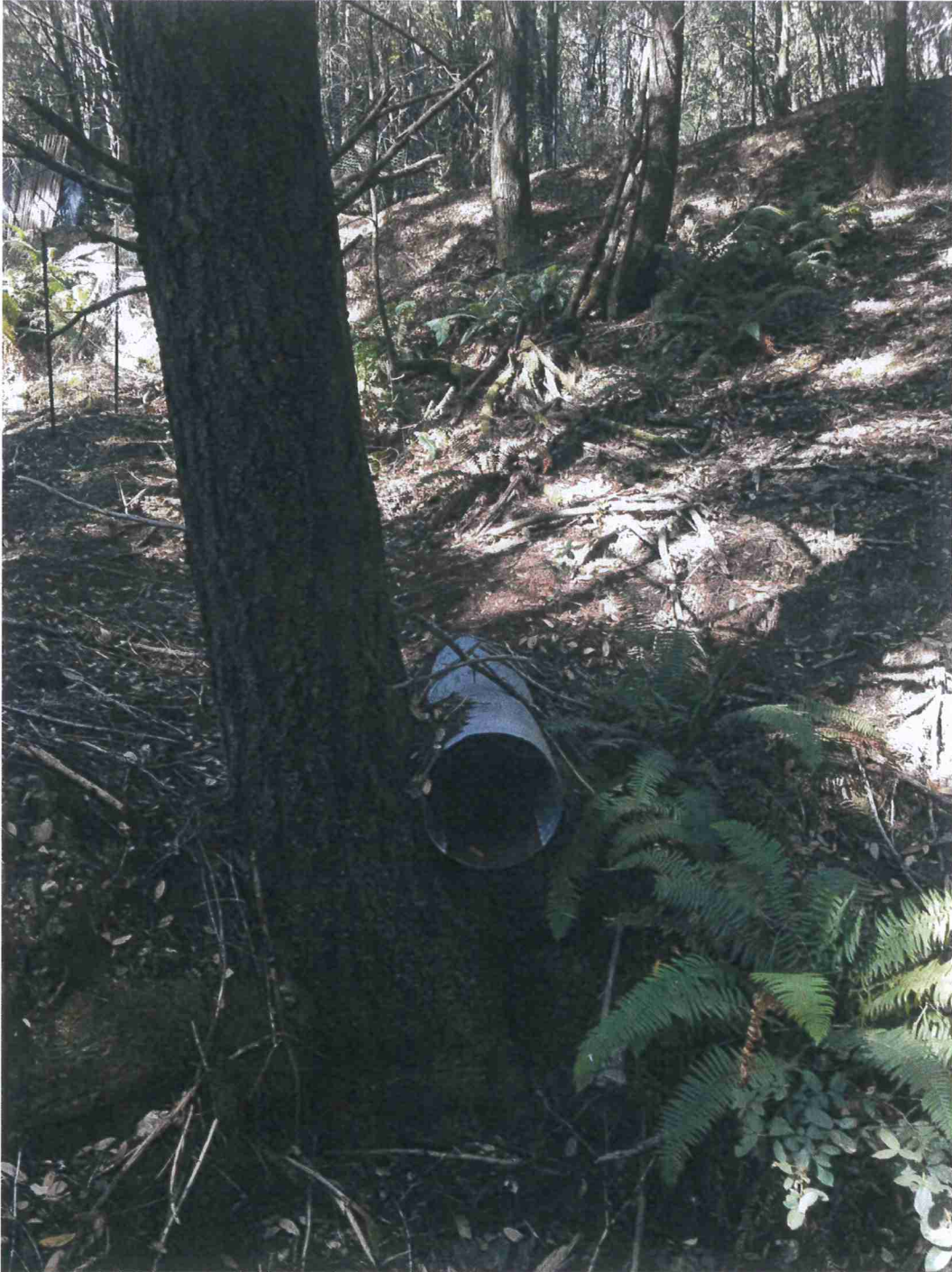
Picture 11: Outlet of Crossing #3. Photo date 8-13-2019
