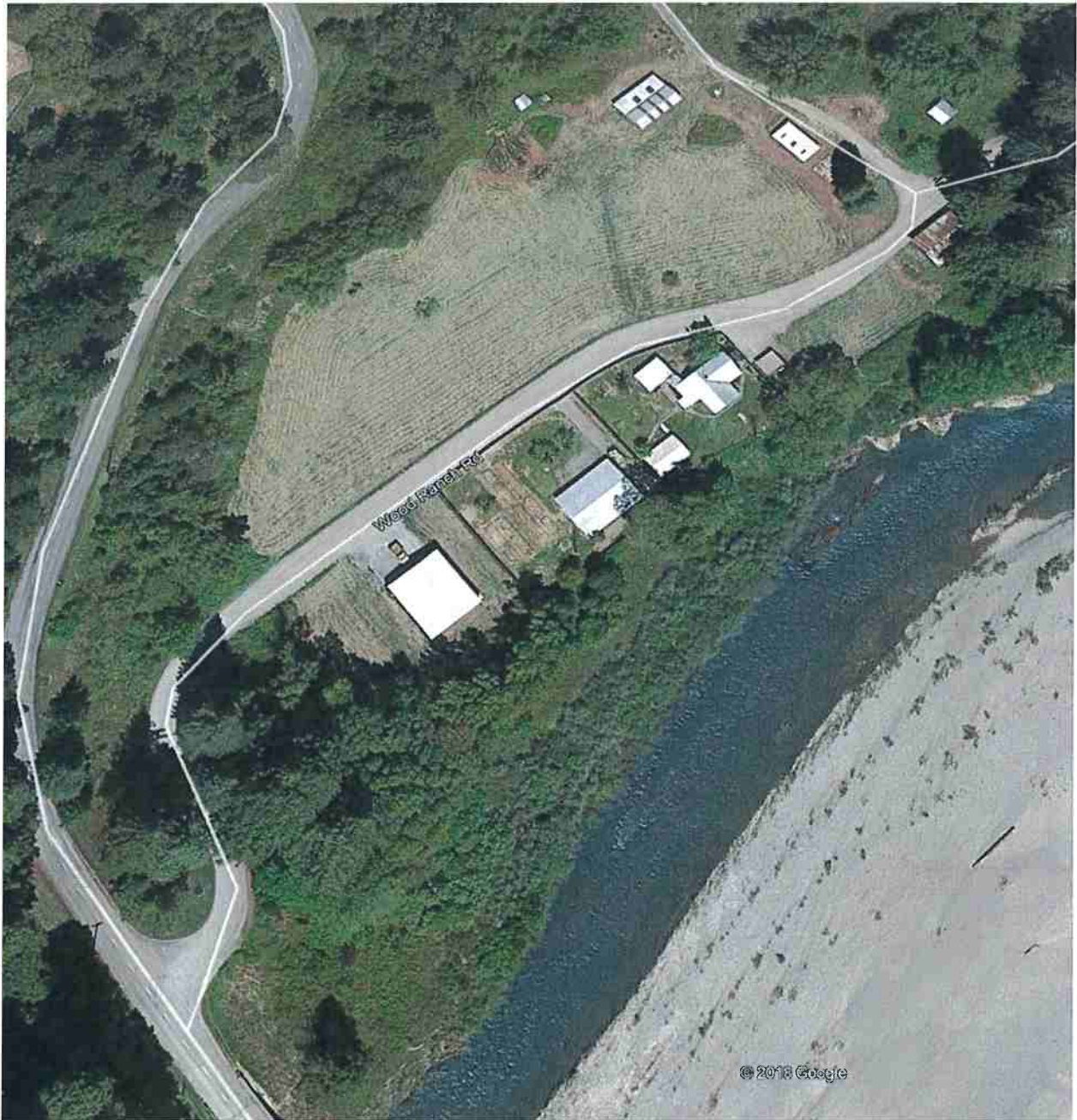
RS1 – The beginning segment of Wood Ranch Road averaging 25' wide for approximately 200 yards.
