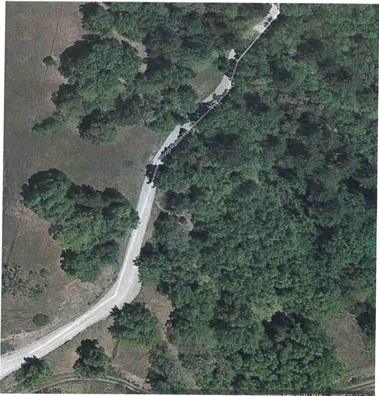
RS3 – The road width at this curve is 22 feet; there is significant pull-out area.
