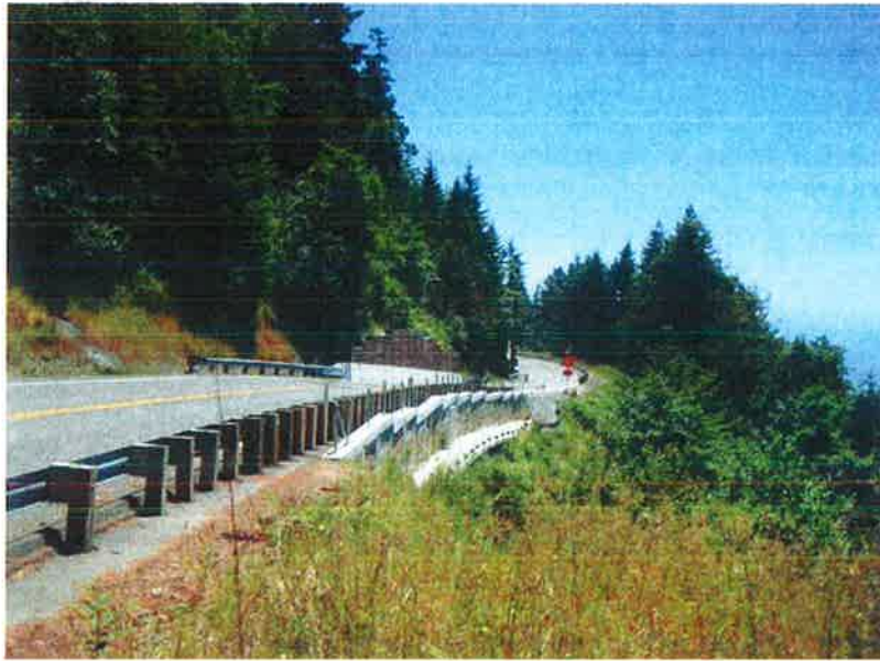
Similar soldier pile retaining wall post construction.
