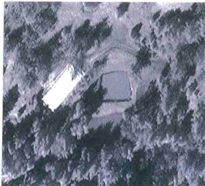
Figure 14: "North Pond" immediately following installation of a liner 3-12-2017.
