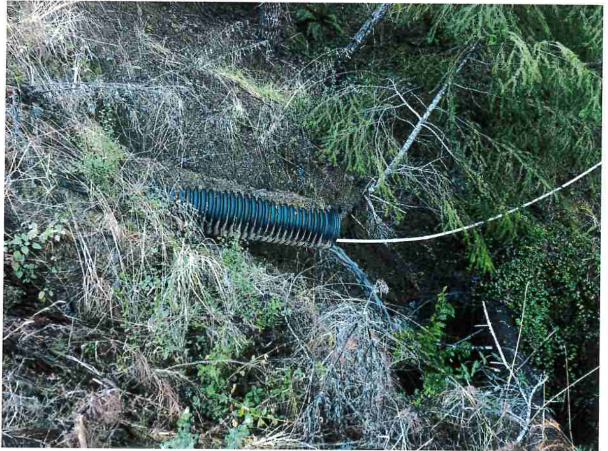
First Culverted Watercourse Crossing, South Of The Dwelling
