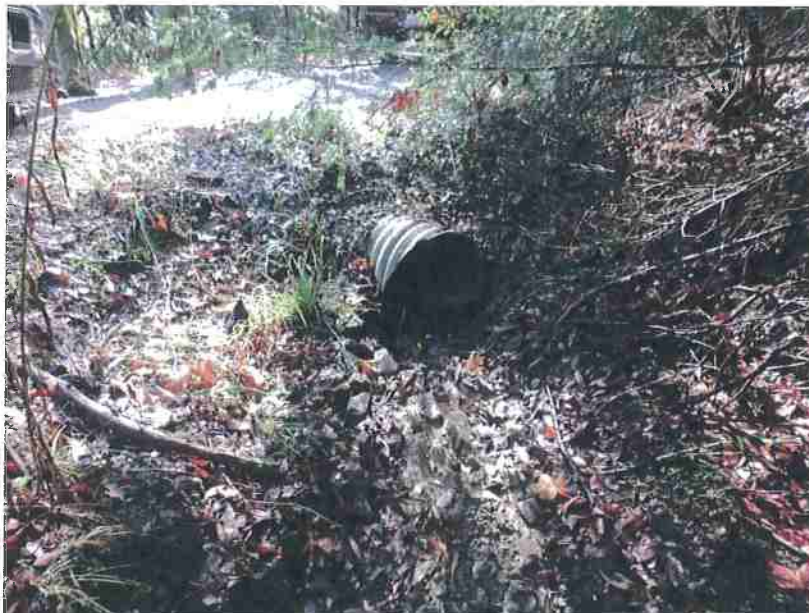
Photo 9. Stream Crossing #4, view of Stream channel entering culvert inlet. Culvert receives sediment contribution from nearby quarry which drains to this crossing during rainfall events.
