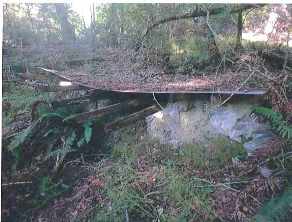
Photo 32. Pond #4 (Guerrilla Pond #2) - View of the concrete embankments, wooden frame and sheet metal roofing of the legacy Guerrilla Pond #2.
