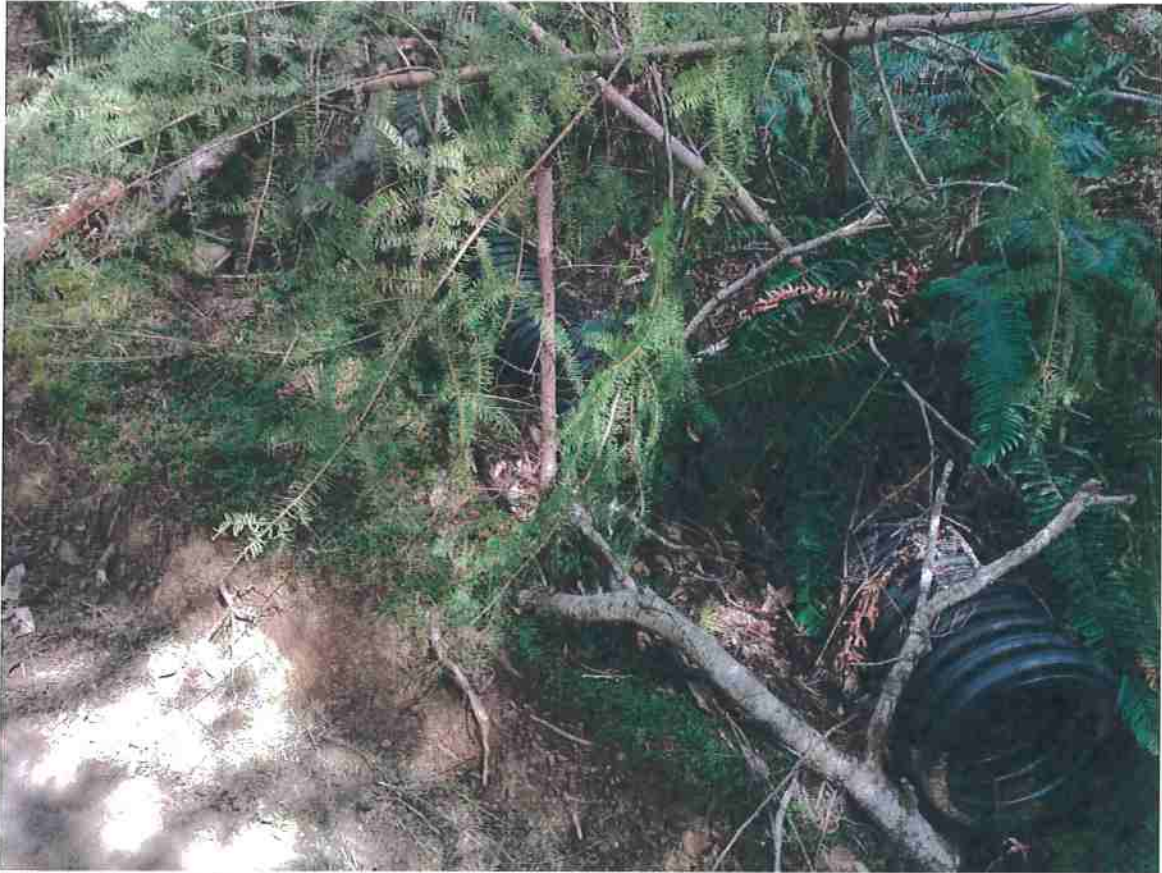
Photo 28. Pond #1-View of Pond #1 spillway culvert outlet. Culvert outlets onto a legacy skid road, which has gullied for several hundred feet down the road before laying out across a natural flat and another legacy haul road.
