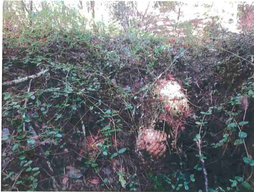
Photo 4. Stream Crossing #2, view of culvert outlet placed short and high in the fill. Culvert is not properly aligned with the natural grade of the stream channel, and outlets water onto rock and fill material.
