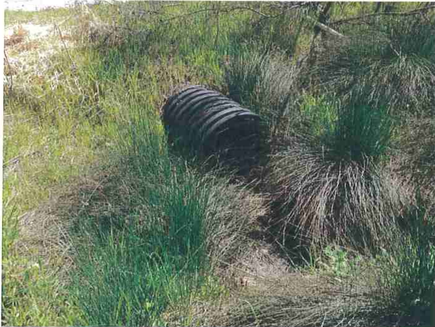
Photo 19. Stream Crossing #8, view of 18-inch diameter culvert. Culvert is properly aligned with the natural grade of the stream channel.
