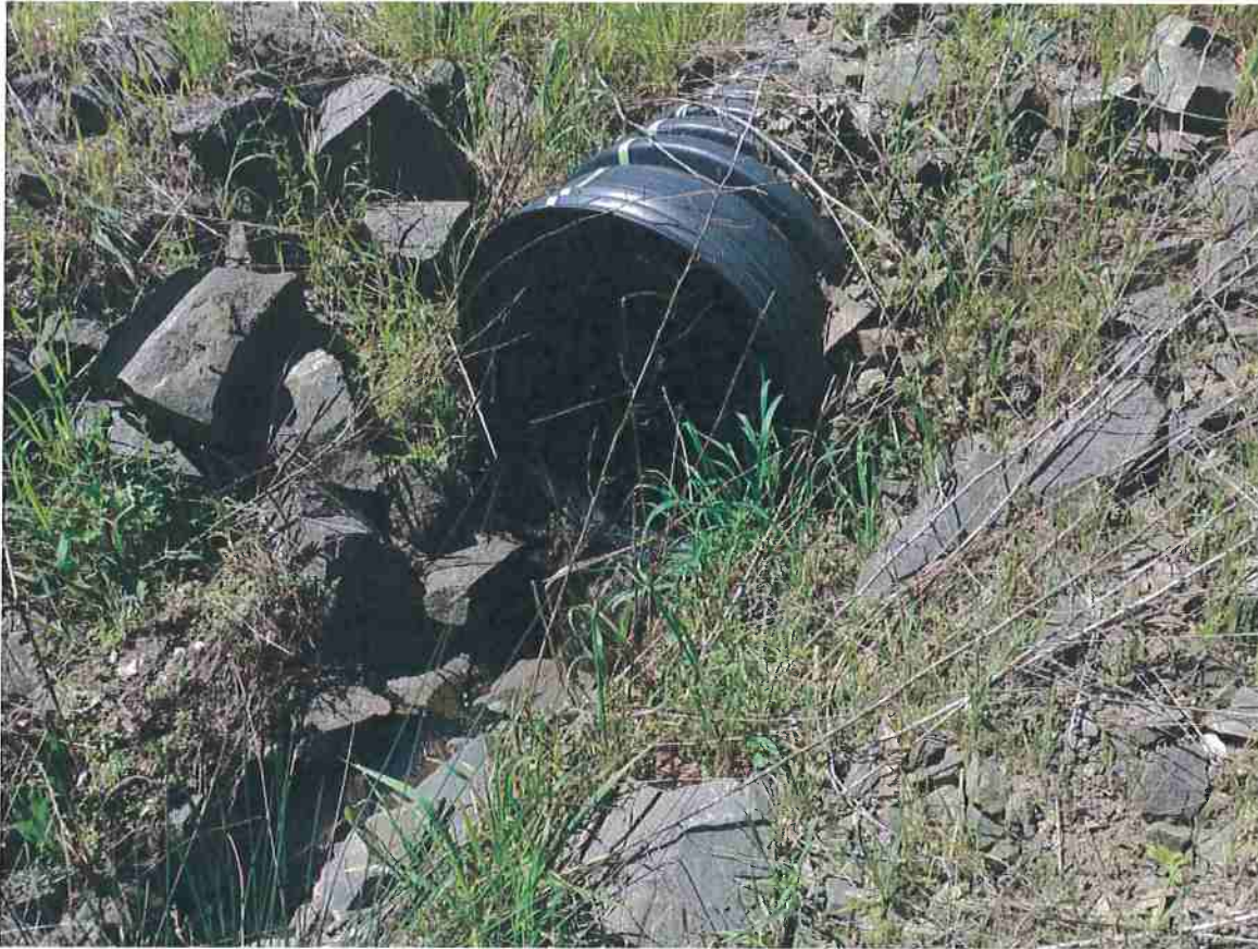
Photo 21. Stream Crossing #8, view of outlet. Stream flow exits culvert onto 6" minus angular rock apron.
