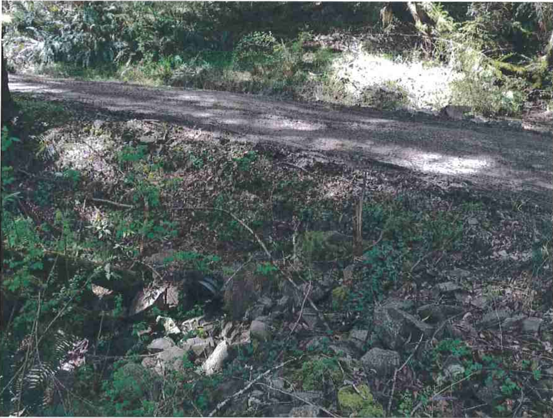
Photo 14. Stream Crossing #6, view of culvert outlet placed short in the fill. Culvert is properly aligned with the natural grade of the stream channel, and outlets water onto rock armor. OBF is armored to prevent erosion. Legacy waste was observed in the channel (tire).
