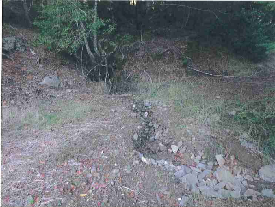
Photo 22. Stream Crossing #9, upstream view of gully incised into a legacy road resulting from a buried culvert inlet. A Class II stream still flows through the 12-inch diameter plastic culvert outlet, and overtops during high flow events following the gully path back into the channel.
