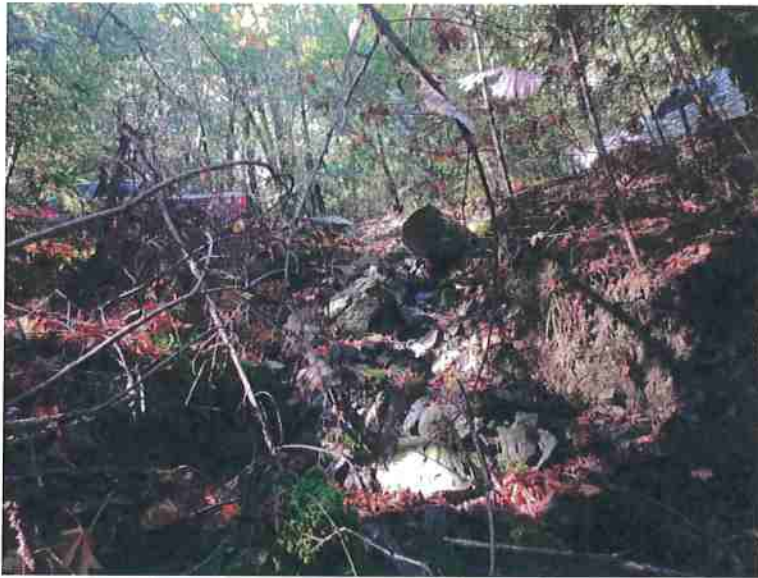
Photo 10. Stream Crossing #4, view of watercourse exiting culvert outlet. Culvert is placed short and high in the fill. Flow path takes an approximate 2-foot plunge at the outlet.
