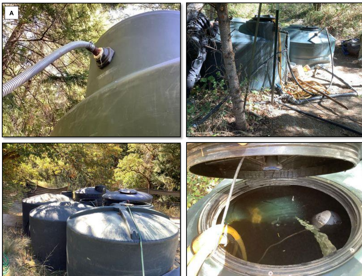
Figure 15. Showing a portion of the water storage tanks on the Property receiving diverted water from Little Larabee Creek. Photo (A) shows the water tank directly connected to water diversion WS-1. Note the gray hose, which was also found near the site of water diversion WS-1 (see Figure 14).
