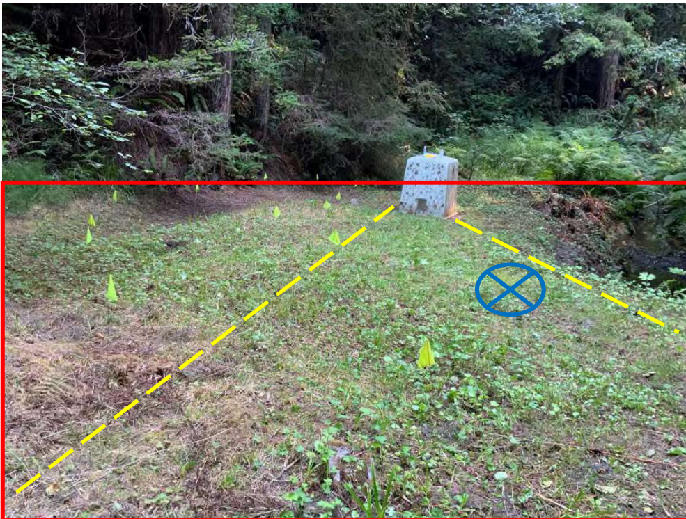
Figure 12. Temporary impact area (red box): palustrine emergent non-persistent wetland (flagged), replacement of utility pipes (yellow dash), and well pump relocation (circle-x)
