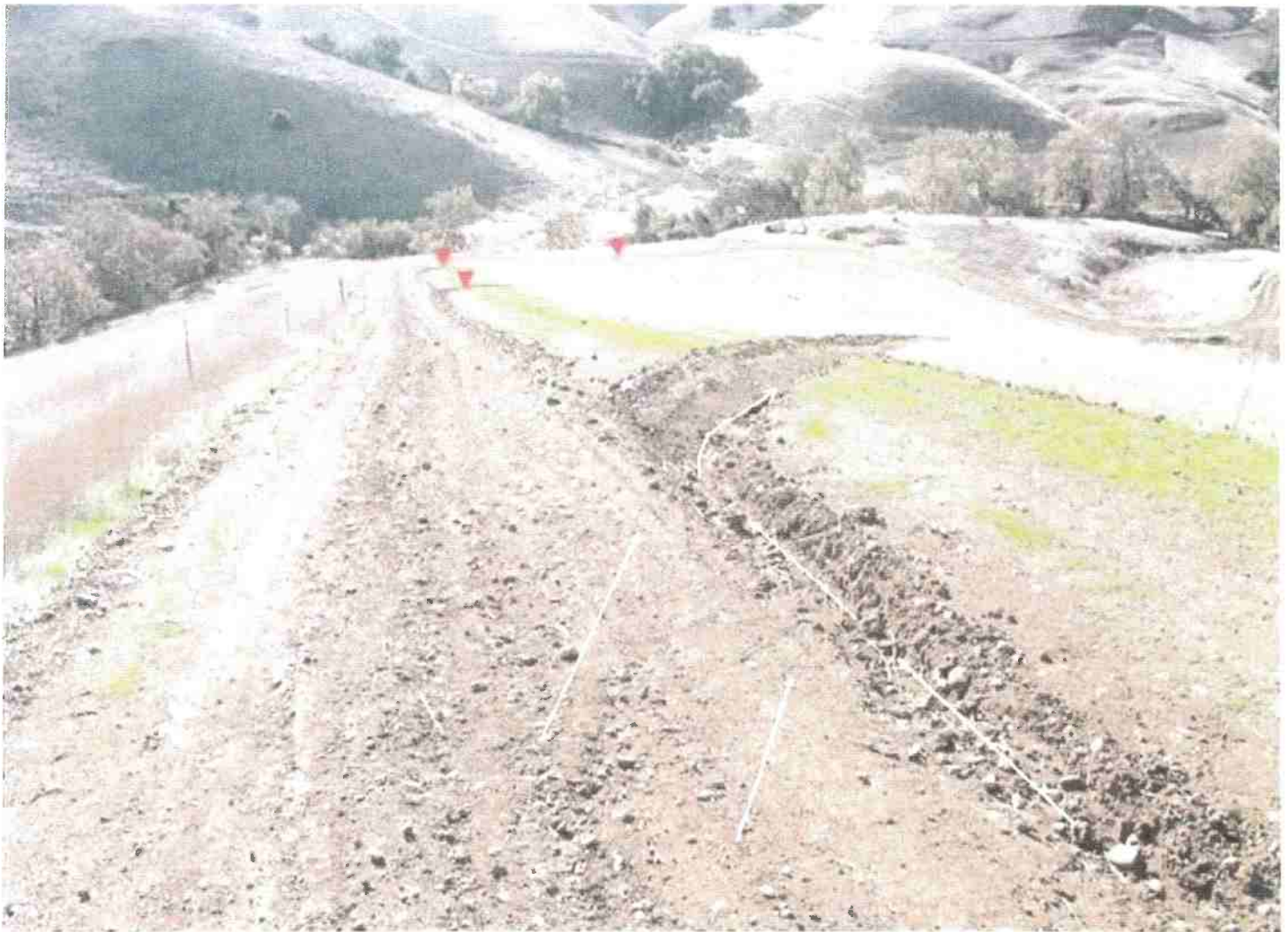
FIGURE 55. Steep roads that go straight up or down a hillside are very difficult to drain. This steep, fall line road developed a through cut cross section that was drained using lead out ditches to direct runoff off the road and onto the adjacent, vegetated hillside. The road was "outsloped" to drain runoff to the right side, and the lead out ditch was built slightly steeper than the road grade, to be self-cleaning. Four lead out ditches have been constructed at 100-foot intervals to the bottom of the hillside.
