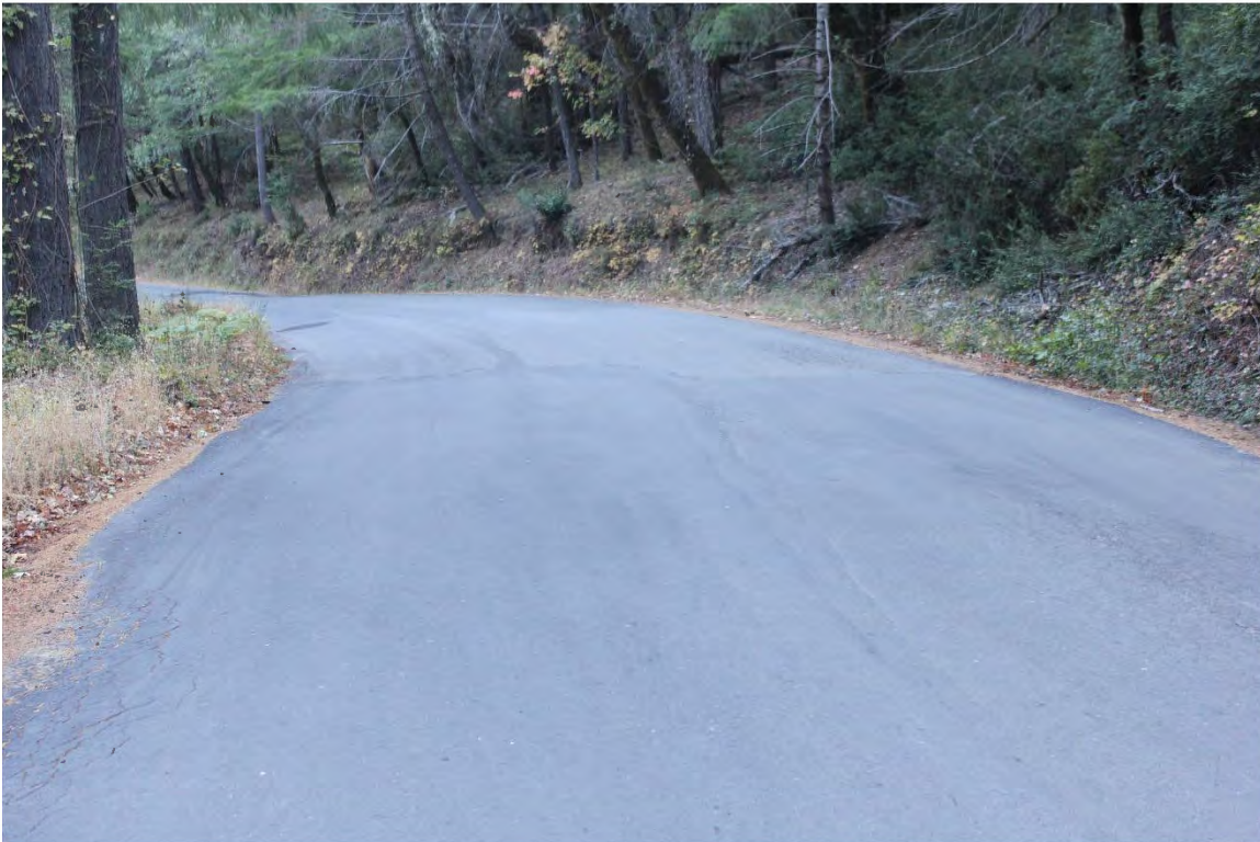
Photo 12. Mile 1.1: 20-ft road width with 2-ft shoulders.
