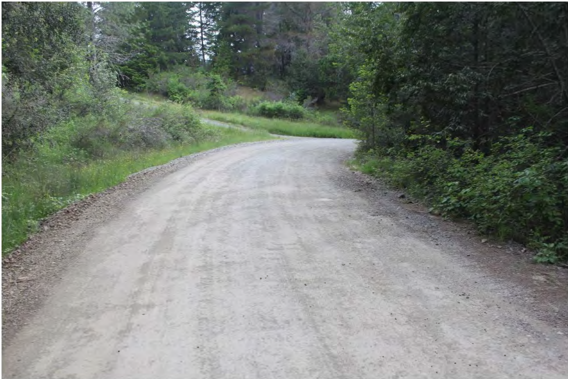
Photo 4. Mile 0.3: 18' width, 1' shoulders.
