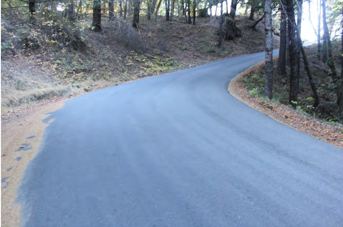
Photo 37. Mile 3.2: 20-ft road width with 2-ft shoulders.
