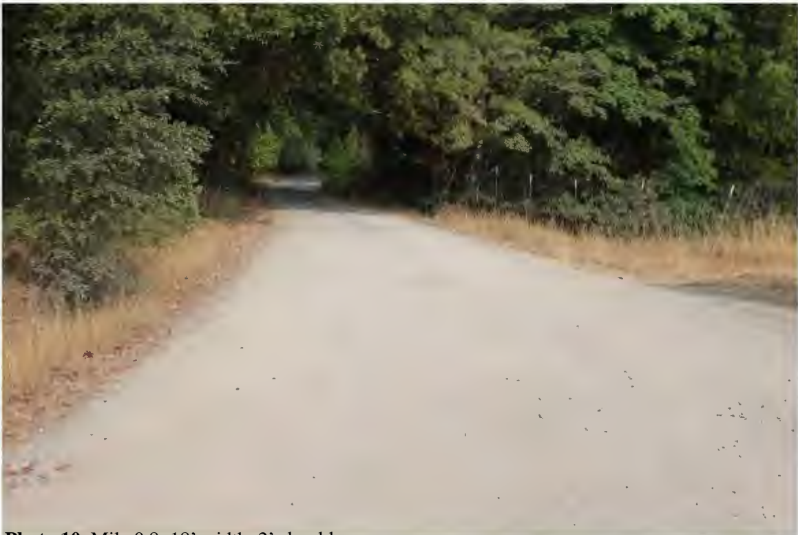
Photo 10. Mile 0.8: 18' width, 2' shoulders.
