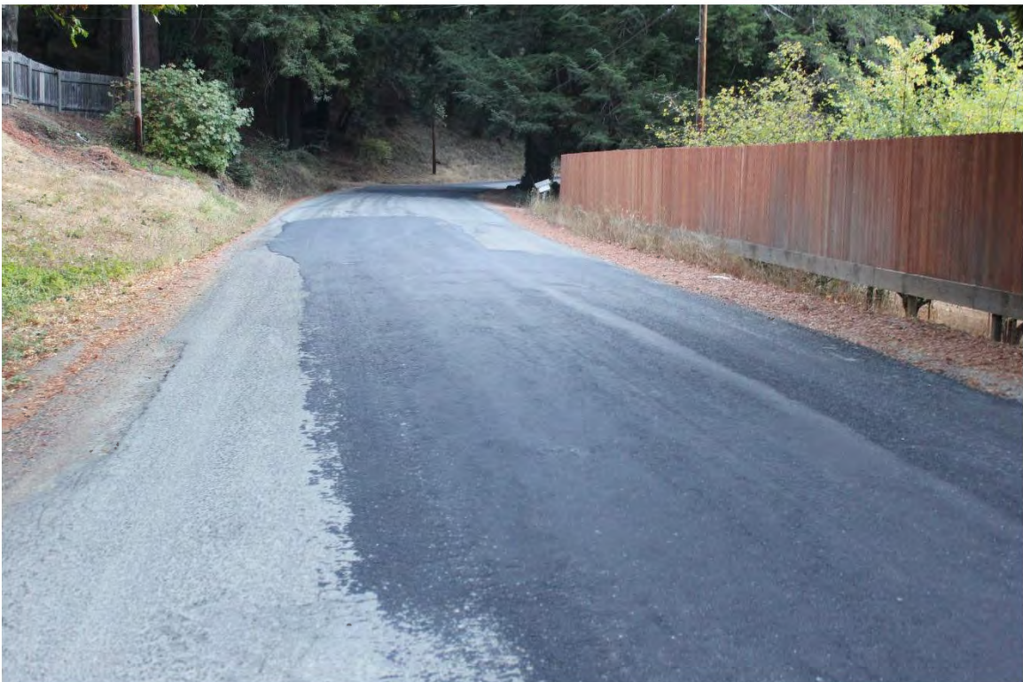
Photo 10. Mile 1.4: 22' width, 2' shoulders.
