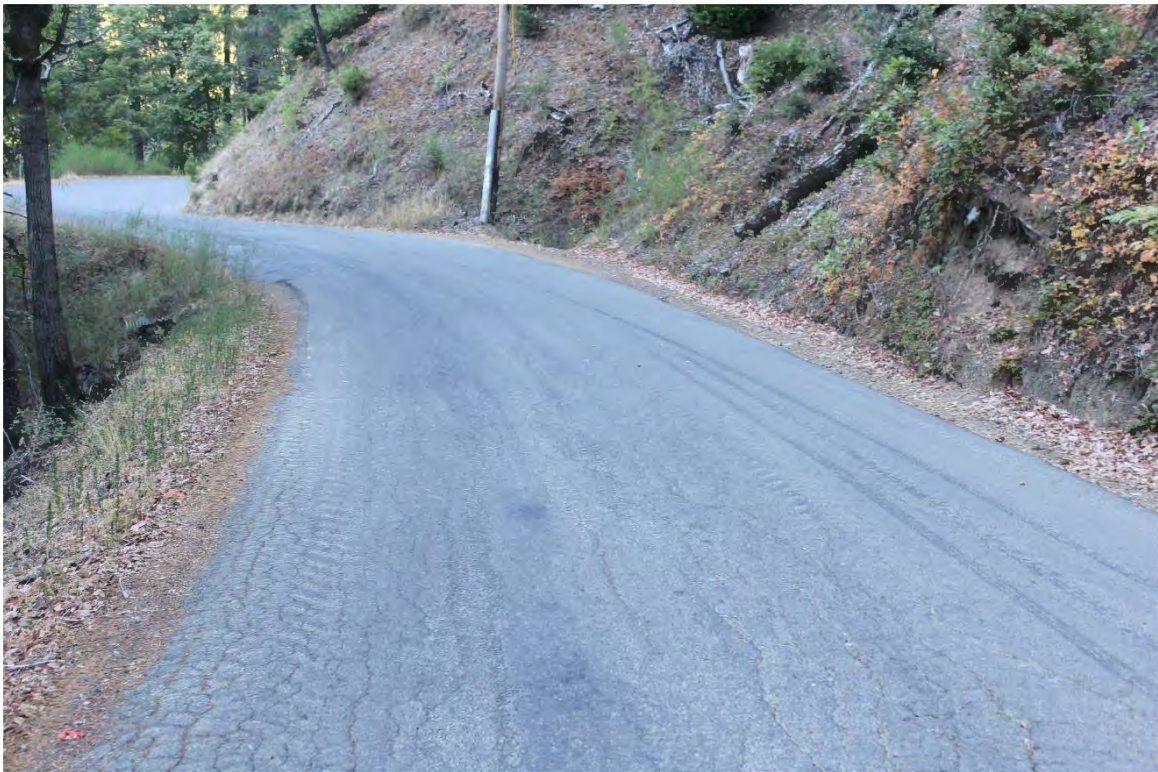
Photo 22. Mile 2.1: 18-ft road width with 1-ft shoulders.
