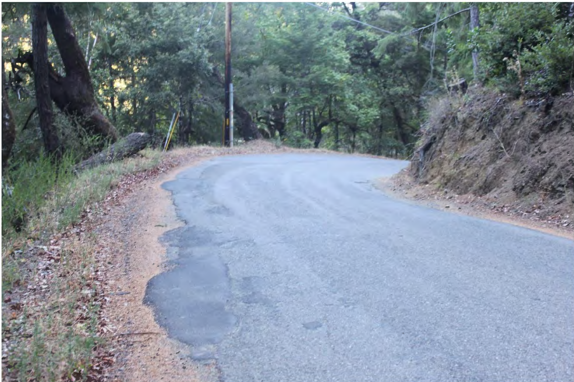
Photo 24. Mile 2.2: 20-ft road width with 1-ft shoulders.
