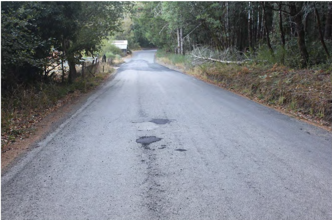
Photo 8. Mile 0.7: 20-ft road width with 2-ft shoulders.
