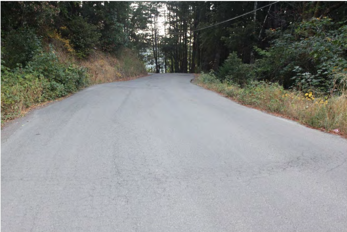
Photo 8. Mile 1.2: 24' width, 1' shoulders.
