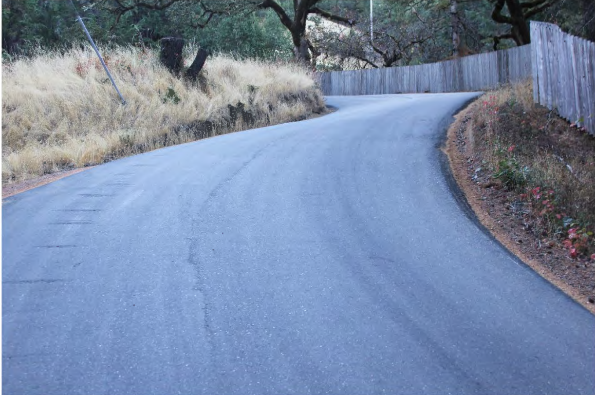
Photo 35. Mile 3.1: 20-ft road width with 1-ft shoulders.
