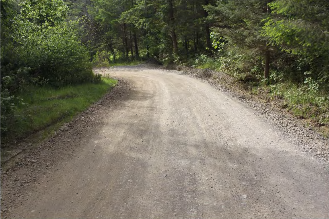
Photo 7. Mile 0.5: 18' width, 1' shoulders.
