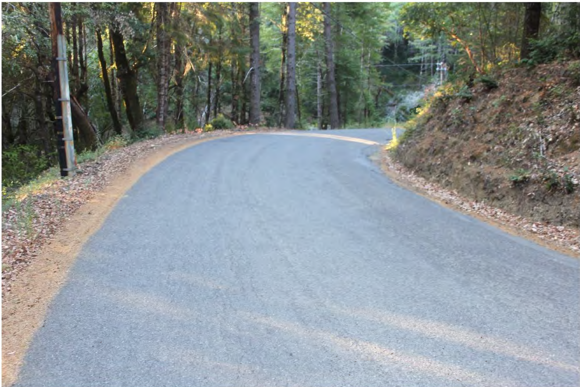
Photo 18. Mile 1.7: 20-ft road width with 1-ft shoulders.
