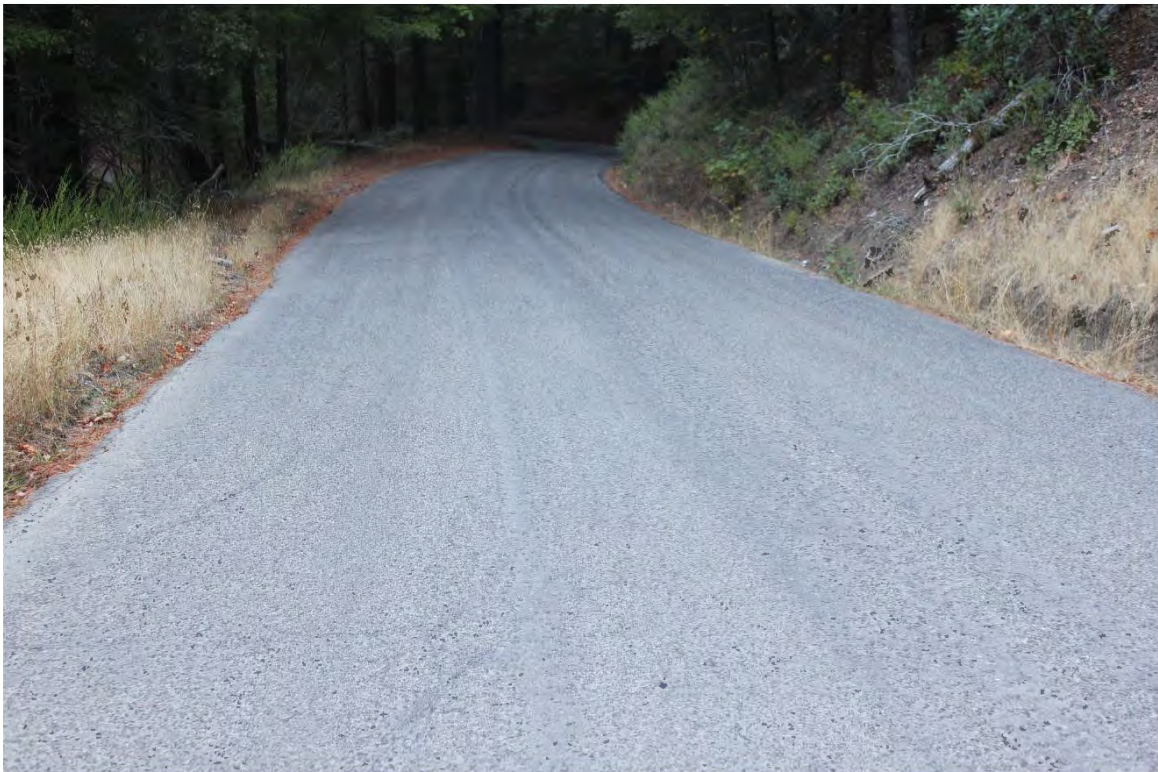
Photo 2. Mile 0.2: 18-ft road width with 1-ft shoulders.
