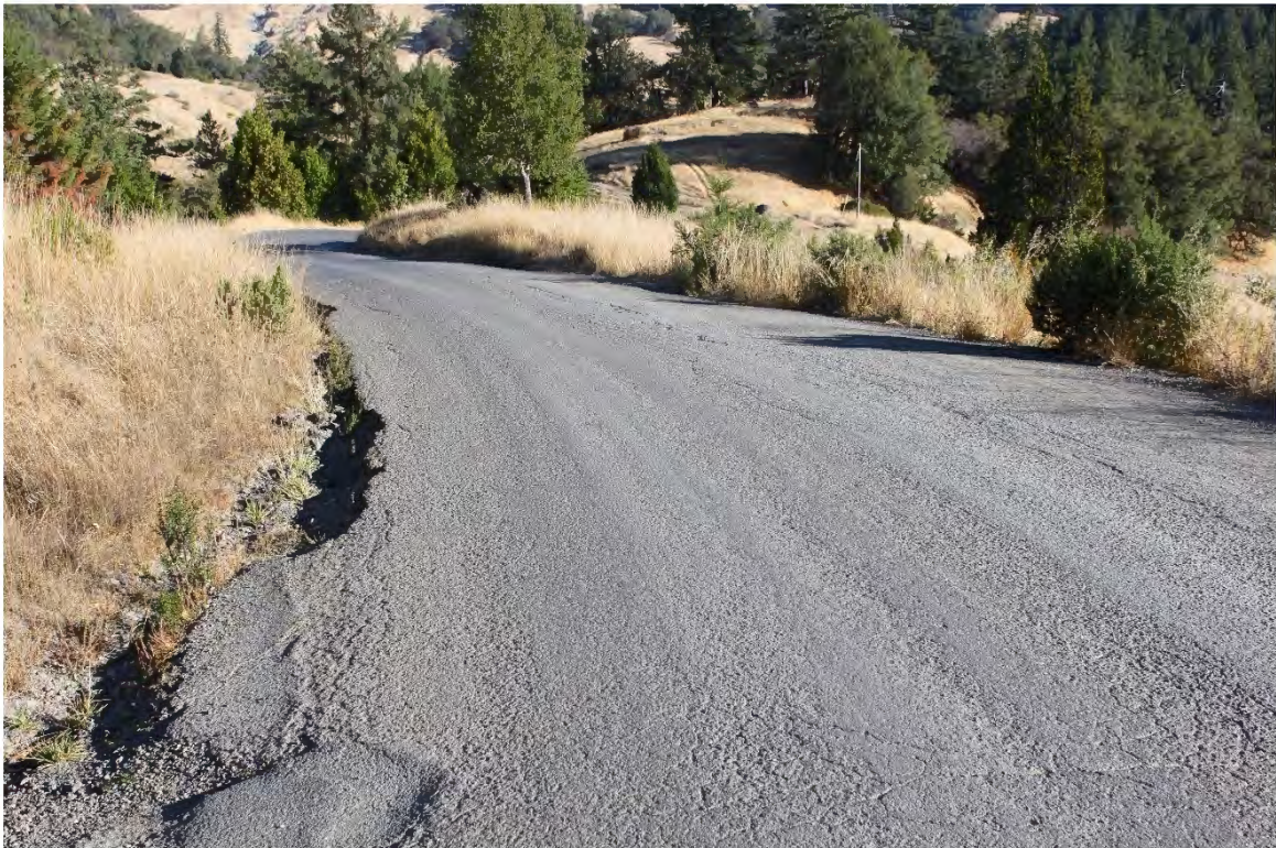
Photo 44. Mile 3.8: 18-ft road width with 1-ft shoulders.
