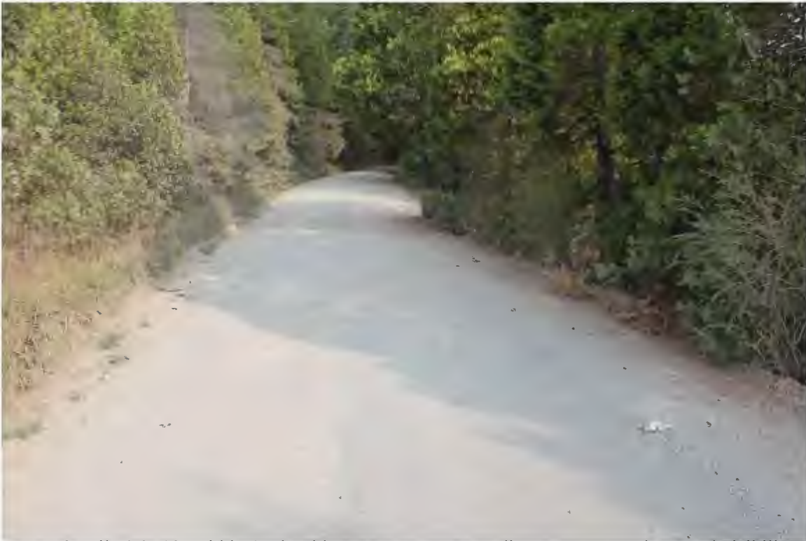
Photo 4. Mile 0.3: 18' width, 1' shoulders, some narrower adjacent segments but good visibility.
