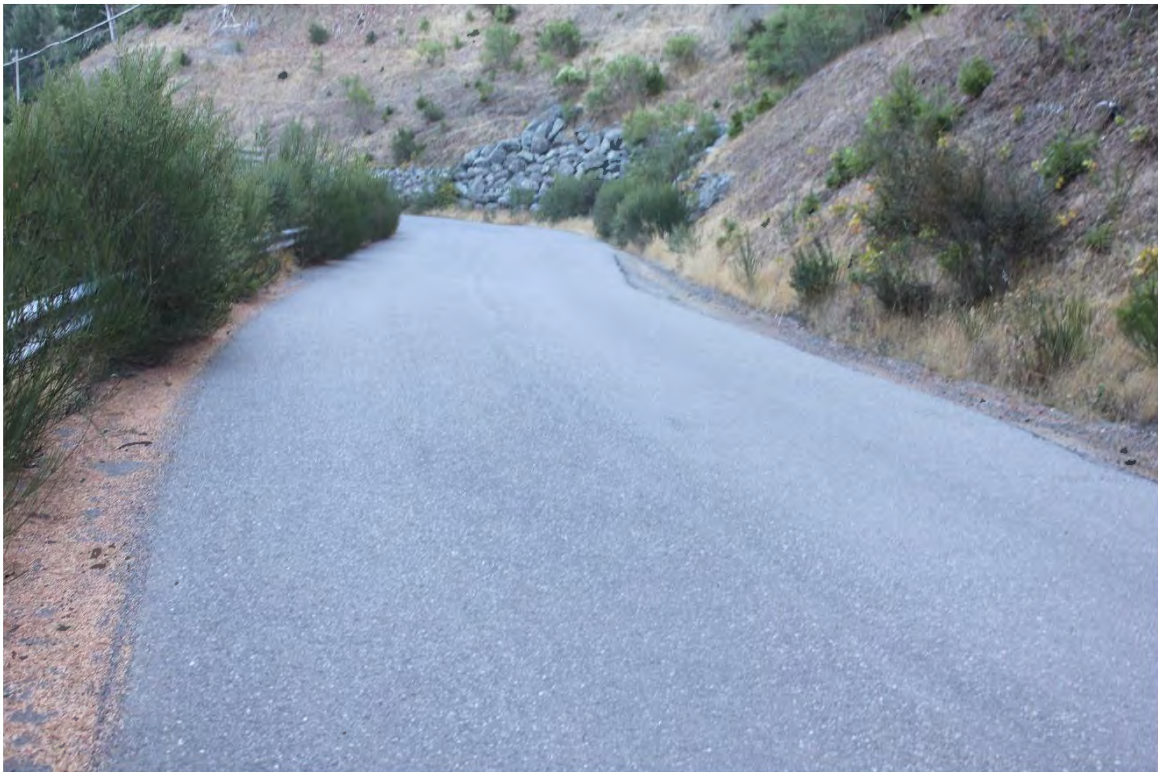
Photo 32. Mile 2.8: 18-ft road width with 1-ft shoulders.
