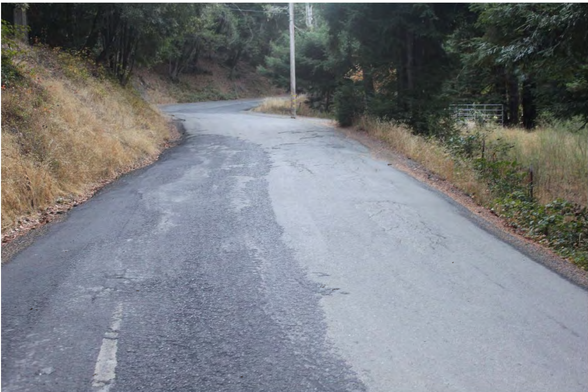
Photo 6. Mile 1.1: 20' width, 1' shoulders.
