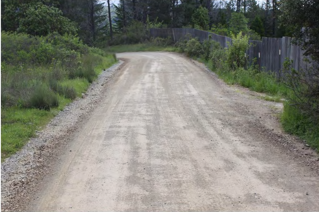
Photo 3. Mile 0.2: 18' width, 1' shoulders.
