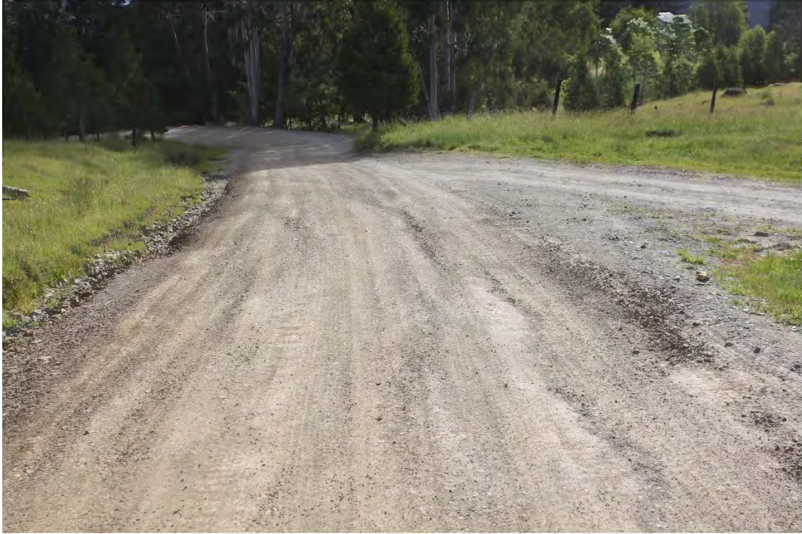
Photo 11. Mile 0.8: 18' width, 2' shoulders.
