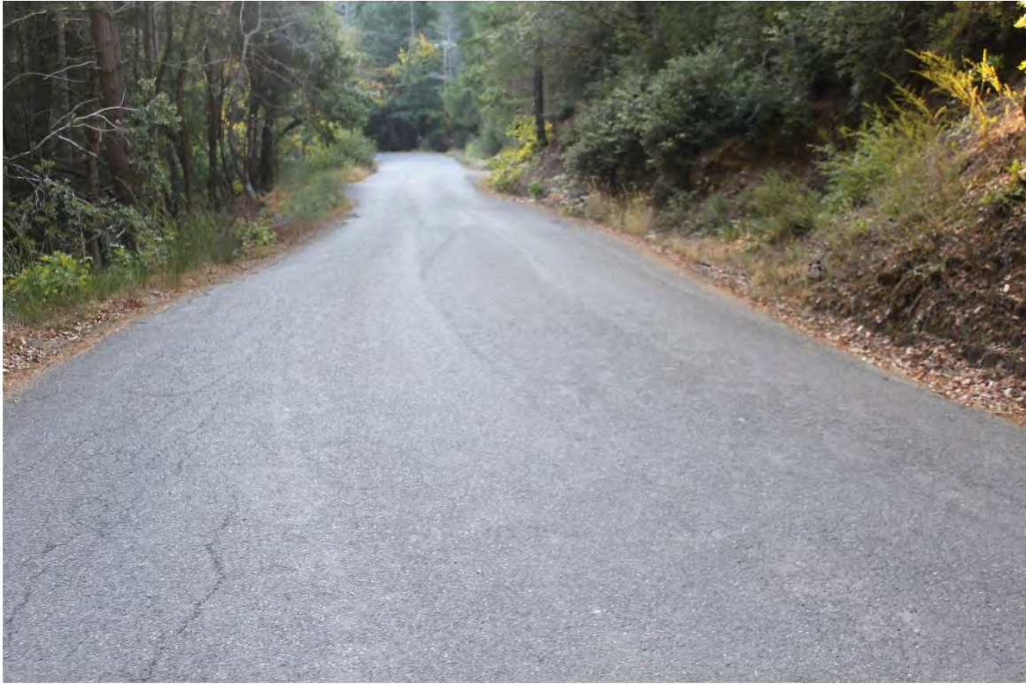
Photo 15. Mile 1.4: 22-ft road width with 1-ft shoulders.
