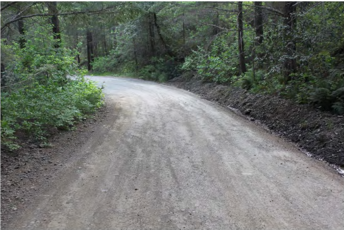
Photo 8. Mile 0.6: 18' width, 1' shoulders.
