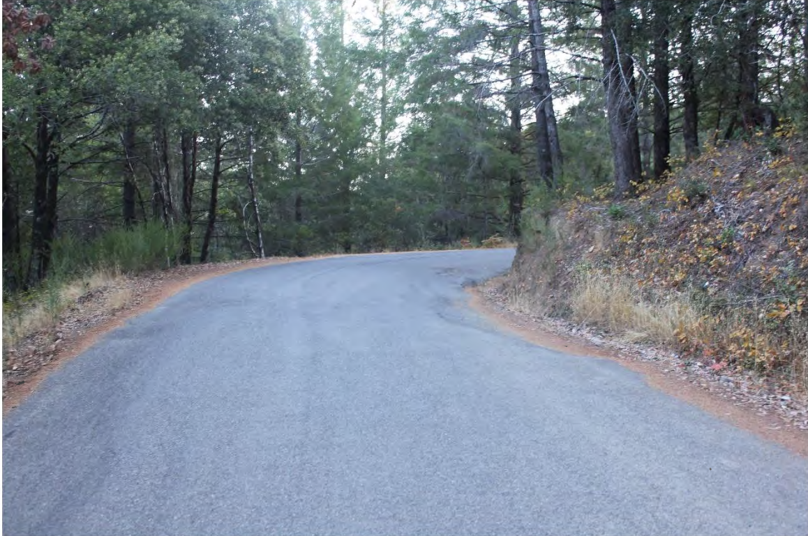
Photo 13. Mile 1.2: 20-ft road width with 1-ft shoulders.
