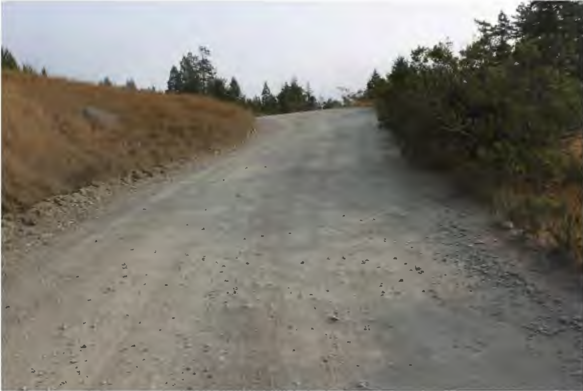
Photo 5. Mile 0.4: 18' width, 1' shoulders.
