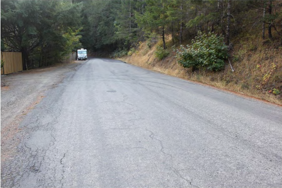
Photo 13. Mile 1.6: 24' width, 2' shoulders.
