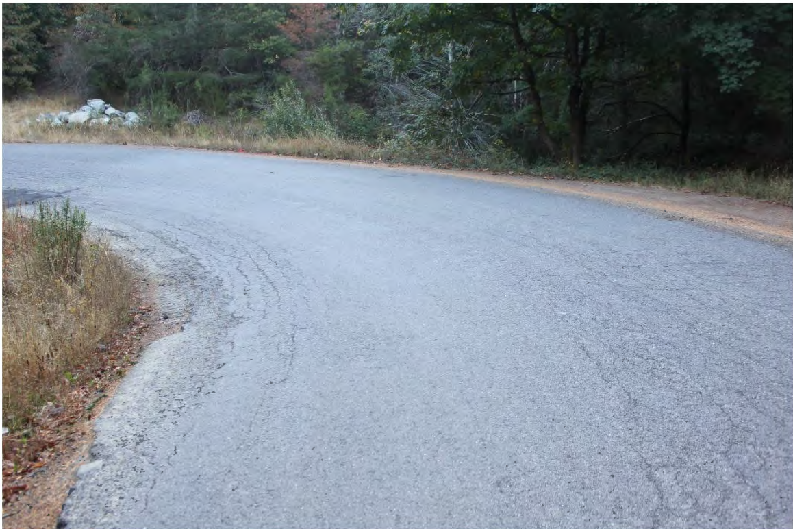
Photo 10. Mile 0.9: 24-ft road width with 2-ft shoulders.
