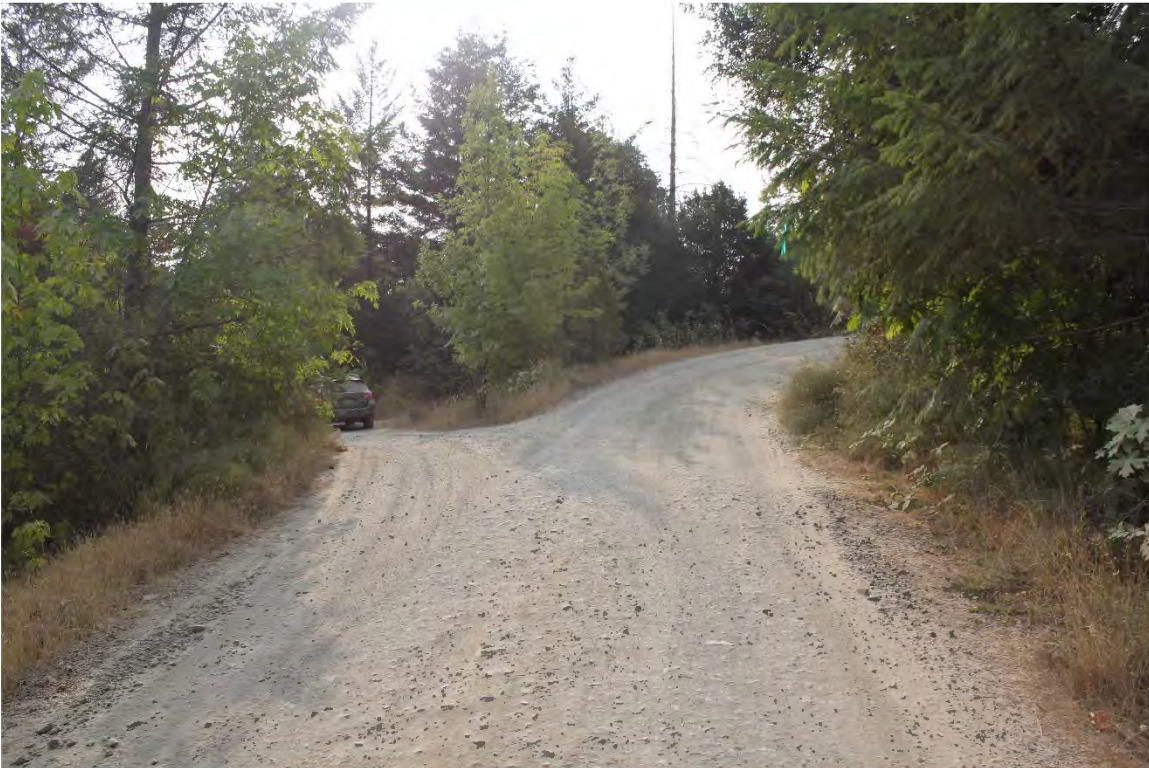
Photo 14. Mile 1.2: 18' width, 1' shoulders; end segment four at major intersection.
