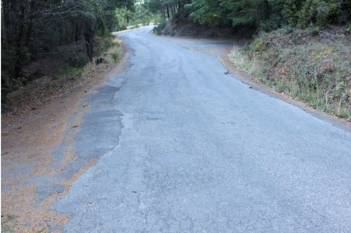
Photo 33. Mile 2.9: 18-ft road width with 1-ft shoulders.
