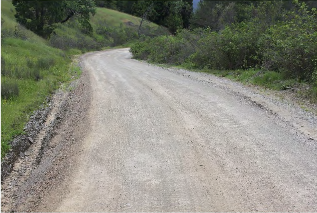
Photo 1. Mile 0.1: 16' width, 1' shoulders; road crosses geologically unstable area with some wider turnouts and brush impairing visibility.
