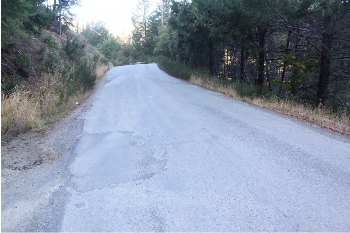
Photo 31. Mile 2.7: 20-ft road width with 2-ft shoulders.
