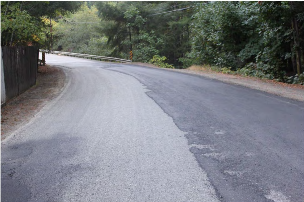
Photo 12. Mile 1.5: 24' width, 2' shoulders.
