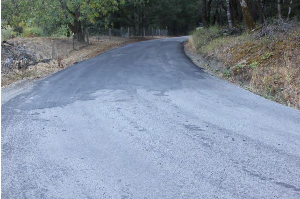
Photo 9. Mile 0.8: 30-ft road width with 1-ft shoulders.
