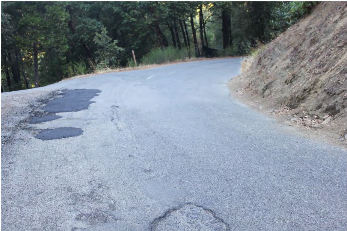
Photo 20. Mile 1.9: 18-ft road width with 2-ft shoulders.
