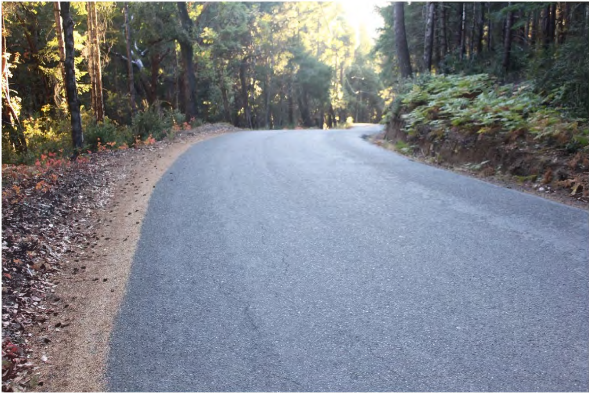
Photo 17. Mile 1.6: 20-ft road width with 2-ft shoulders.
