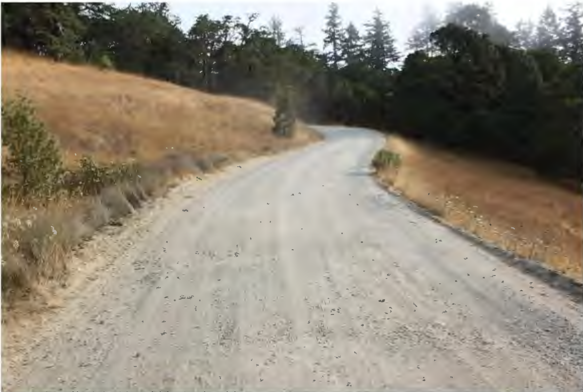
Photo 2. Mile 0.2: 18' width, 1' shoulders.
