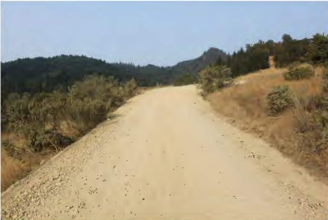
Photo 8. Mile 0.7: 18' width, 1' shoulders.
