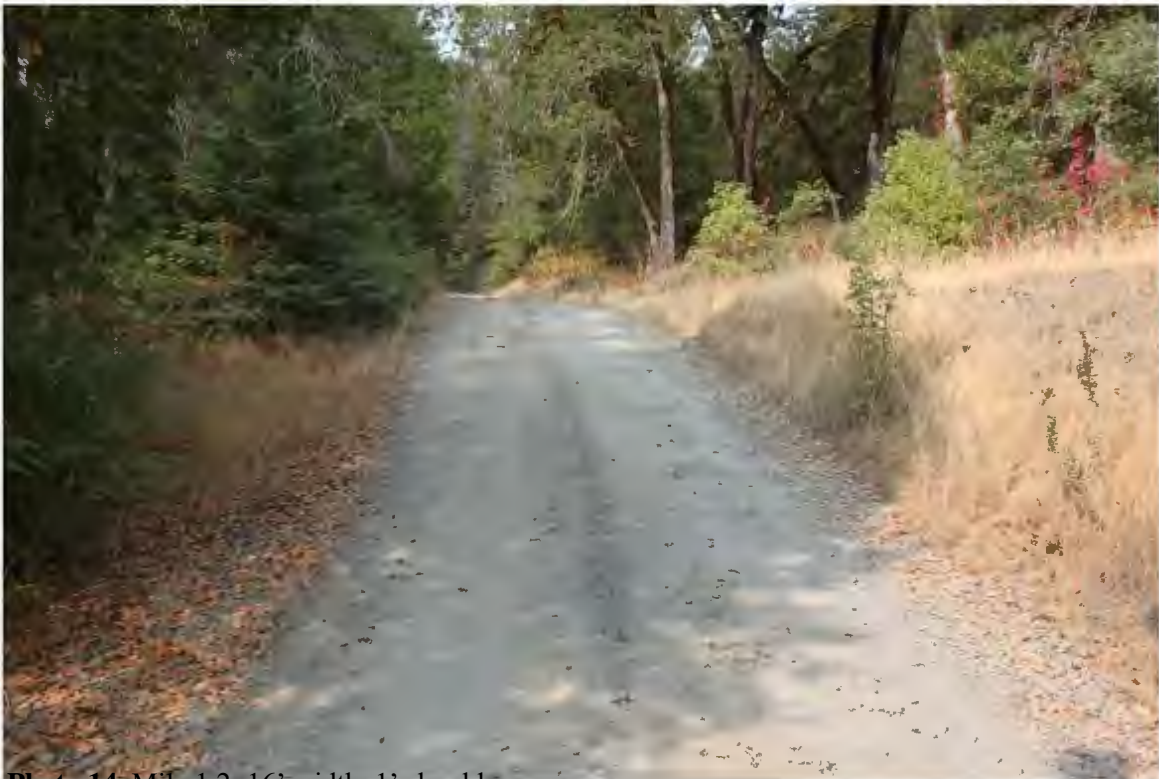
Photo 14. Mile 1.2: 16' width, 1' shoulders.
