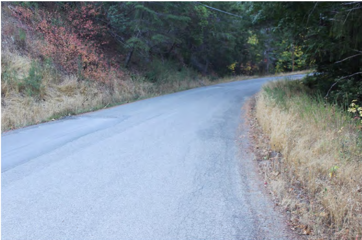
Photo 14. Mile 1.3: 22-ft road width with 2-ft shoulders.
