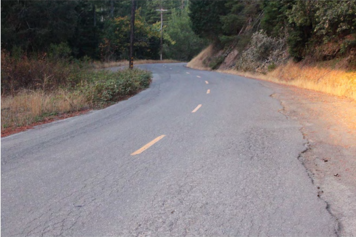
Photo 1. Mile 0.1 Category 4 segment with yellow stripe, typical of segment from 0.0 to 0.7.
