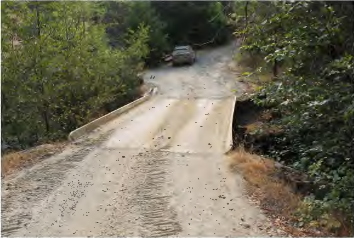
Photo 15. Mile 1.22: 12' width bridge with turnouts on both sides and good visibility.
