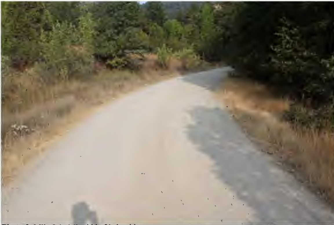
Photo 2. Mile 0.1: 16' width, 2' shoulders.
