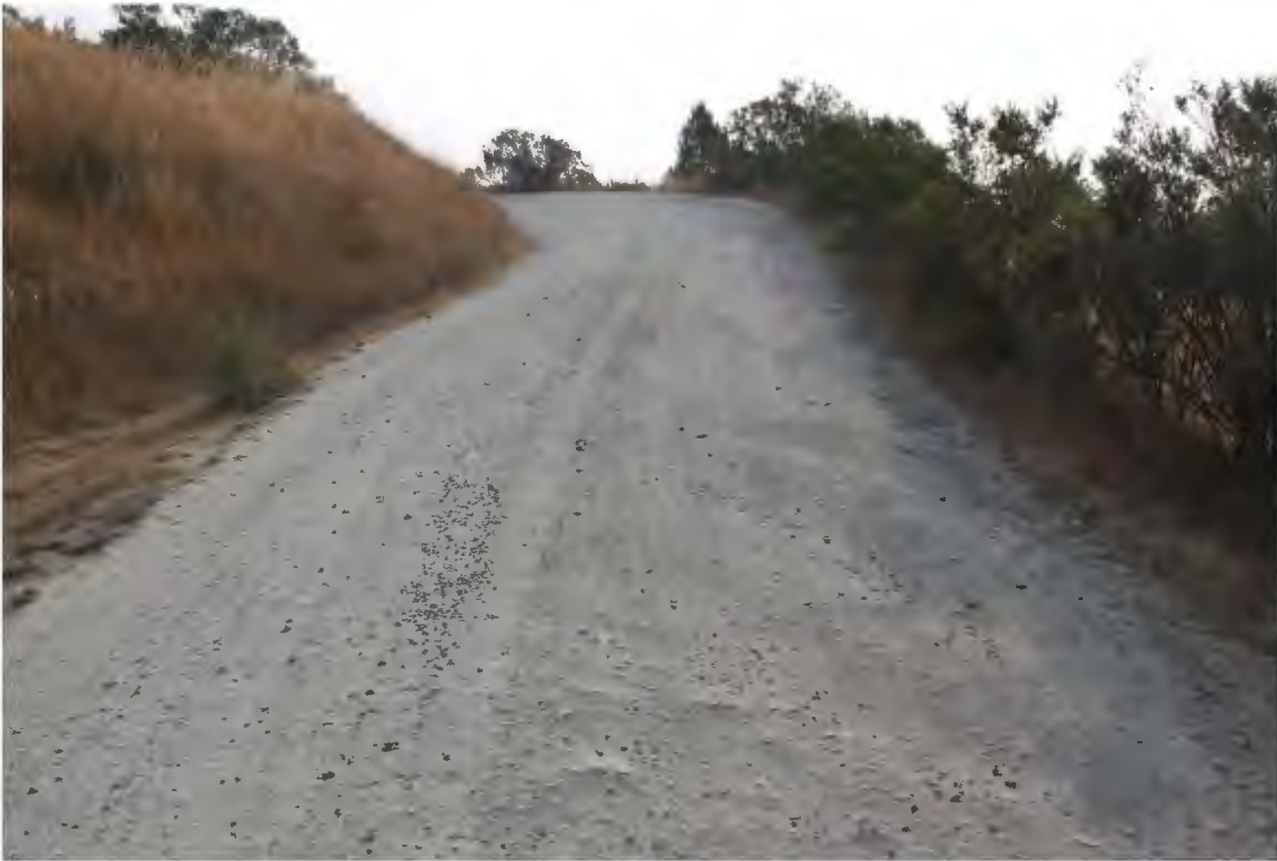
Photo 7. Mile 0.6: 18' width, 2' shoulders.
