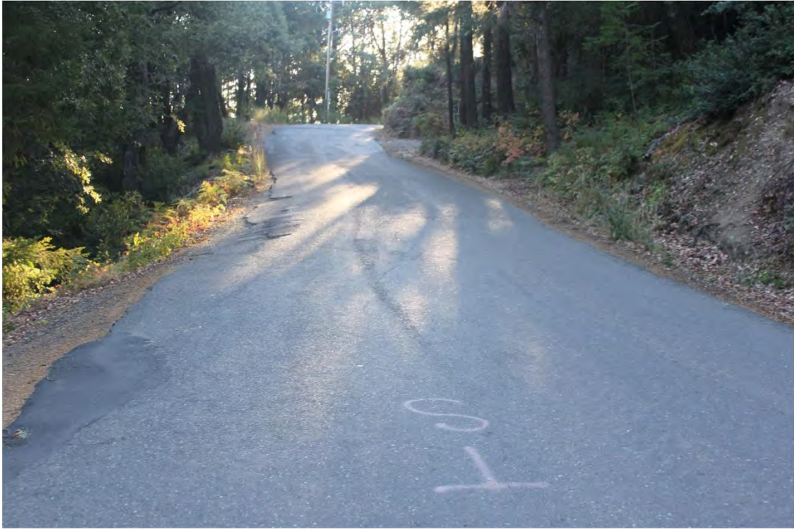
Photo 19. Mile 1.8: 20-ft road width with 2-ft shoulders.
