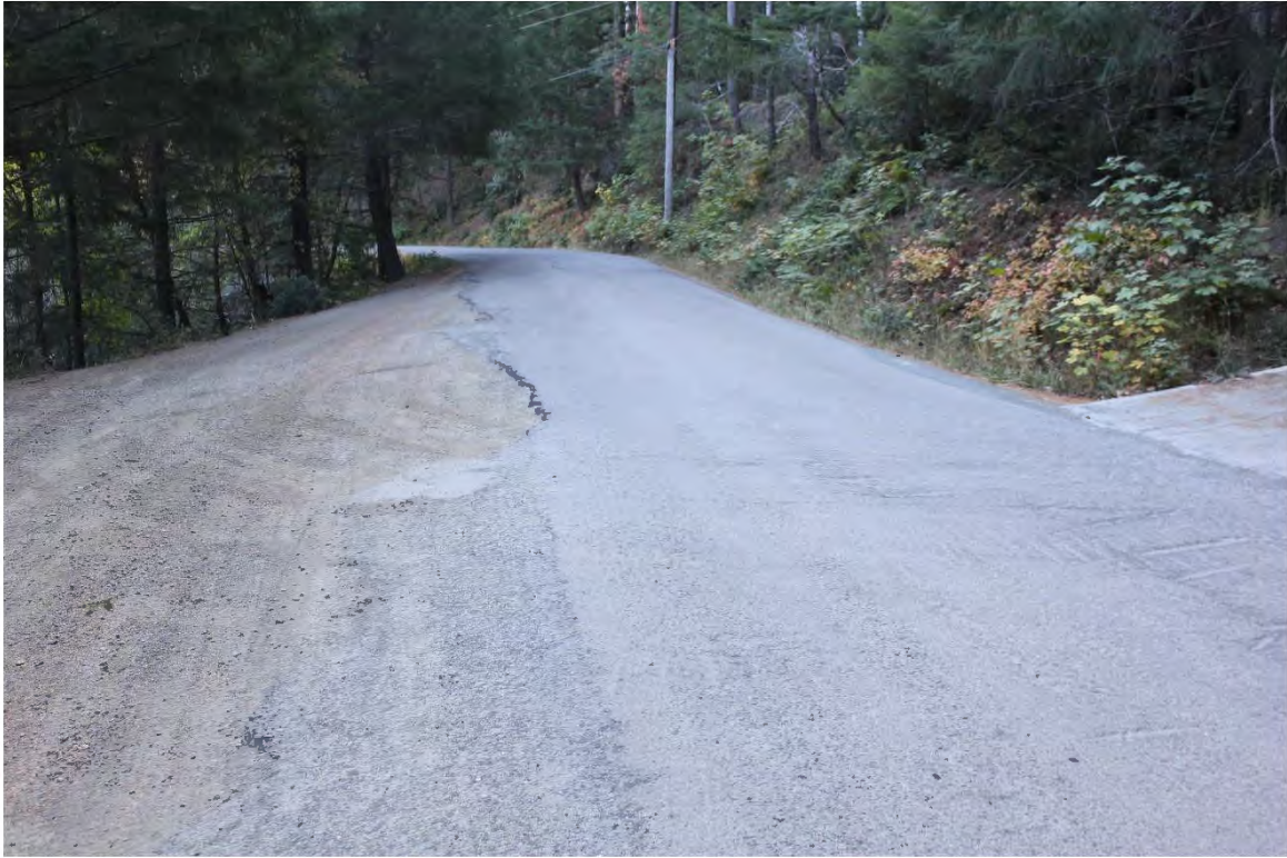
Photo 25. Mile 2.3: 20-ft road width with 2-ft shoulders.
