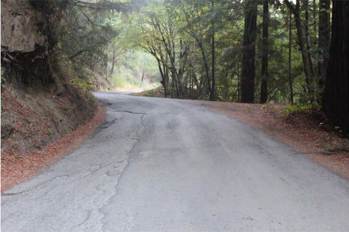
Photo 9. Mile 1.3: 16' width, 1' shoulders pinch point, OK visibility.
