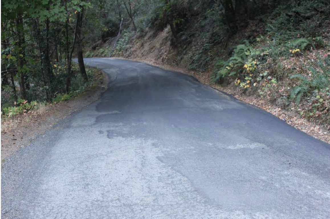
Photo 3. Mile 0.3: 18-ft road width with 1-ft shoulders.
