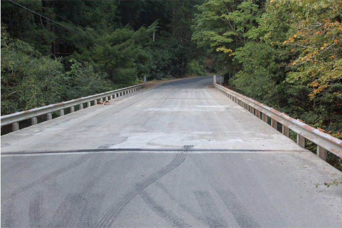
Photo 11. Mile 1.45: 28' width bridge, no shoulders.
