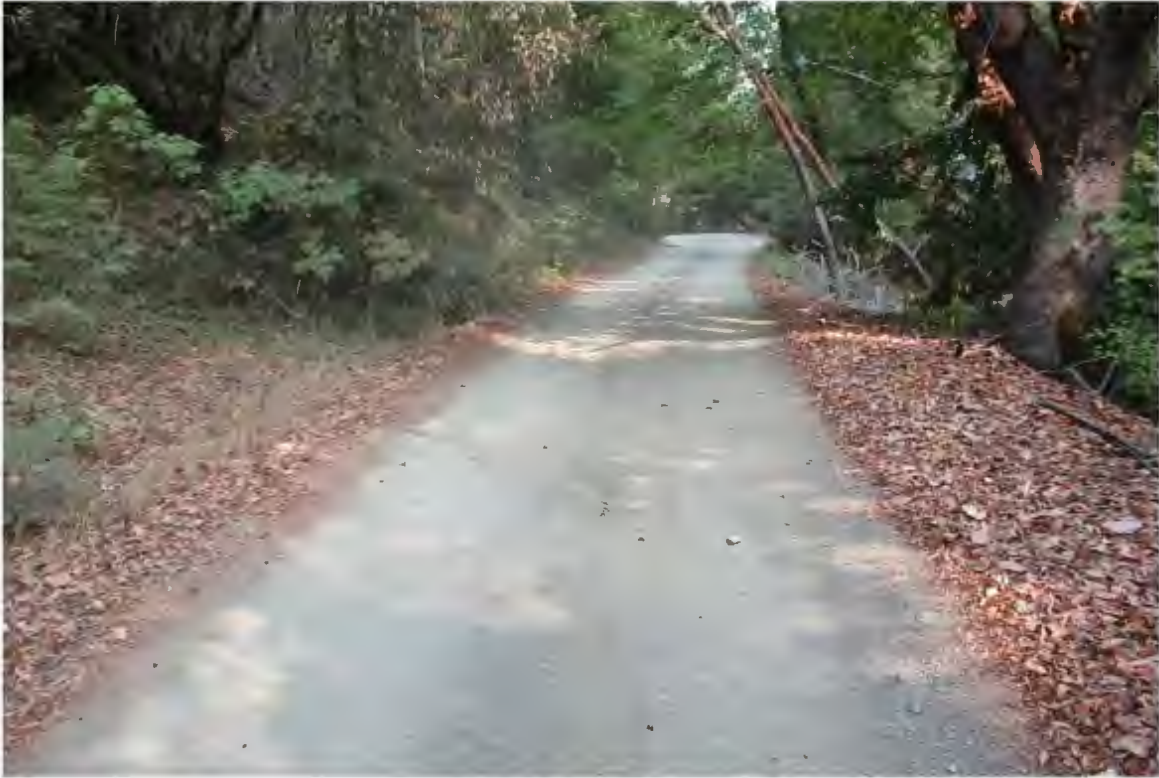
Photo 9. Mile 0.7: 14' width, 2' shoulders, with vegetation encroachment into roadway.
