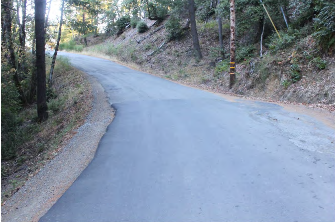
Photo 29. Mile 2.5: 18-ft road width with 2-ft shoulders.
