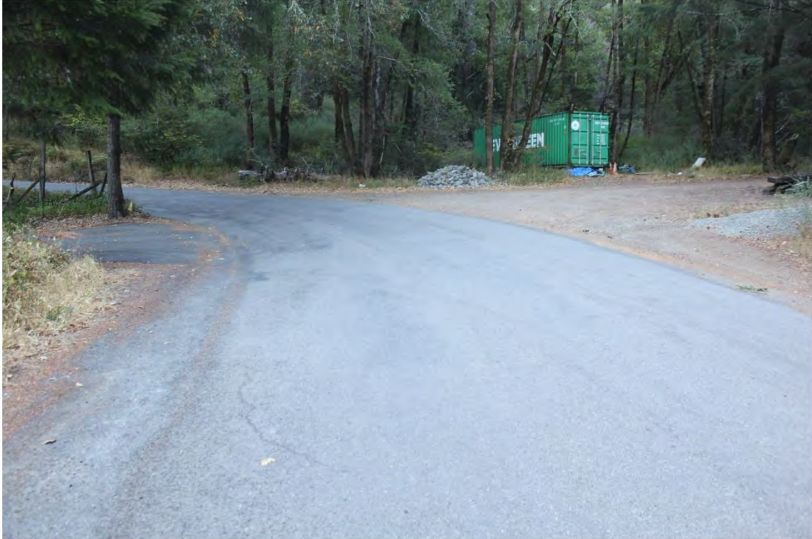
Photo 7. Mile 0.6: 24-ft road width with 2-ft shoulders.
