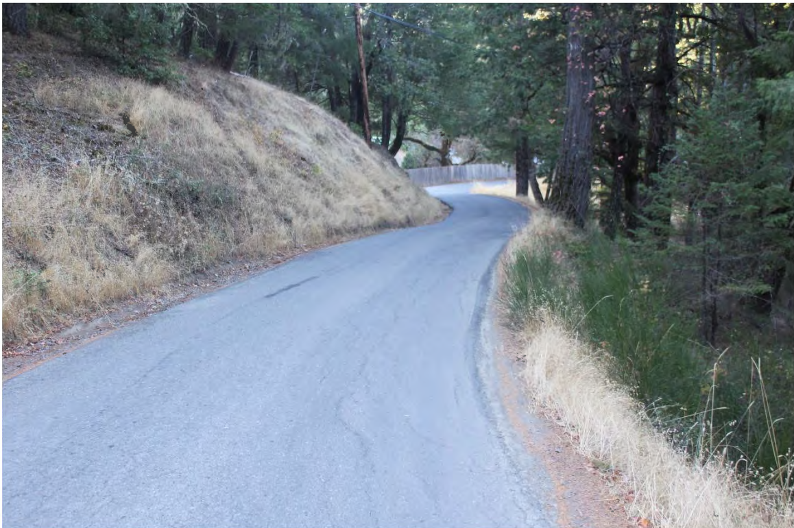
Photo 34. Mile 3.0: 15-ft road width with 1-ft shoulders.
