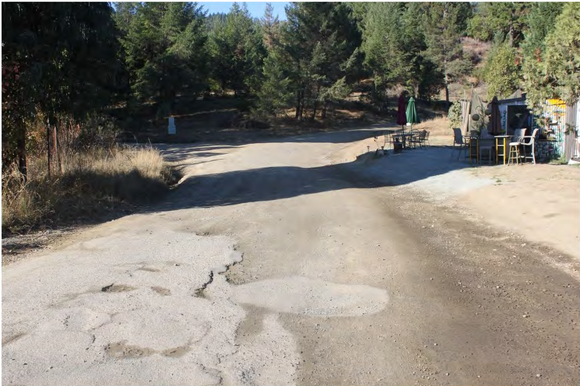
Photo 48. Mile 4.1: 20-ft road width with 2-ft shoulders. Intersection with Upper Thomas Road and end of County-maintained road. End of Segment 2.
