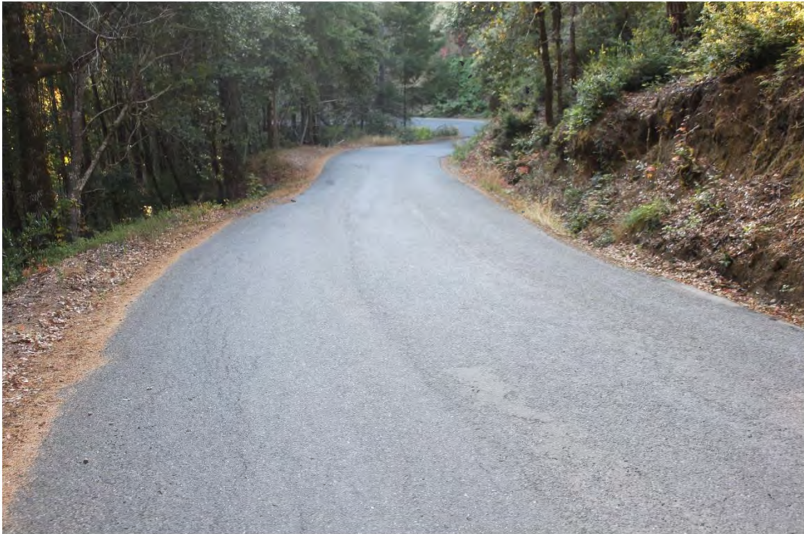
Photo 16. Mile 1.5: 20-ft road width with 1-ft shoulders.
