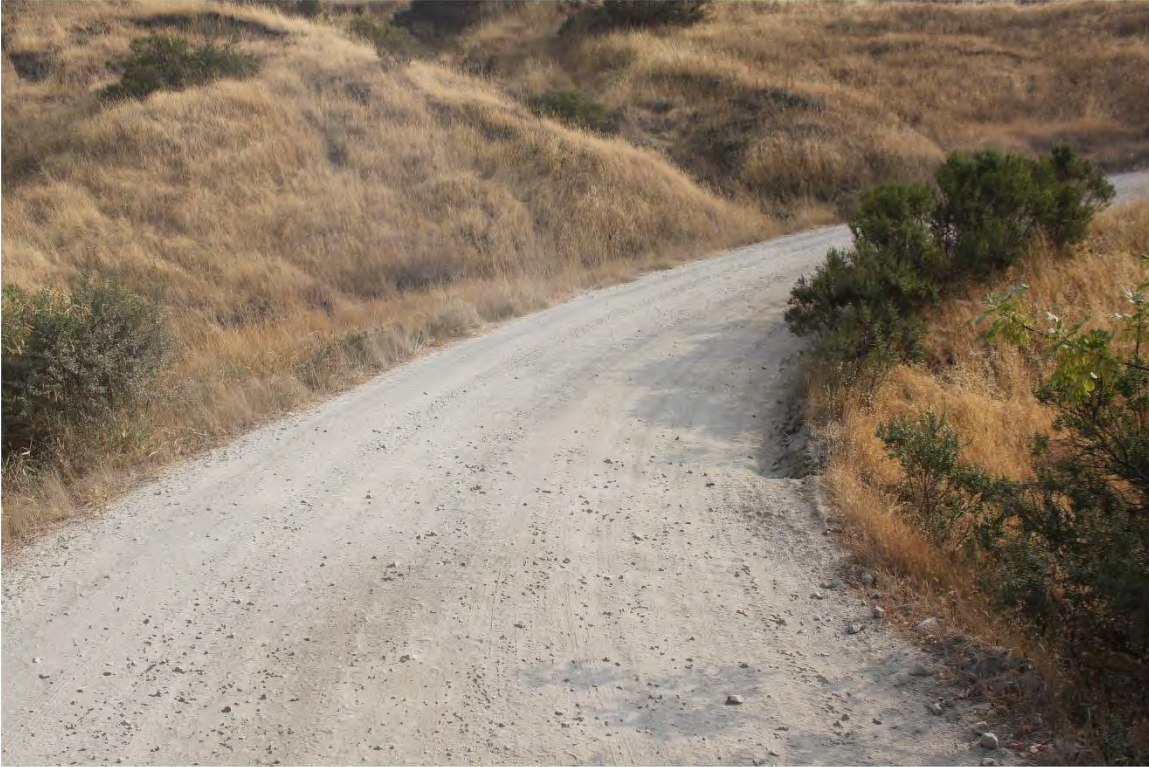
Photo 11. Mile 0.9: 18' no shoulders, good visibility at deep culvert crossing.
