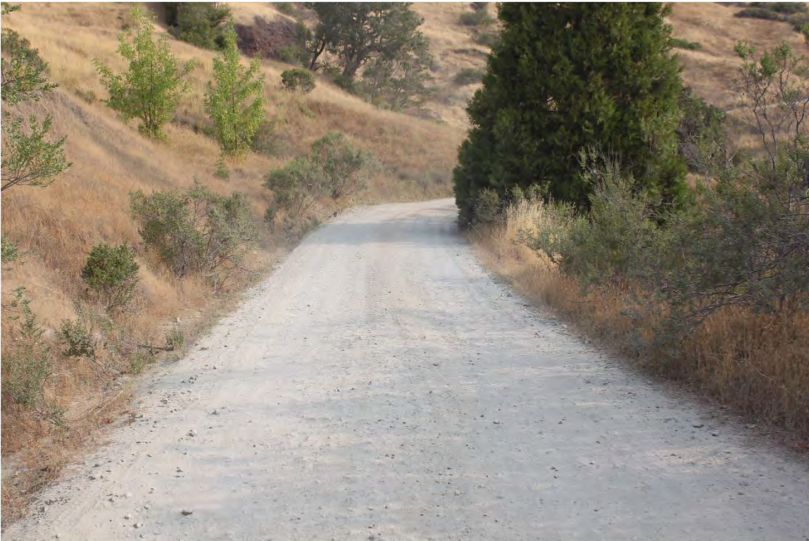
Photo 12. Mile 1.0: 15' width, 1' shoulders, generally ok visibility.
