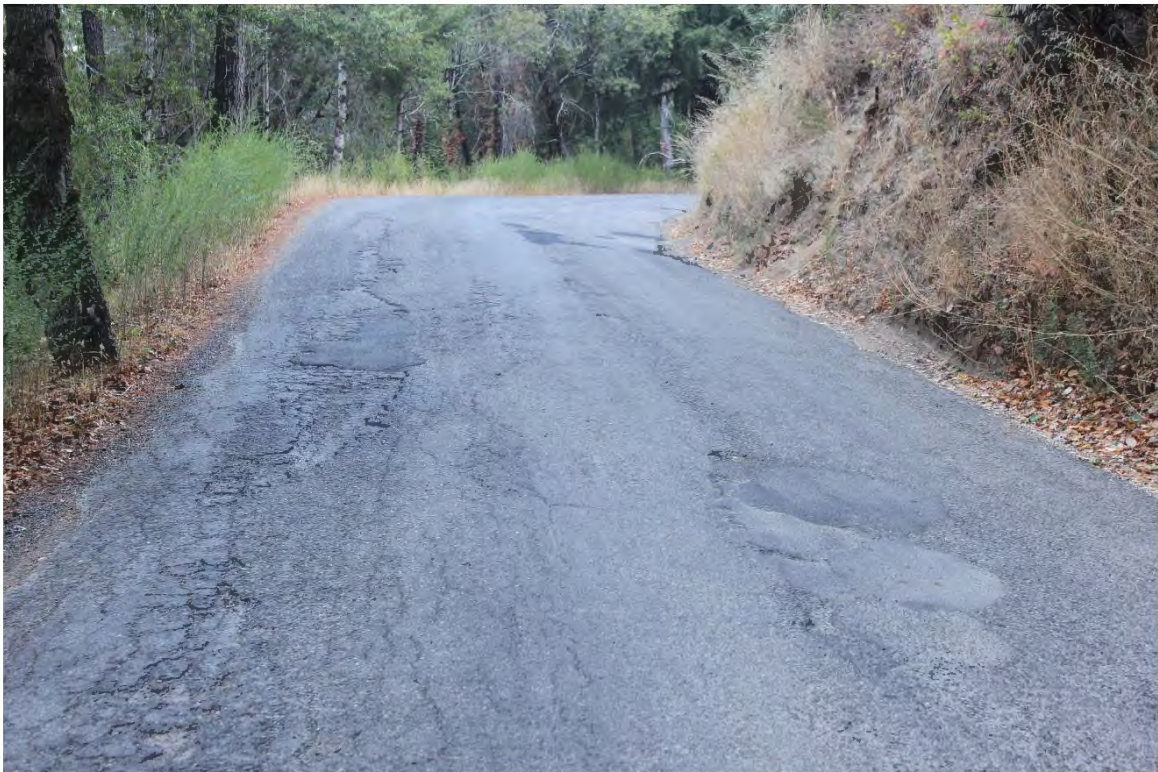
Photo 6. Mile 0.5: 18-ft road width with 1-ft shoulders.
