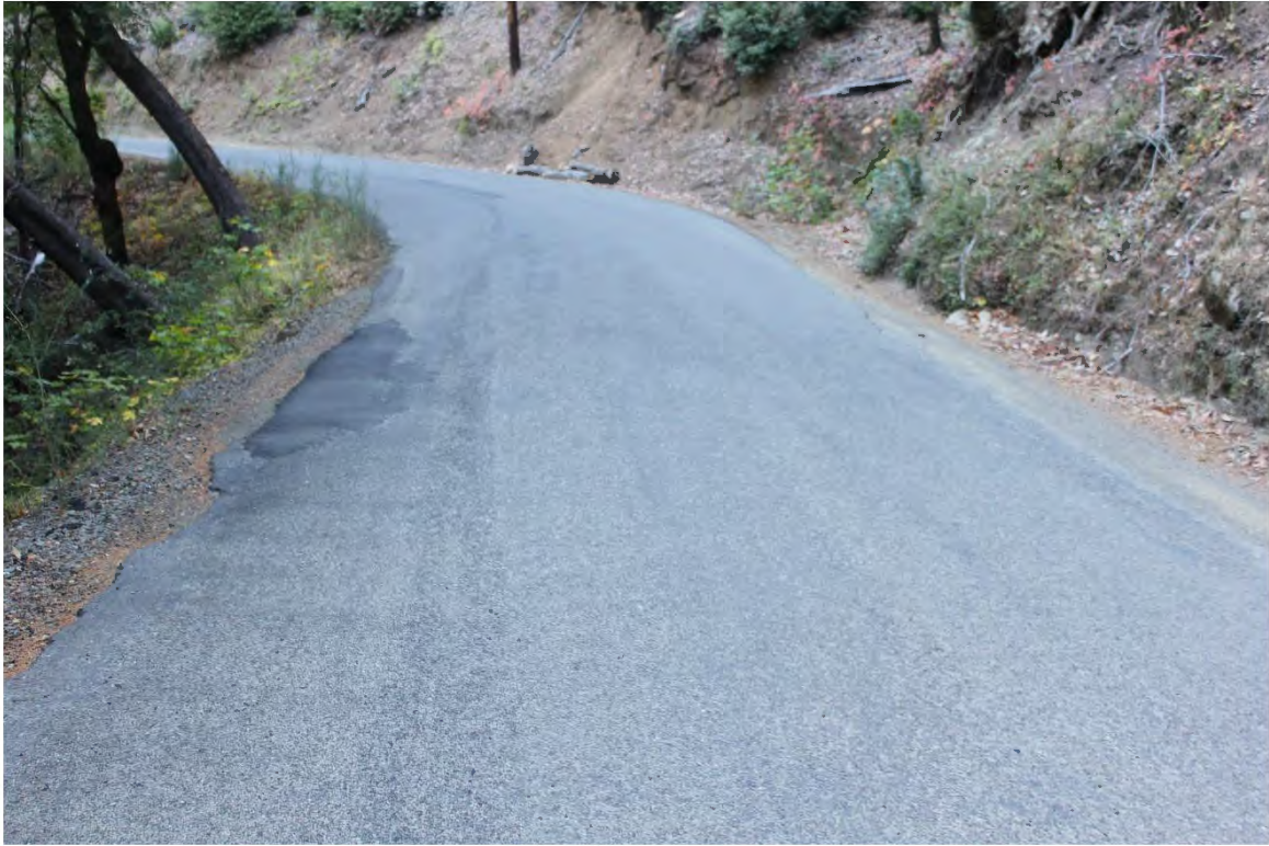
Photo 21. Mile 2.0: 15-ft road width with 1-ft shoulders.
