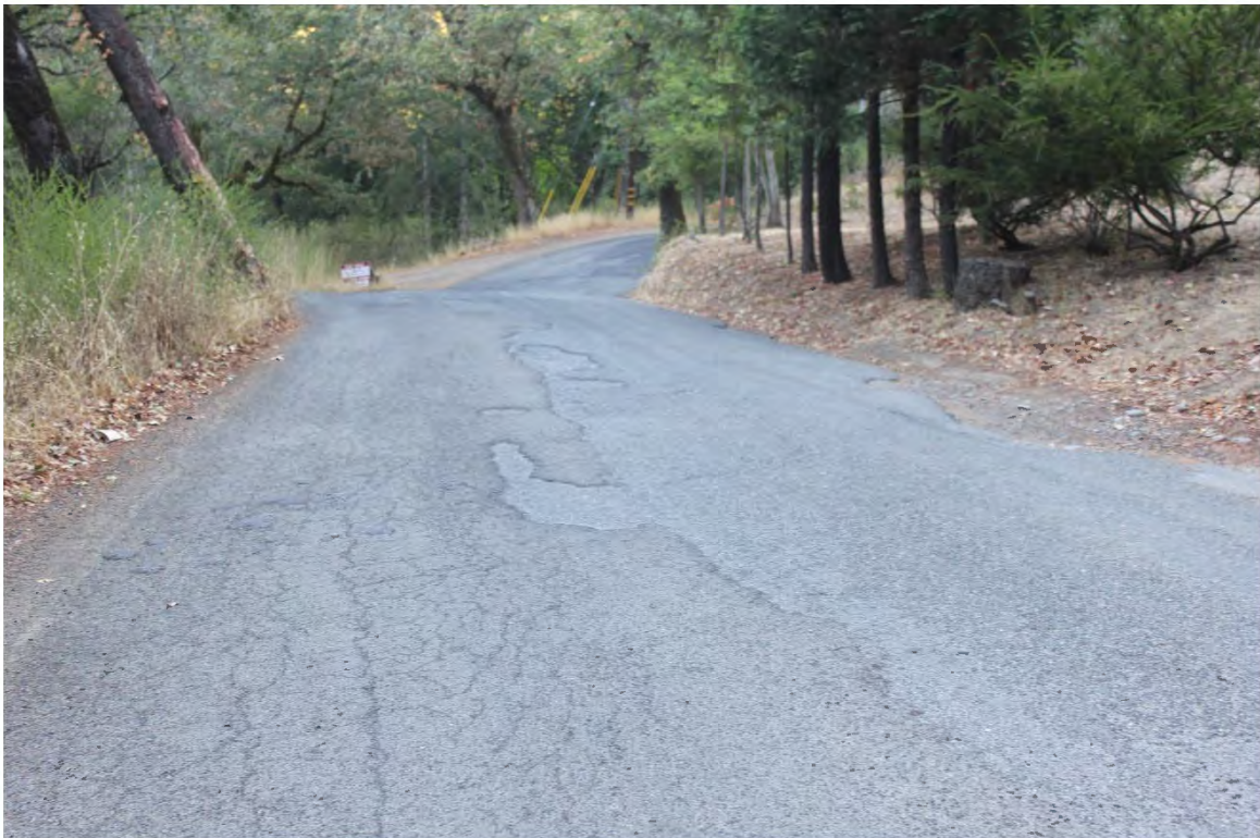
Photo 4. Mile 0.4: 18-ft road width with 1-ft shoulders.
