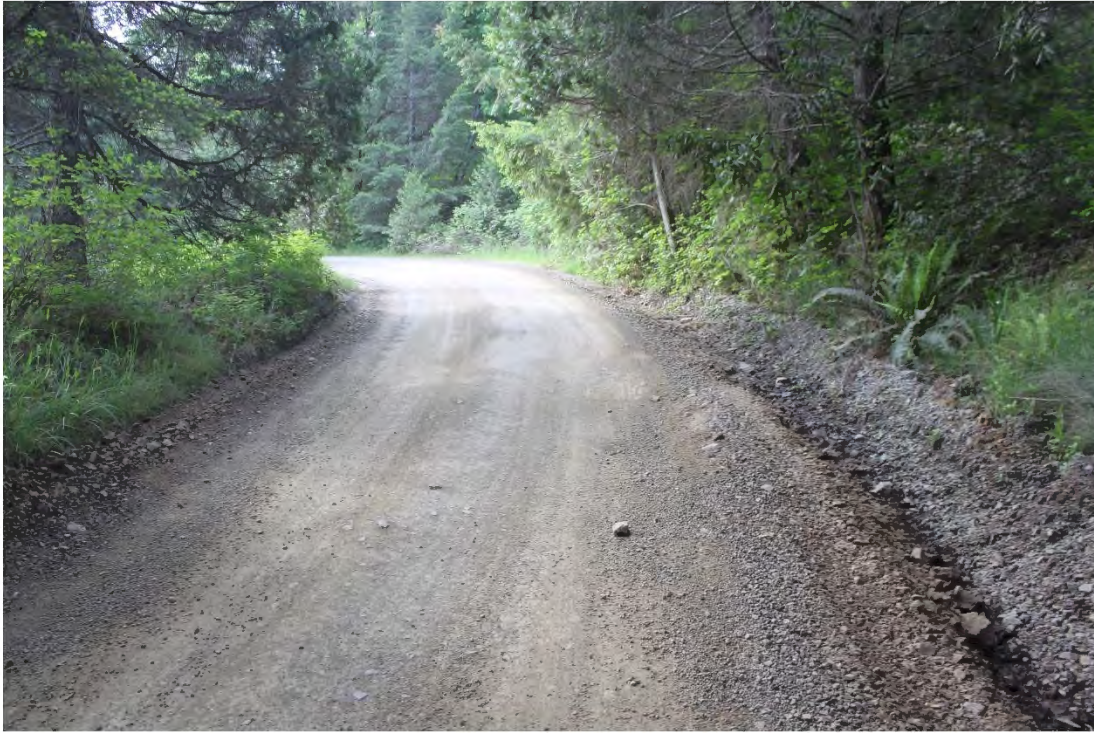
Photo 9. Mile 0.65: ~16' width pinch point with deep ditch.
