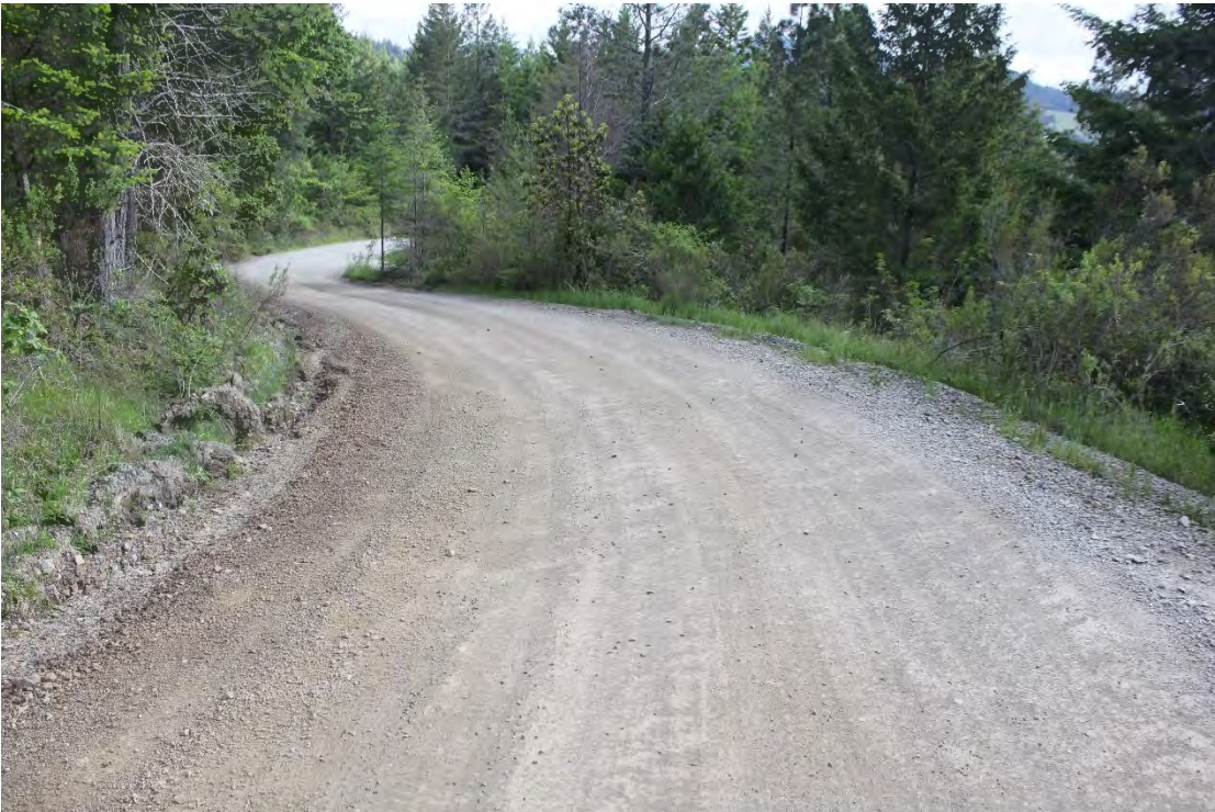
Photo 6. Mile 0.4: 18' width, 1' shoulders.
