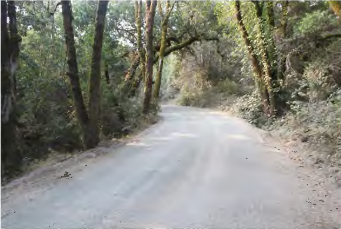
Photo 3. Mile 0.25: 15' pinchpoint at culvert crossing.
