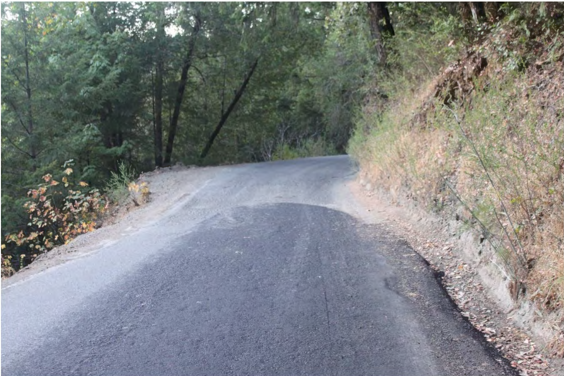
Photo 4. Mile 0.9: relatively narrow section, 15' width, 1' shoulders.
