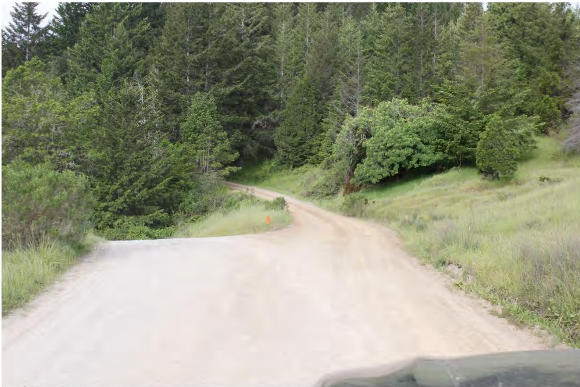
Photo 12. Mile 0.85: End Segment 3 at driveway.
