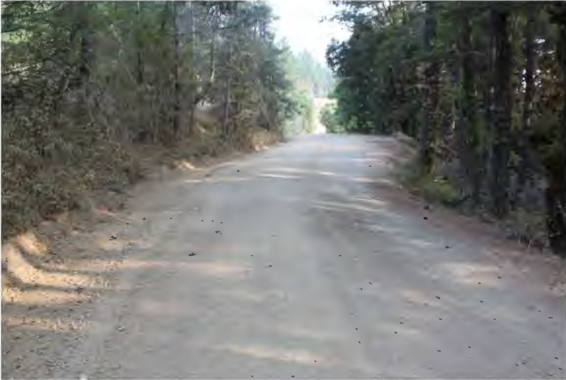
Photo 1. Mile 0.1: 18' width 1' shoulders.
