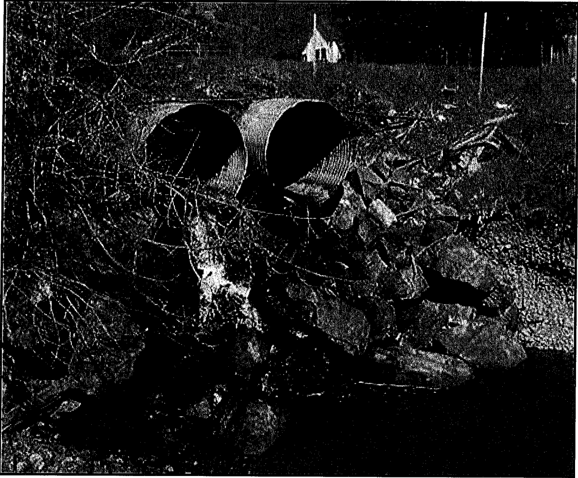
Figure 3. Rock armoring on shotgun culvert outlet. Photo Courtesy of California Department of Transportation (Caltrans).
