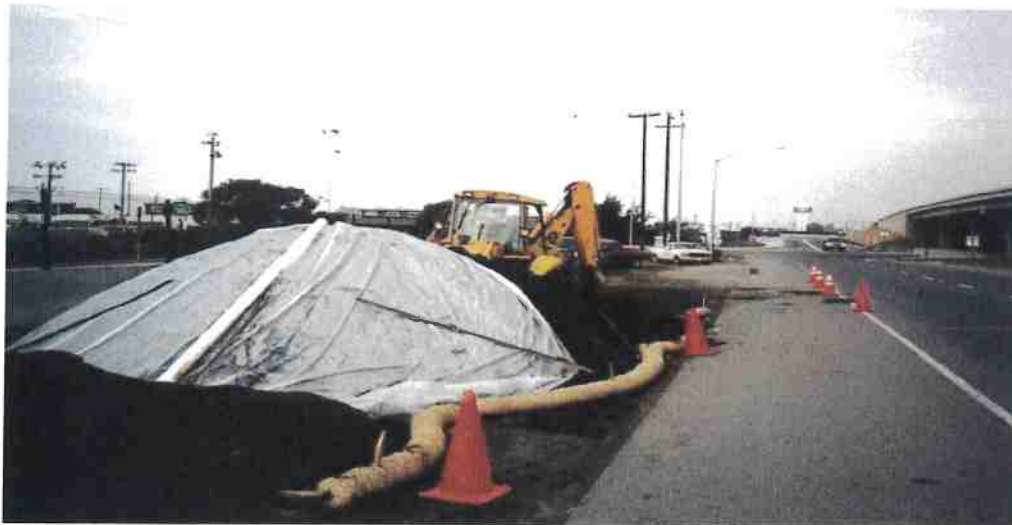
Figure 1. Stock piles should be covered with erosion and sediment control BMPs employed to keep sediment on site. From Caltrans (2003).
