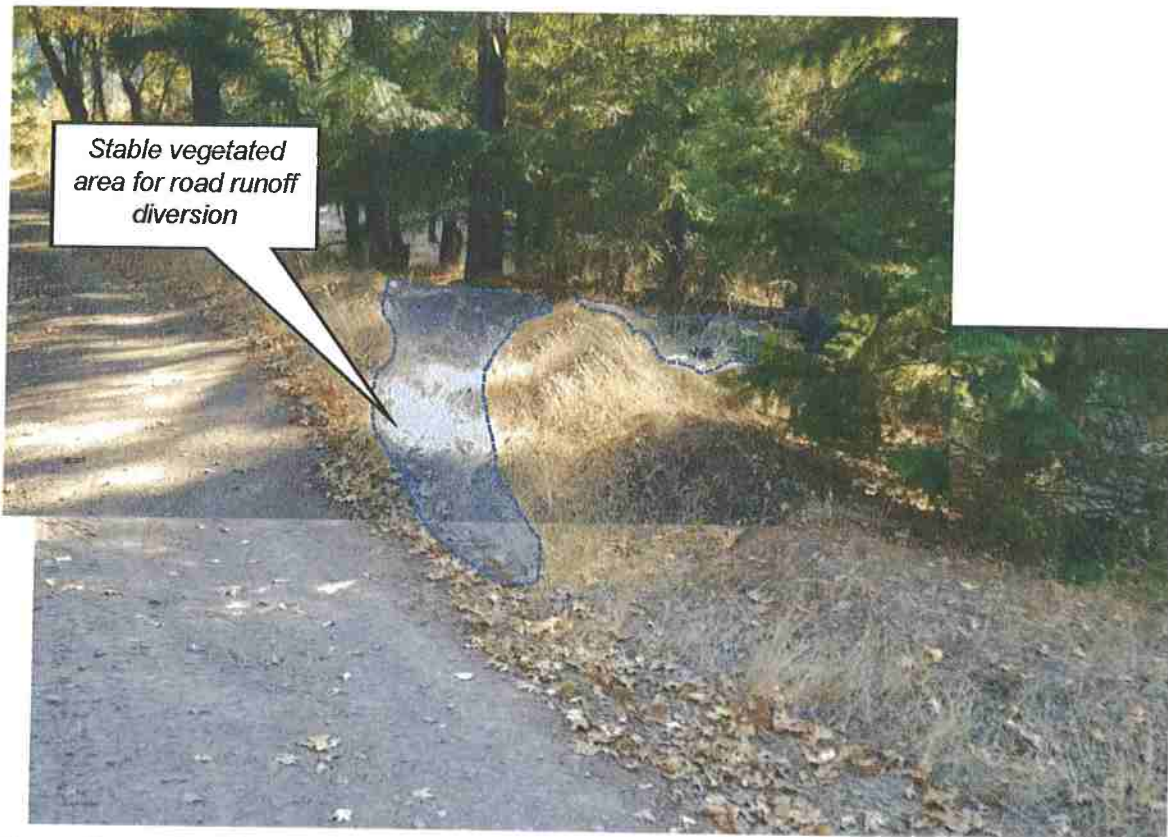
Figure 2. Interim Measure A – Installation of a 20', 9" diameter straw wattle at the top of the steep road segment (right) to direct runoff from the upper road (behind photographer in these photos) into a stable vegetated area (top), and prevent additional erosion problems.
