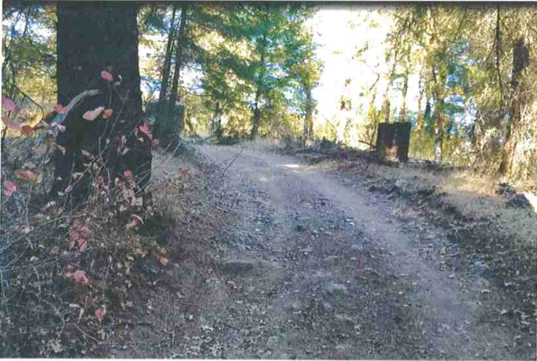
Figure 3. Interim Measure B – View of the steep (19% grade) road segment east of the culverts. Use of the road will be discontinued pending assessment for potential restoration or other measures to eliminate erosion.
