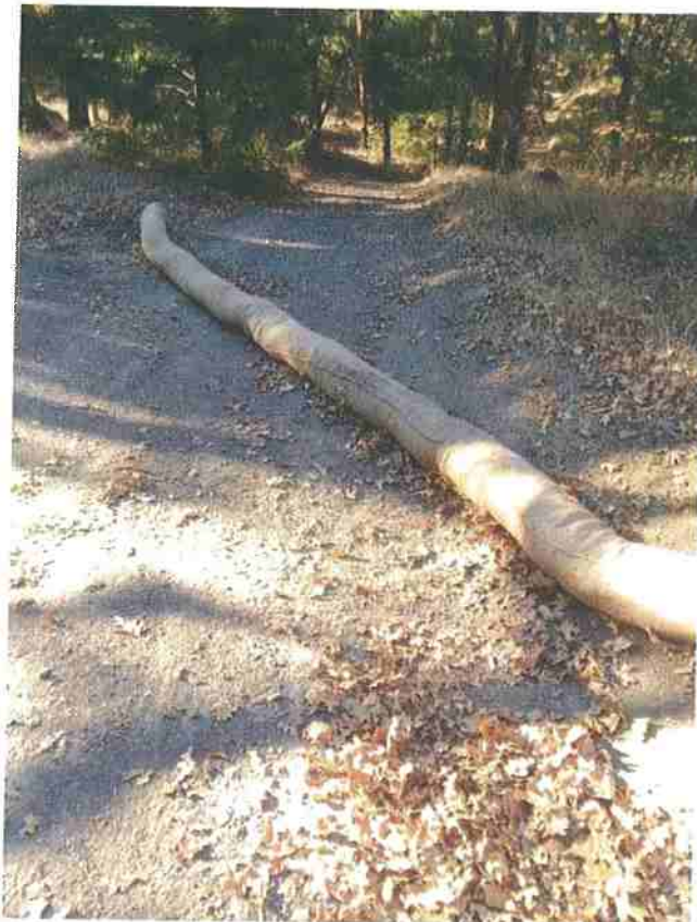
Figure 2. Interim Measure A – Installation of a 20', 9" diameter straw wattle at the top of the steep road segment (right) to direct runoff from the upper road (behind photographer in these photos) into a stable vegetated area (top), and prevent additional erosion problems.
