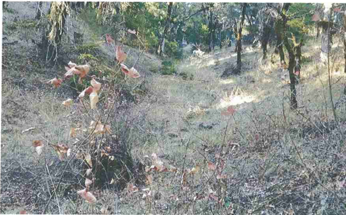
Figure 4. Interim Measure C – View of watershed above eastern culvert. The combined watershed for both eastern and western culverts is 7.25 acres. The eastern portion of the watershed is less than 5 acres, with an estimated 100-year peak flow rate of less than 5 cfs, and 5-year rate of less than 3 cfs.
