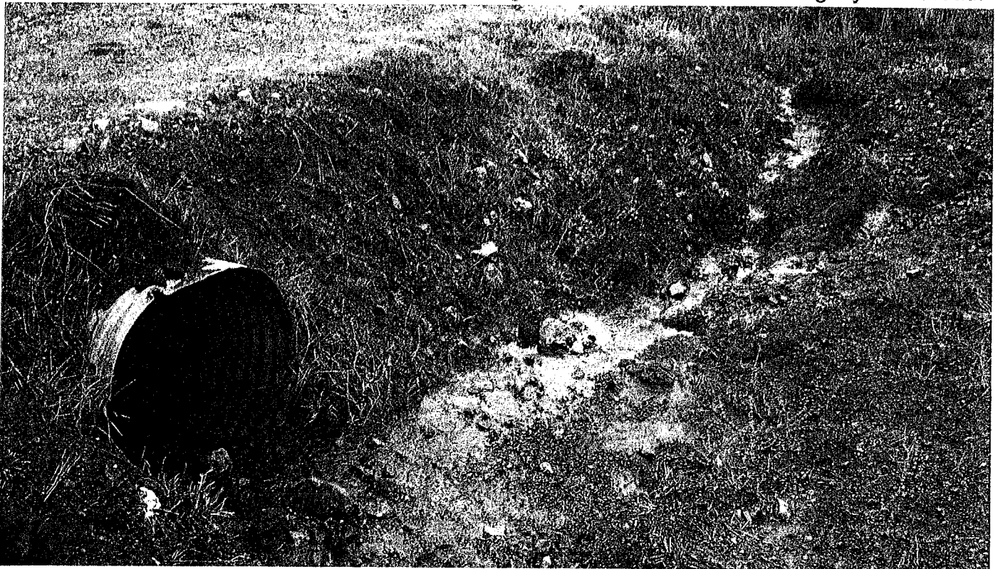
Site 11 – Class III watercourse crossing consisting of a 36" culvert. This culvert is misaligned and too short however is functioning adequately and sized appropriately.
