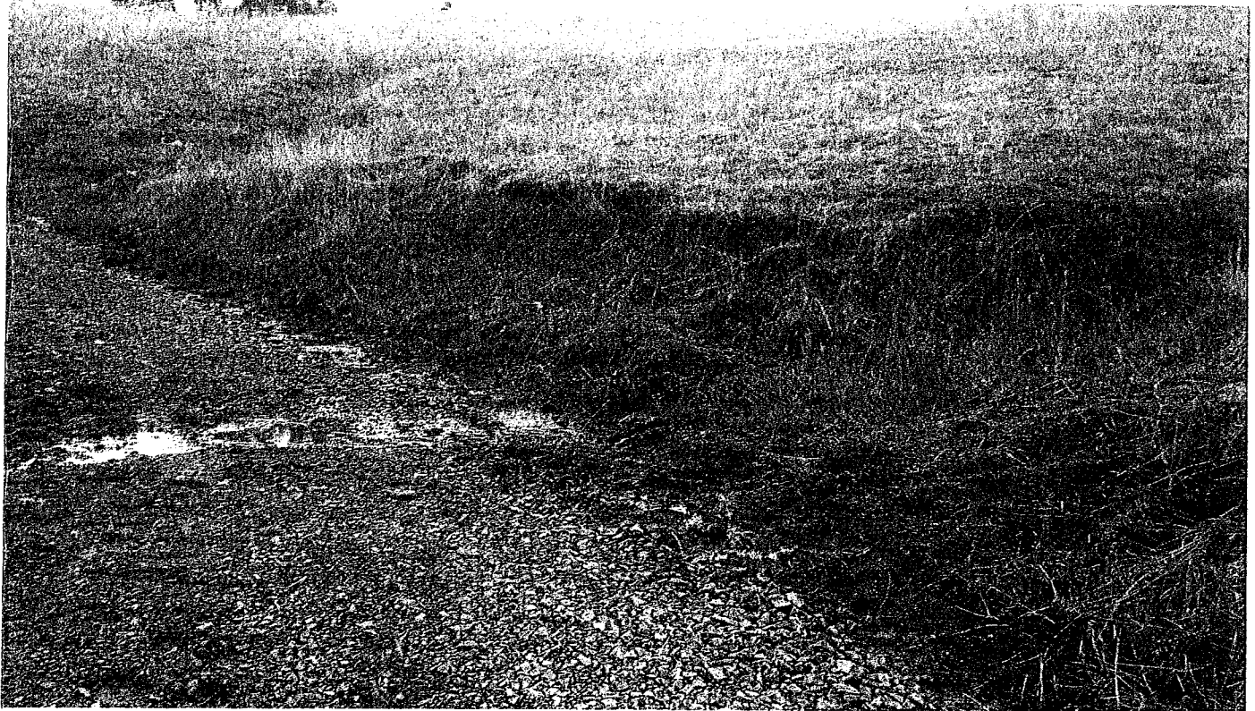
Site 13 – Class III watercourse crossing consisting of a rock ford. It has been recommended to install additional rock consisting of 3-6" minus on the 15 feet of inside ditch.
