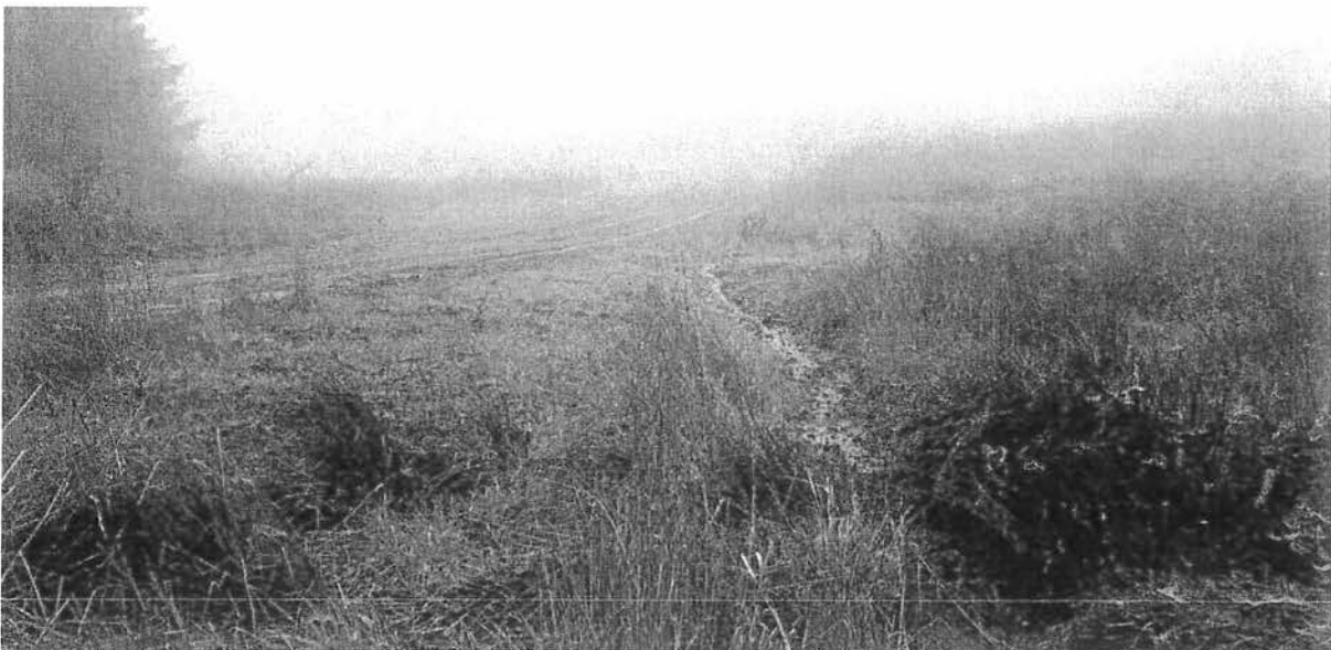
Photo looking north at Site 11, taken from Site 12. The culvert proposed to be installed here will outlet into the ditch shown in the photograph. This culvert installation is being requested by CDFW and North Coast Regional Water Quality Board personnel, to "re-align" a upland swale and wetland area that is being drained by an inside ditch along the left side of the road.
