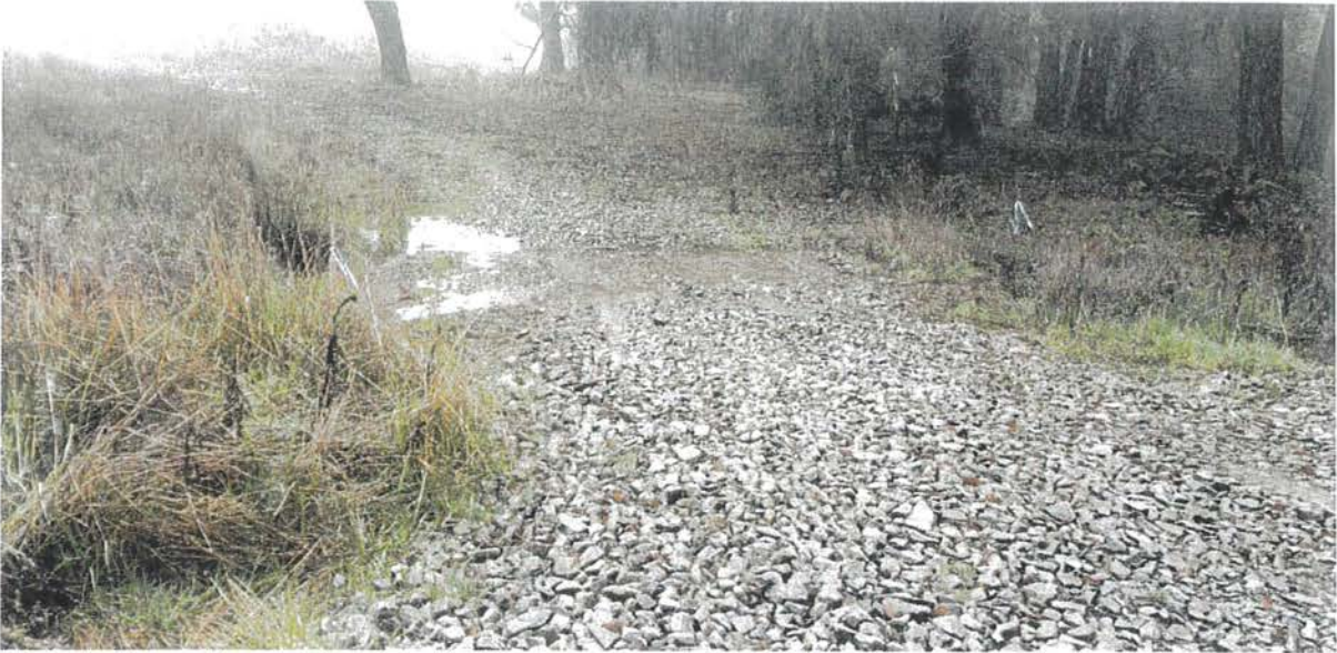
Photo looking southeast at the rocky ford watercourse crossing at Site 12. An 18" D x 20' culvert is being proposed as an upgrade to this crossing, per request by CDFW and North Coast Regional Water Quality Board personnel.
