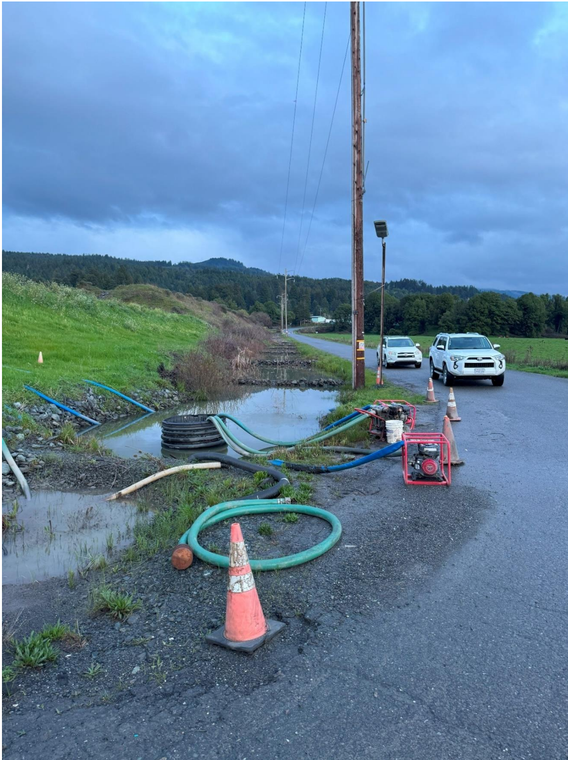
Picture 13 – View of three diesel generators and their pumps observed without required secondary containments. Stormwater is pumped from the swale via the black riser pipe into the newly constructed retention pond. Picture taken by Walt Dragaloski.
