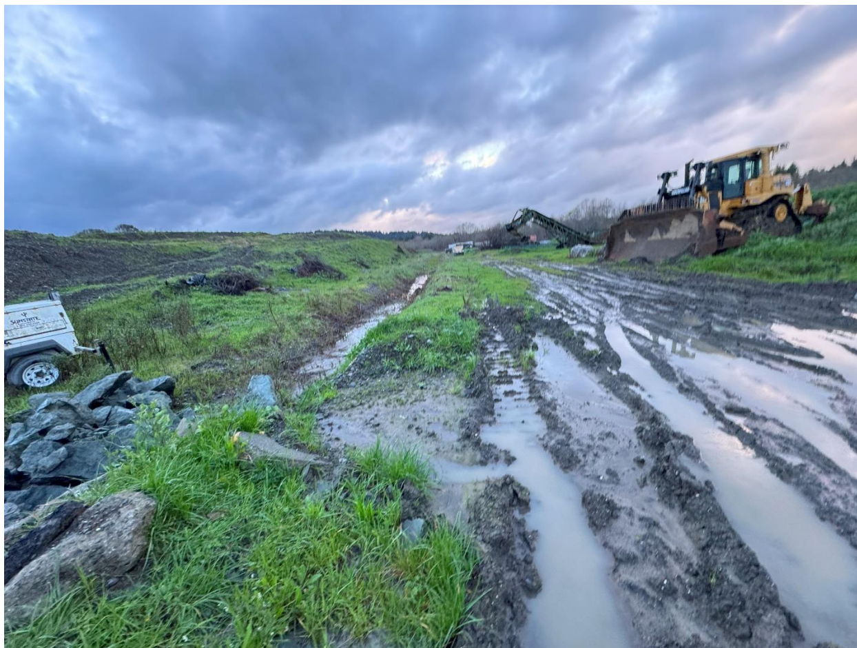
Picture 9 - View of unpaved access road adjacent to an on-site drainage ditch in the lower yard. No sediment and/or erosion control BMPs were observed. Overflow from this ditch discharges into Waters of the State into Noisy Creek or into Waters of the State at an unnamed tributary to Hall Creek. Picture taken by Walt Dragaloski.
