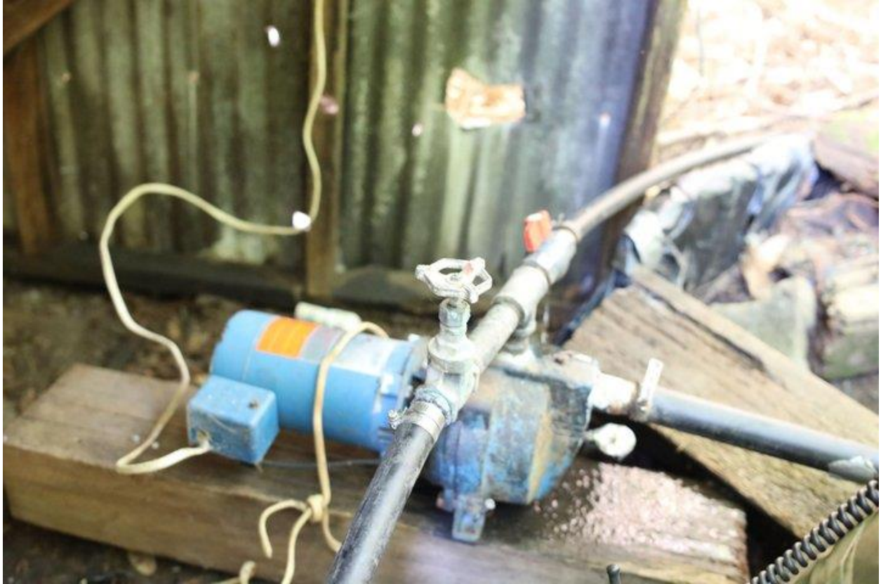
Water pump diverting water from a creek.
