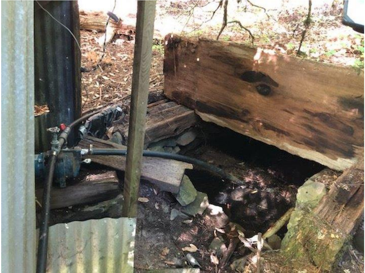
Active water diversion with pump.
