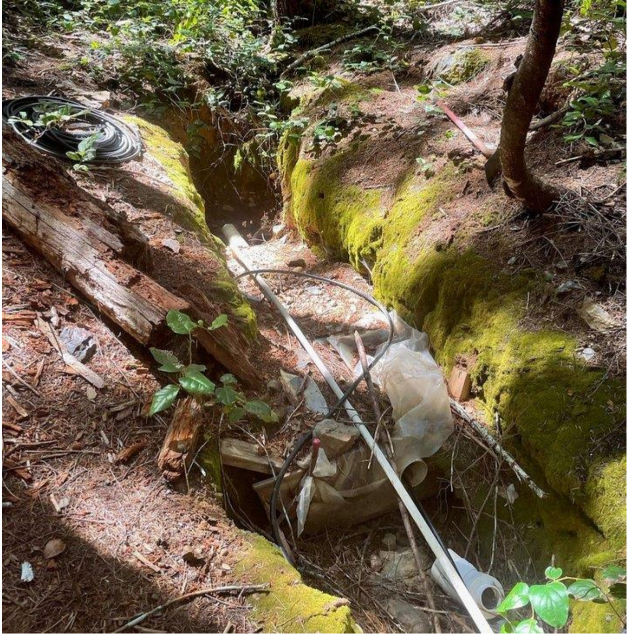
Significant water diversion causing a creek to run dry.
