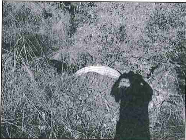
Photo #63 River Rd Looking @ 36" Culvert Out (Dual?)
