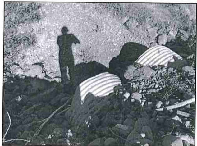
Photo #16 River Rd Looking @ Dual 36" Culverts Out
