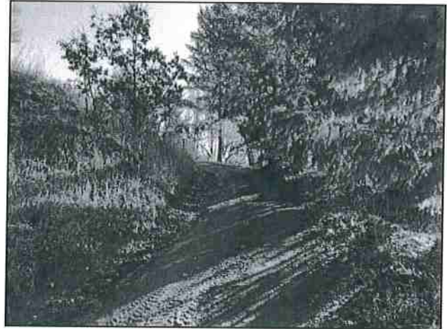
Photo #14 APN 208-241-019 Private Access Rd Looking SE @ Drainage Issue
