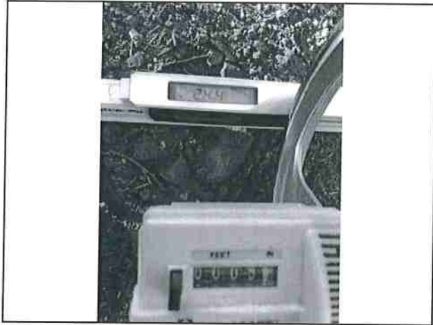
Photo #13 APN 208-241-019 Private Access Rd Width 9'4" Slope 24.4%
