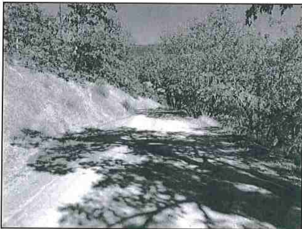
Photo #47 River Rd Looking East @ Turnout
