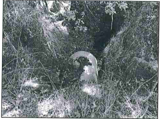
Photo #62 River Rd Looking @ 36" Culvert Out (Dual?)
