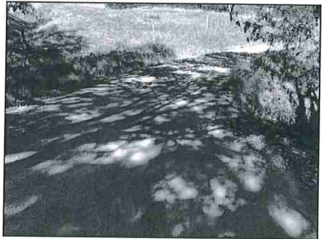
Photo #70 River Rd @ Turnout Looking @ Curve
