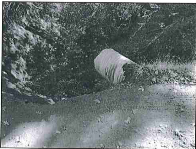
Photo #89 River Rd Looking @ 24" Culvert Out
