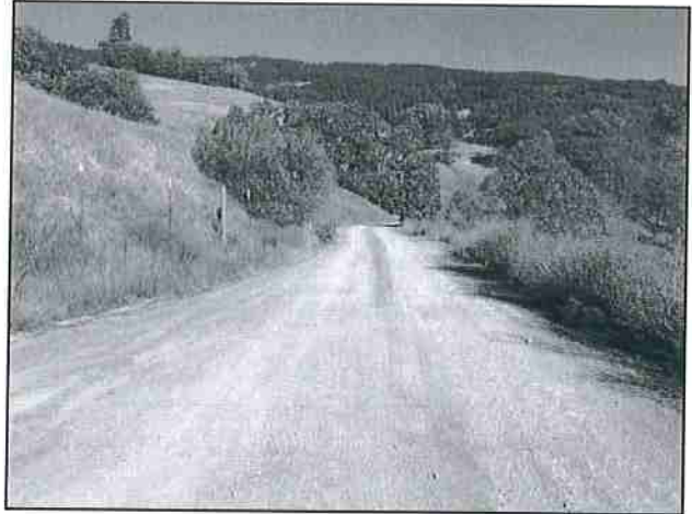
Photo #38 River Rd Looking East
