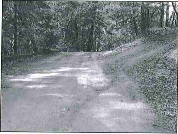
Photo #31 Intersection of River Rd & 208-241-019 Private Access Rd Looking NE
