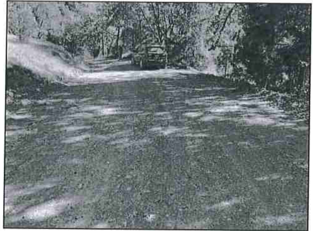
Photo #20 River Rd Looking SE @ Curve w/ Turnout
