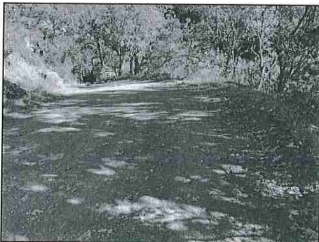
Photo #53 River Rd Looking SE @ Curve w/ Turnout
