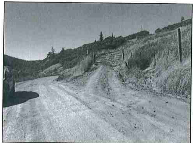
Photo #36 River Rd Looking NW @ Curve w/ Pullout & Approach
