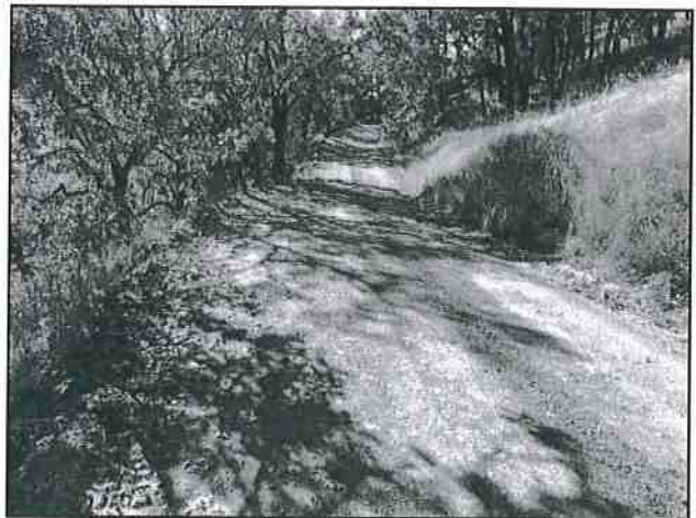
Photo #48 River Rd Looking West @ Turnout
