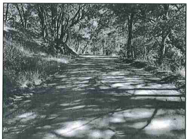
Photo #96 River Rd Looking SE @ curve w/ Turnout
