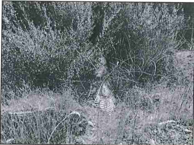
Photo #15 River Rd Looking @ 36" Culvert In
