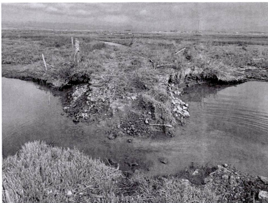
Photo 8—View of failed road crossing on Senestraro Lane (looking northeast) and the large interior slough (unnamed) that now passes over it.
