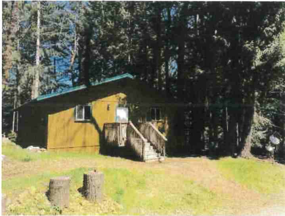
Photo 1. Site A, looking west at house from center of site
